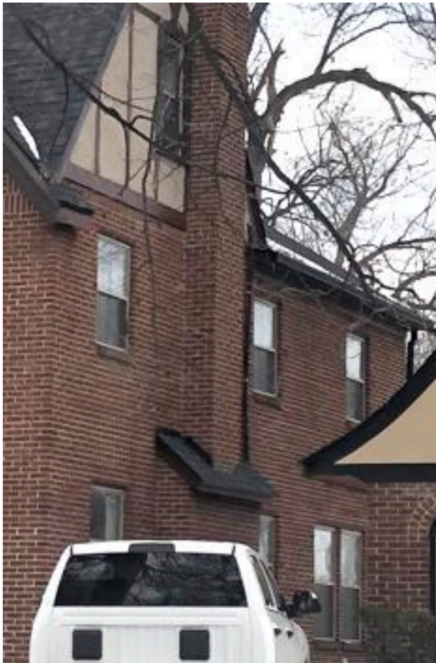
Current picture east elevation
