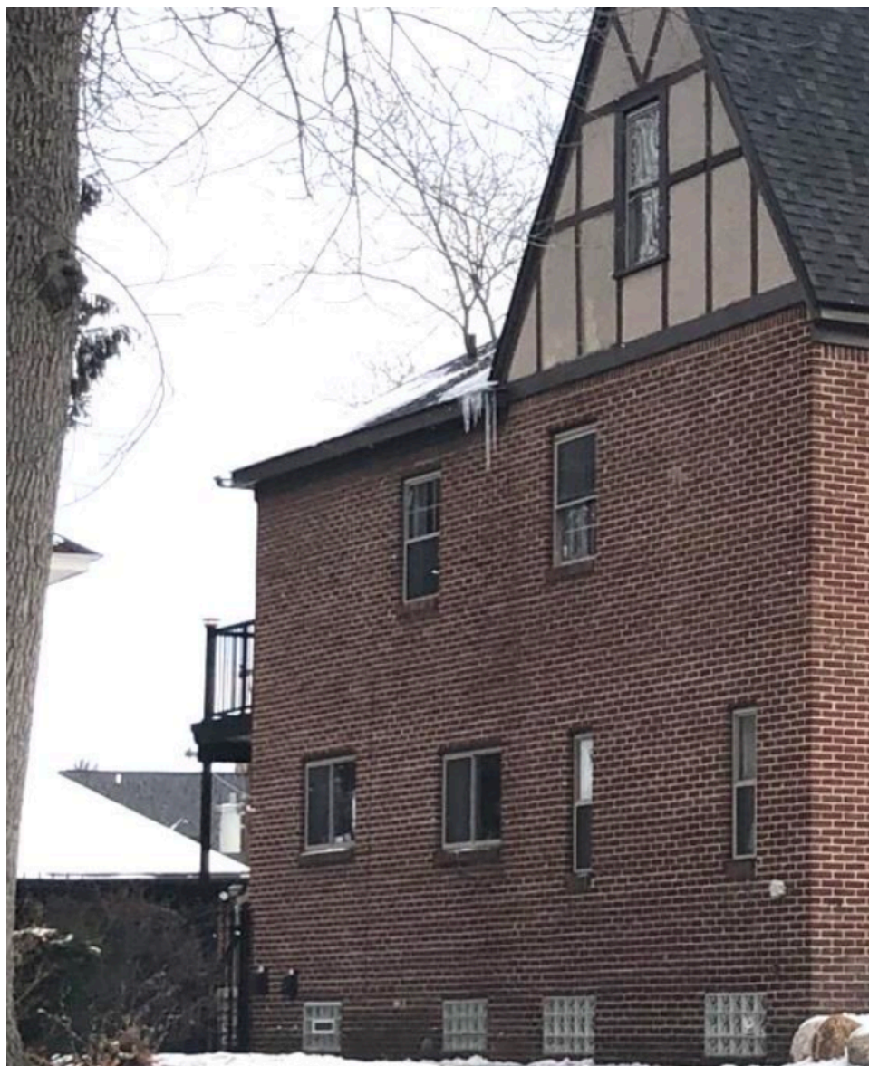
Current picture west elevation
