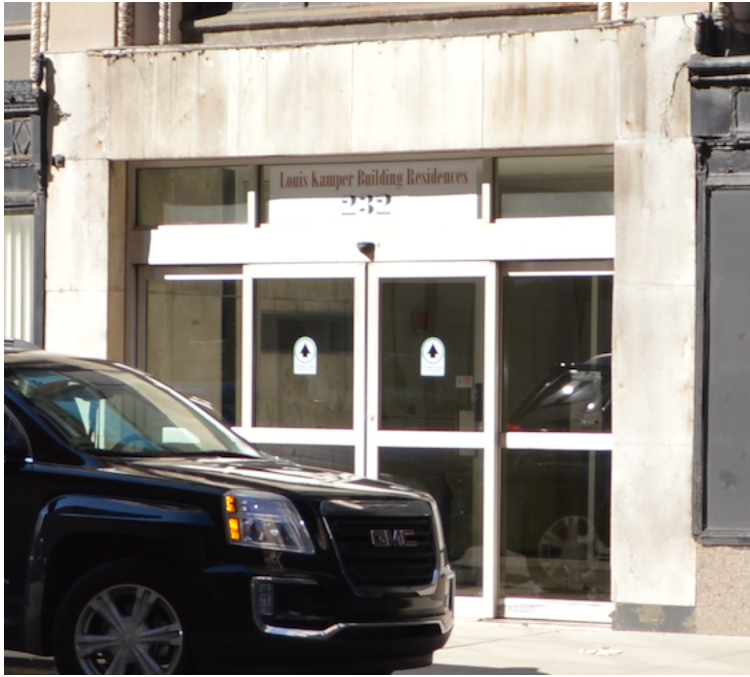
South building entrance, Sept 2016
