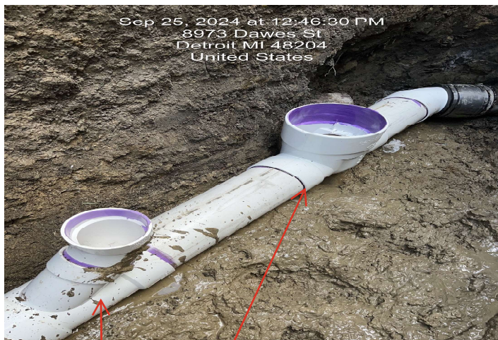
Clean Out & Backflow Valve Installation
