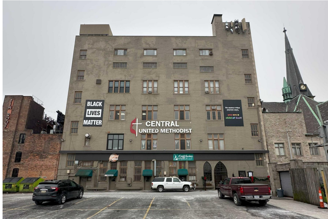
NORTH ELEVATION OF CHURCH HOUSE
