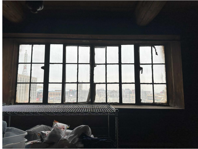
INTERIOR VIEW OF 5TH FLOOR WINDOW
