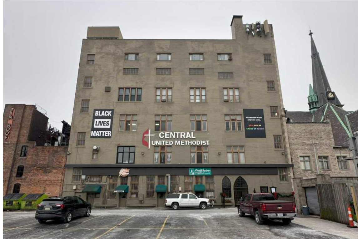
NORTH ELEVATION OF CHURCH HOUSE
