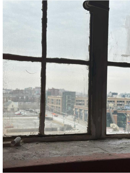
INTERIOR VIEW OF 5TH FLOOR WINDOW
