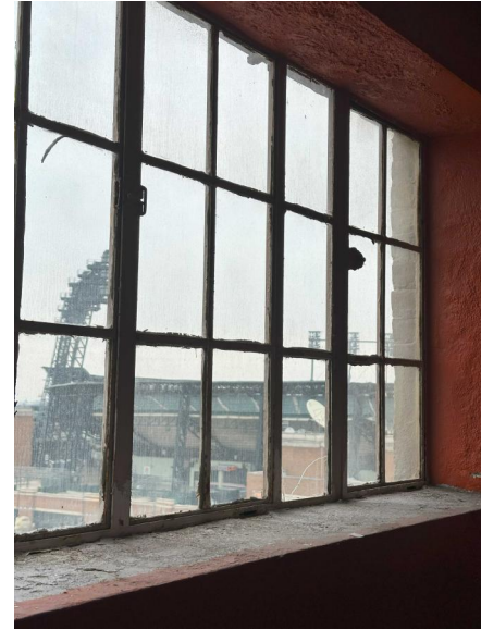
INTERIOR VIEW OF 5TH FLOOR WINDOW
