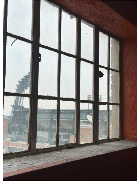
INTERIOR VIEW OF 5TH FLOOR WINDOW
