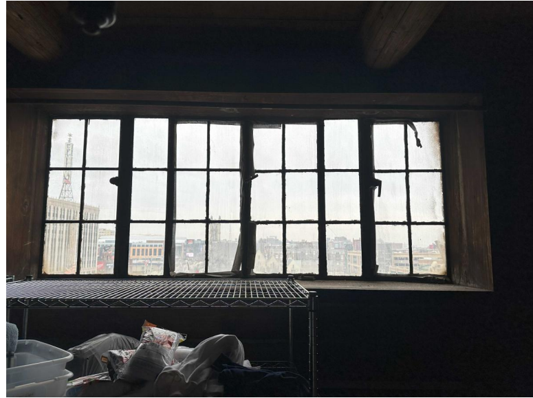
INTERIOR VIEW OF 5TH FLOOR WINDOW
