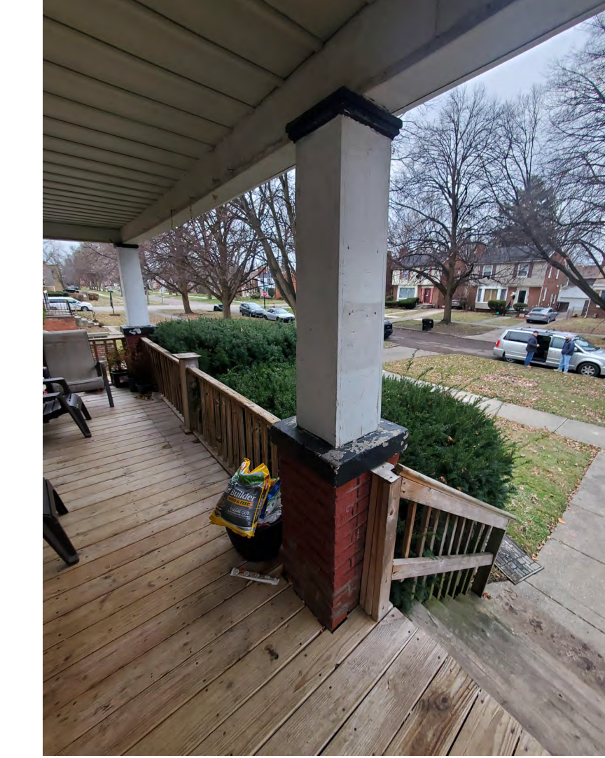
ON PORCH LOOKING SW
