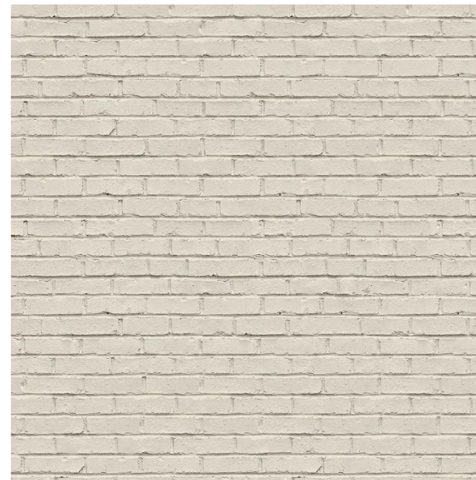
PAINTED BRICK VENEER (COLOR MATCH TO C:4 YELLOWISH WHITE)
