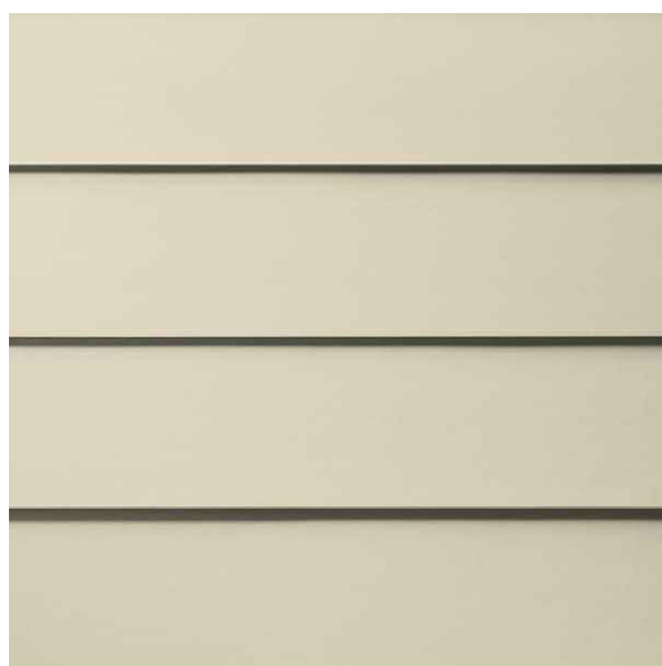
SIDING - PAINTED WOOD LAP SIDING - (COLOR MATCH TO C:4 YELLOWISH WHITE)
