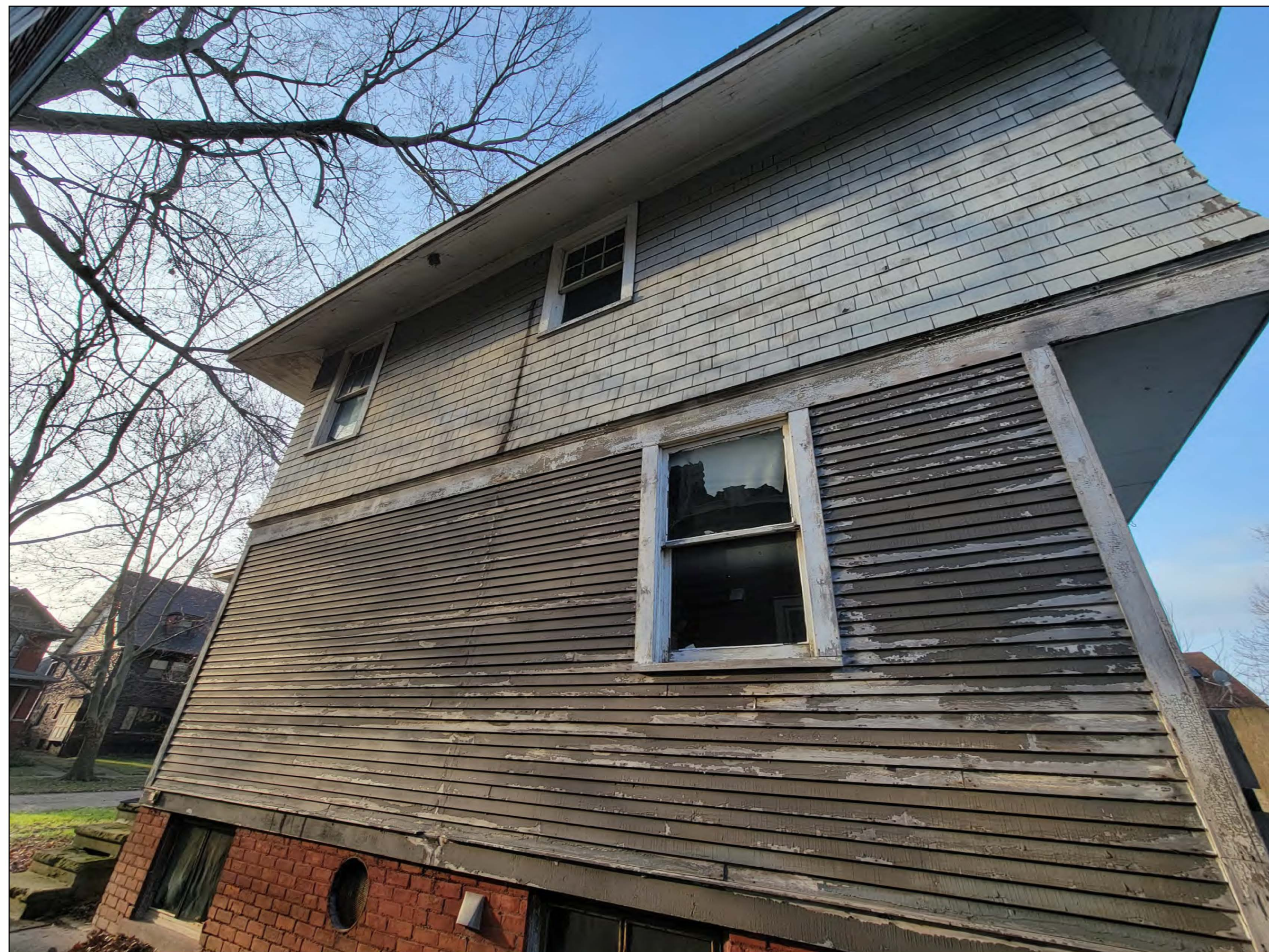
2 EAST ELEVATION - JANUARY 2024
