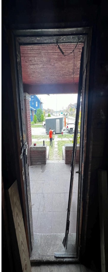
FIRST FLOOR ENTRY DOOR
