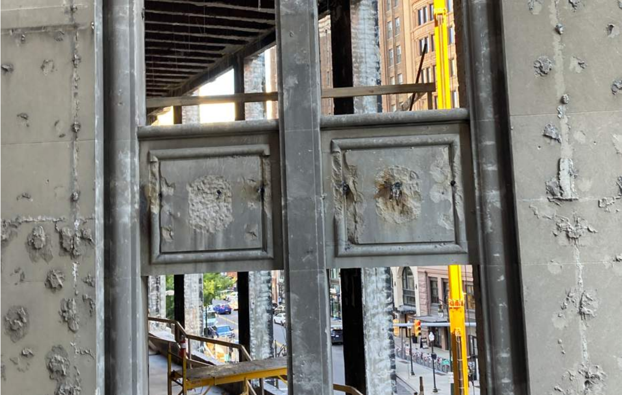
Alley facade after removal of steel angles from spandrels - 5th floor
