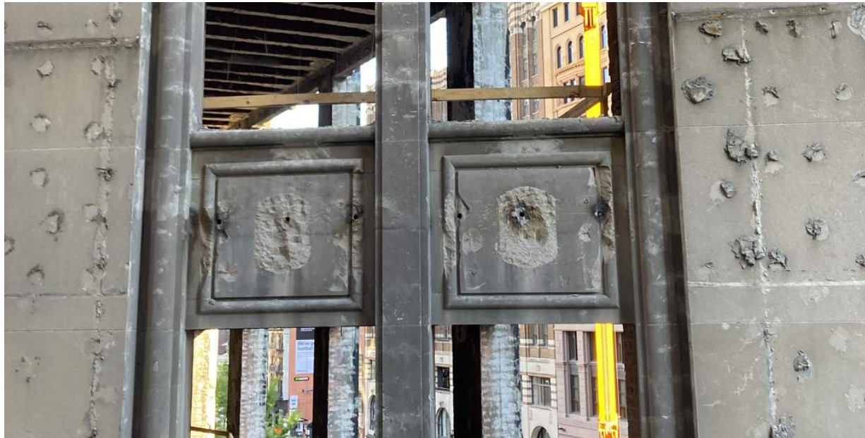
Alley facade after removal of steel angles from spandrels - 6th floor
