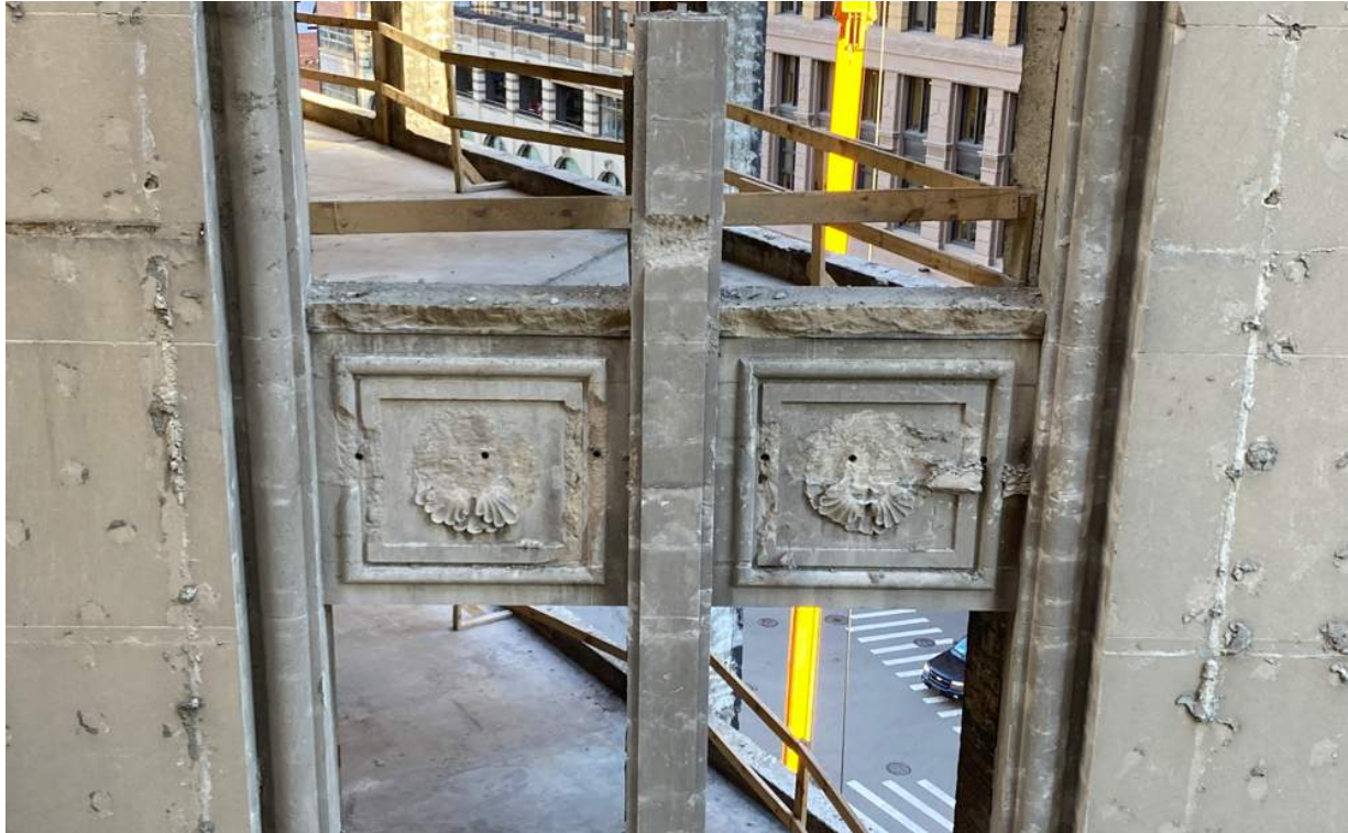
Alley facade after removal of steel angles from spandrels - 7th floor
