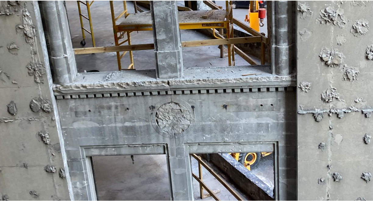
Alley facade after removal of steel angles from spandrels - 4th floor
