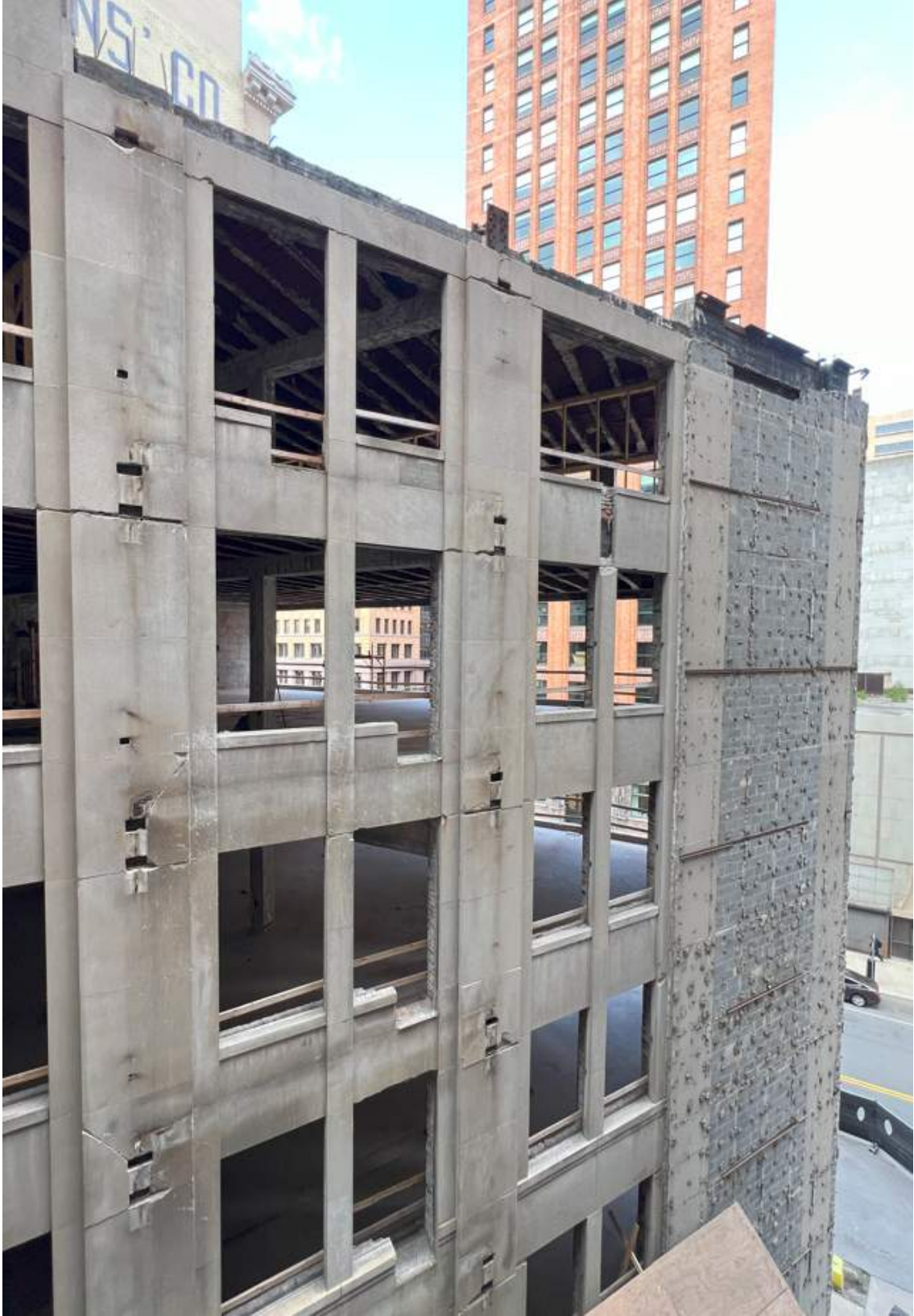
Alley facade prior to removal of CMU block
