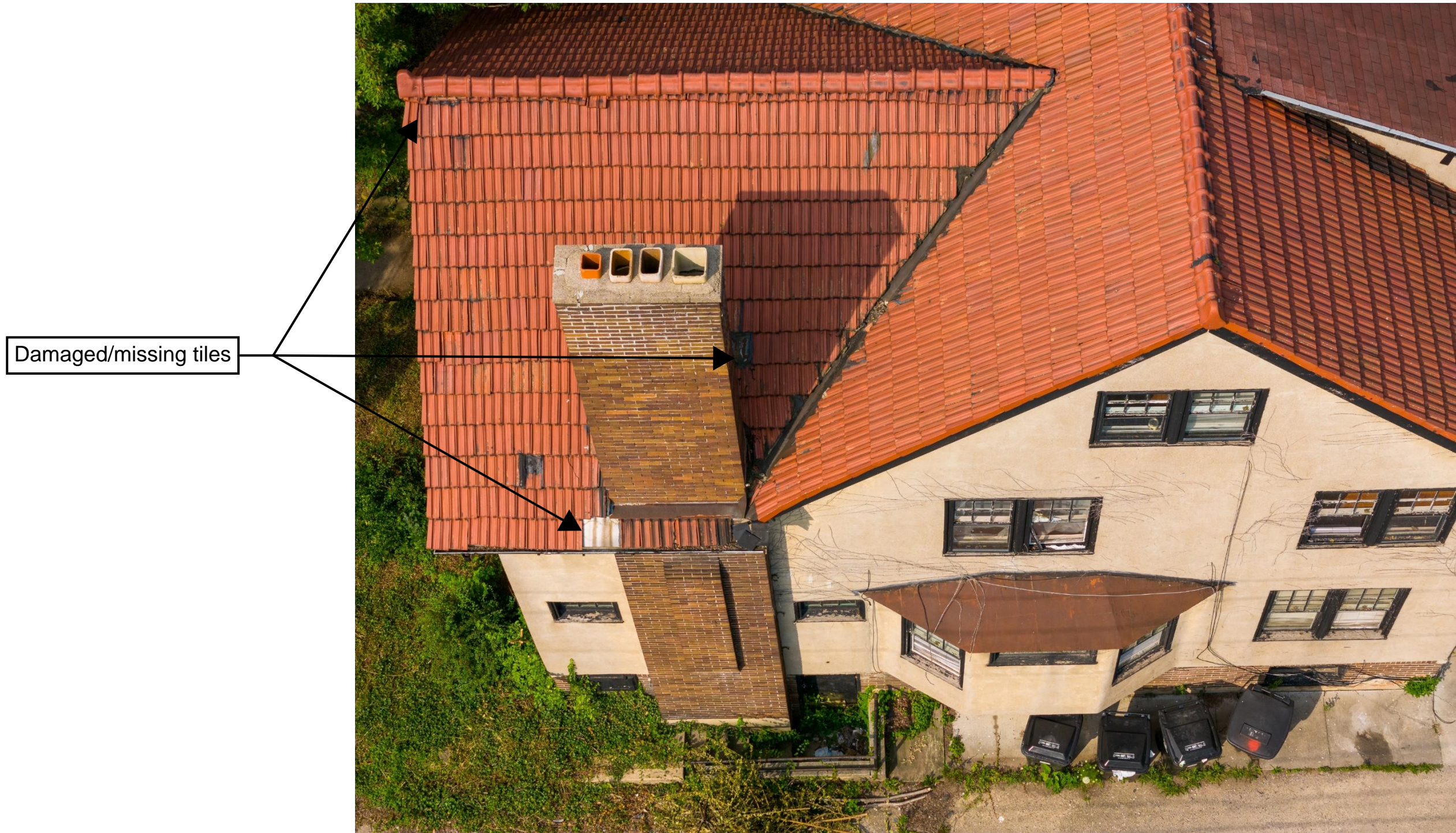
DRONE VIEW AT EAST END OF ROOF FACING ALLEY
