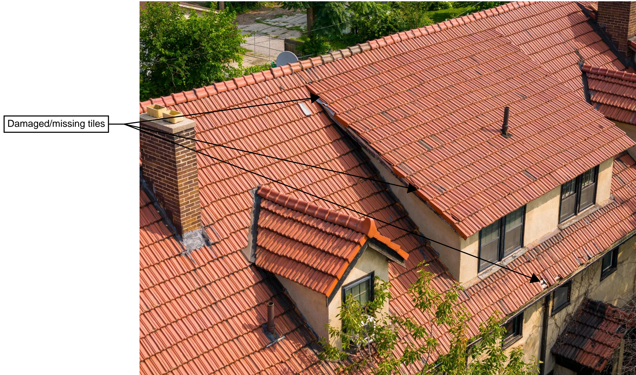
DRONE VIEW OF SOUTH SIDE OF ROOF FACING ST PAUL
