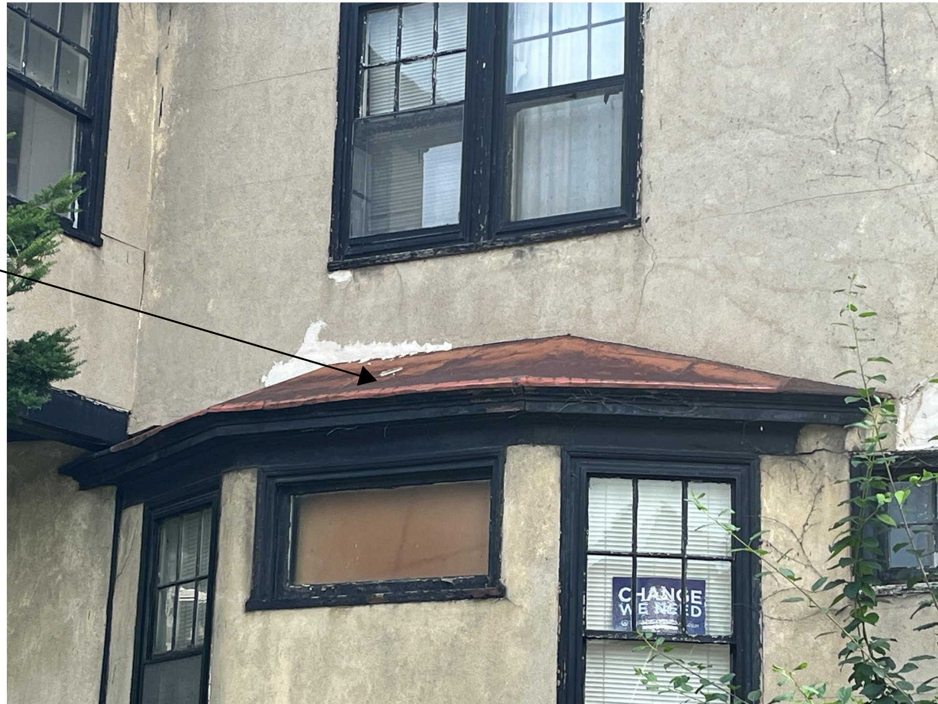
VIEW OF TYPICAL PROJECTING BAY WITHOUT TILE ROOFING
