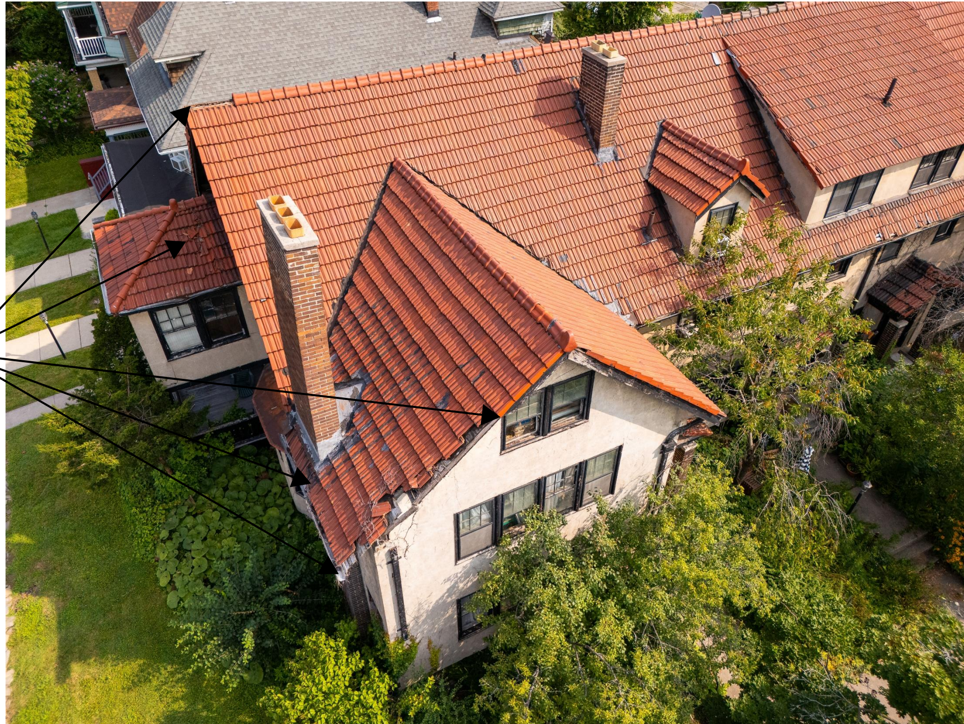
DRONE VIEW AT SW CORNER OF BUILDING
