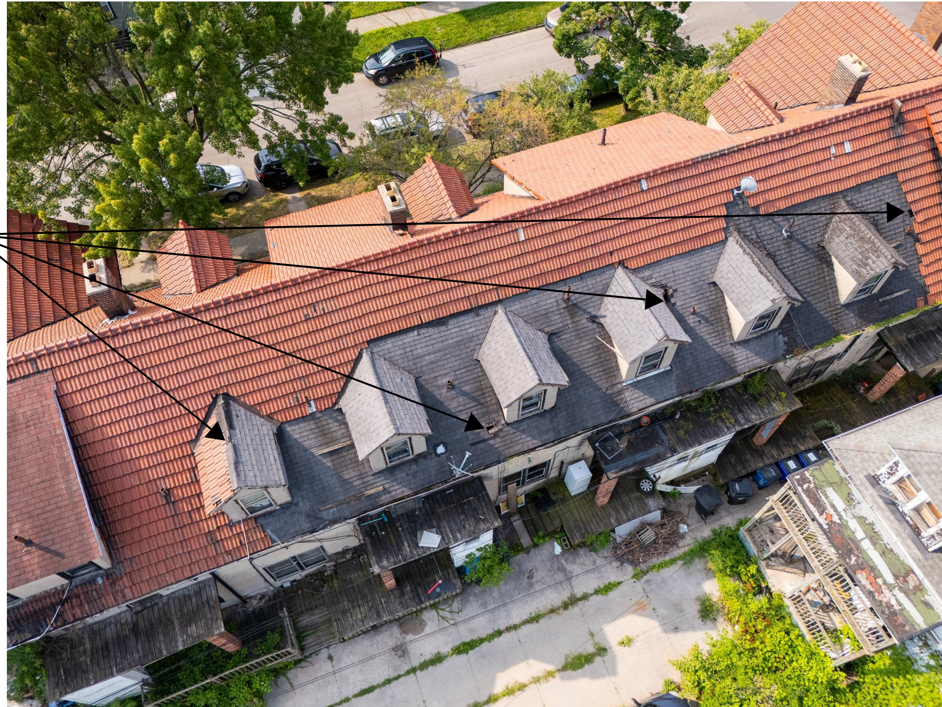
DRONE VIEW OF NORTH FACE OF ROOF SHOWING REPLACEMENT ASPHALT SHINGLES
