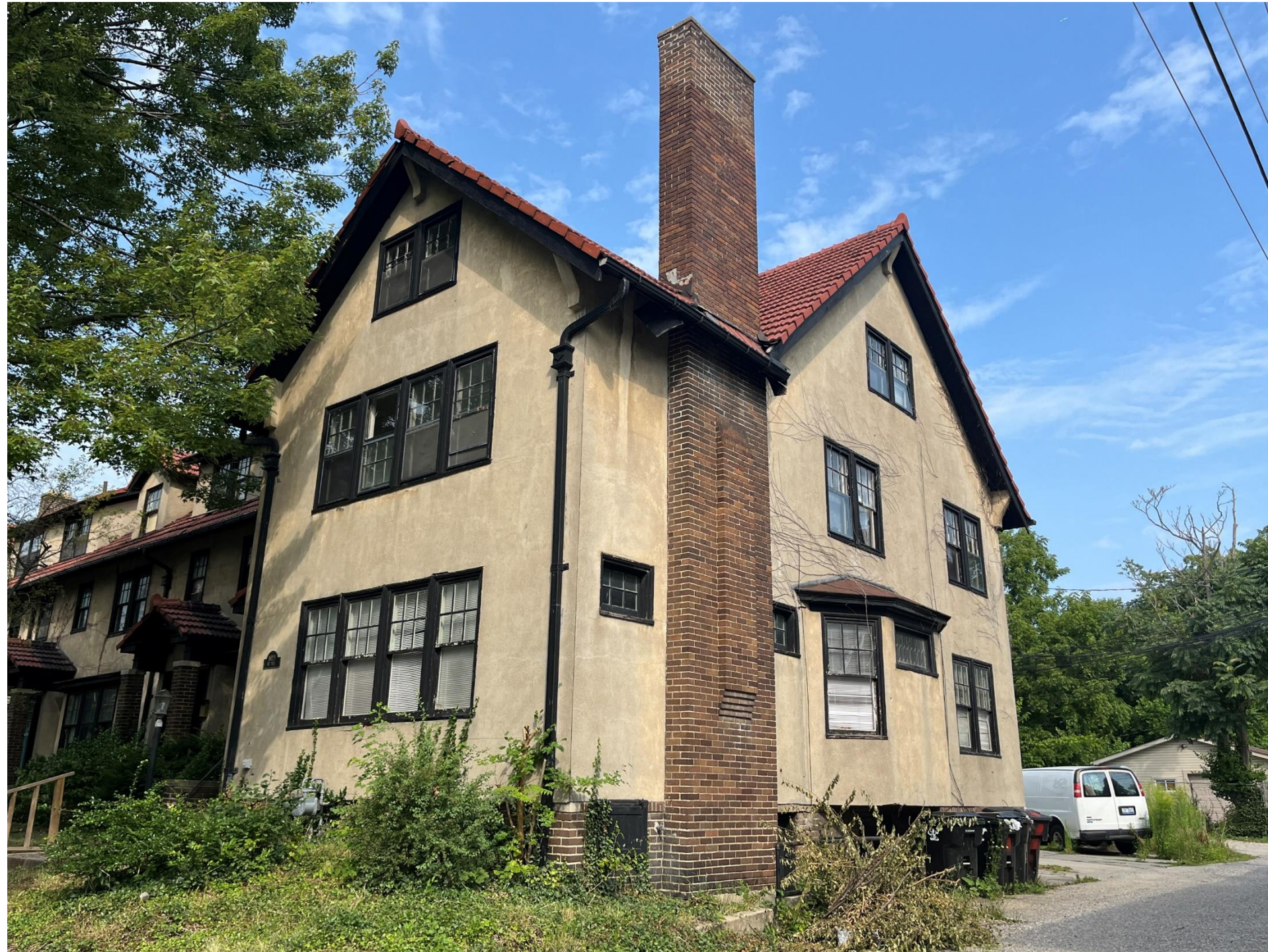
VIEW FROM GRADE AT SW CORNER OF BUILDING FACING ALLEY
