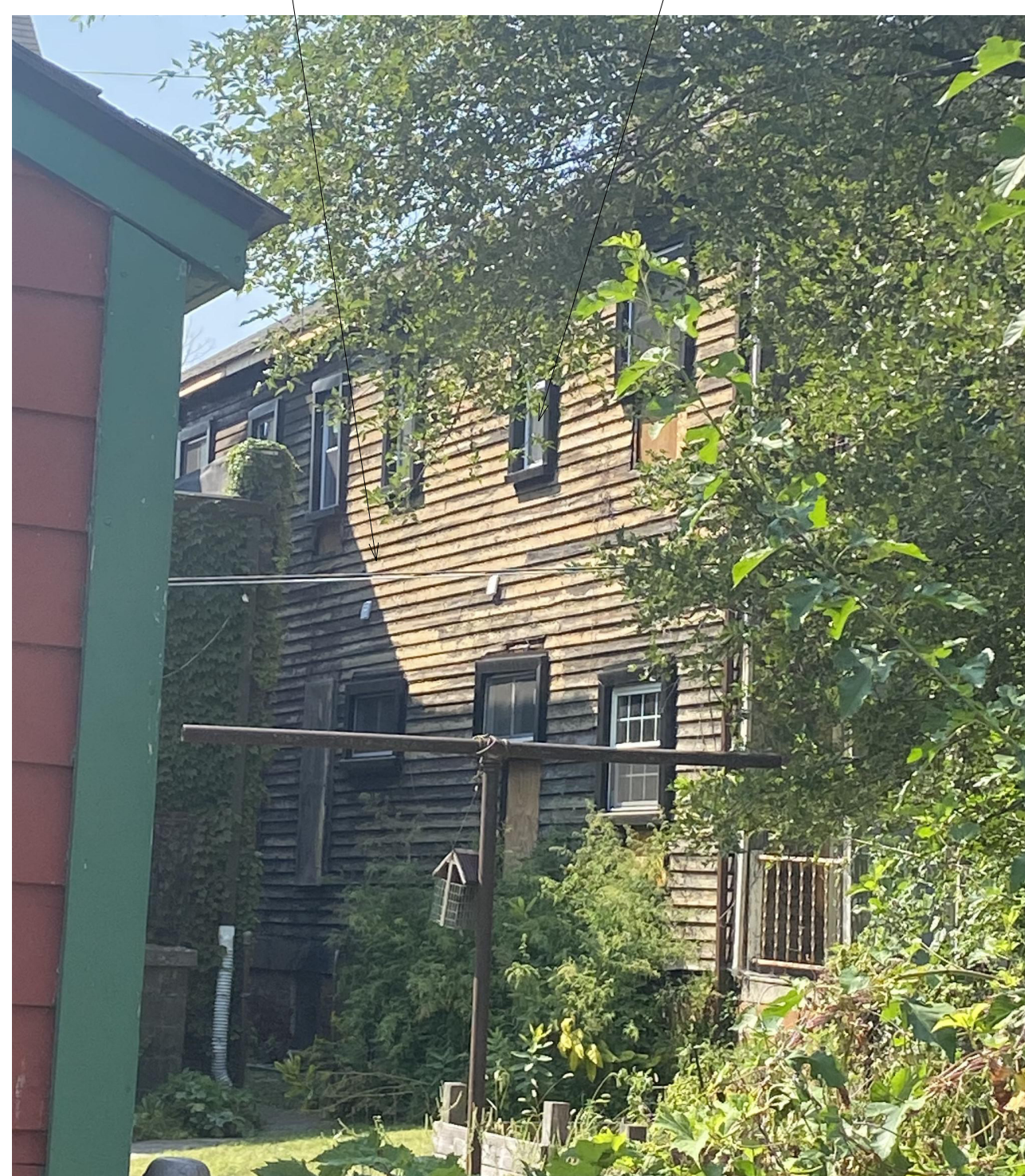
PHOTO OF SIDE (SOUTH) FACADE (09/12/2024)
