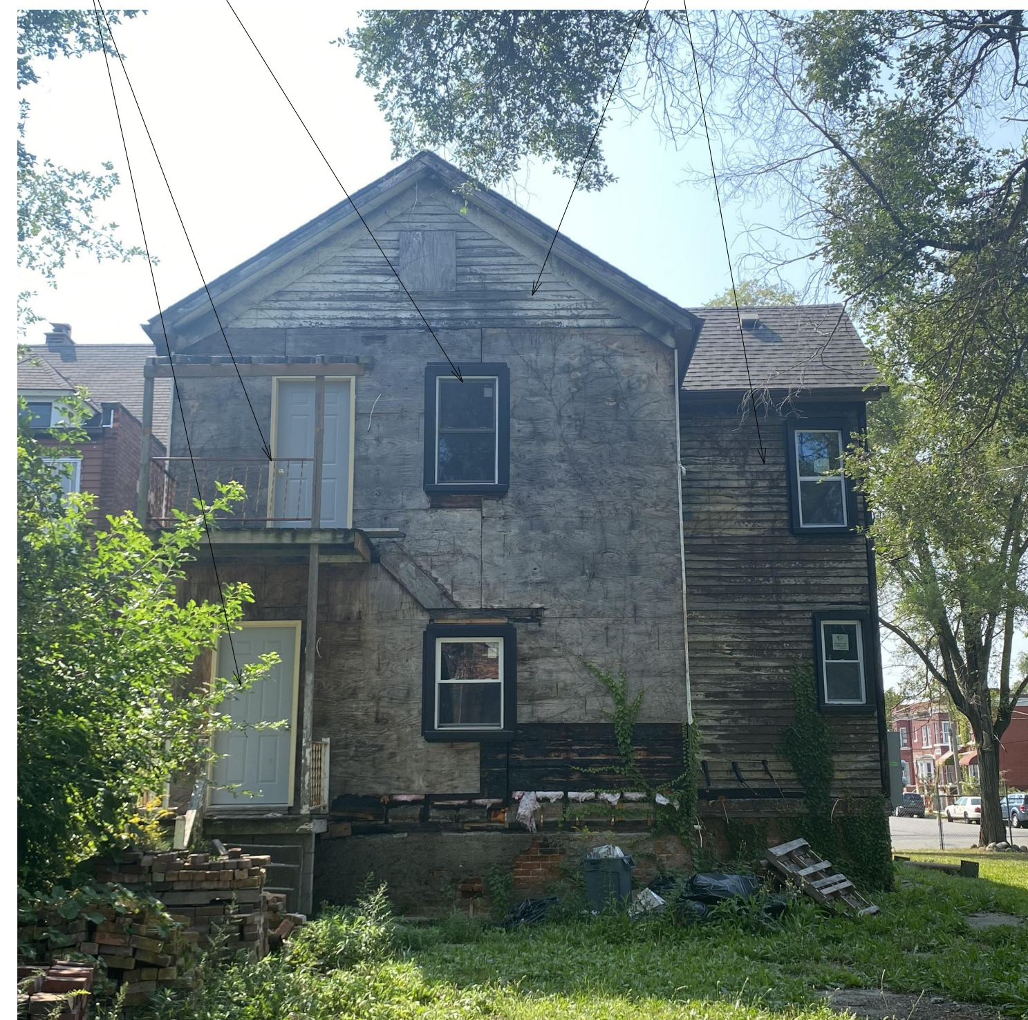
PHOTO OF REAR (EAST) FACADE (09/12/2024)
