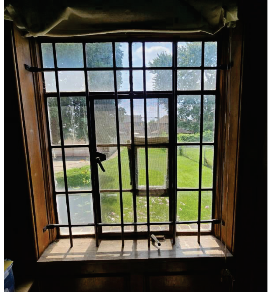
4031 Fullerton St Unit 108 – Replace with single casement window (Grille will be 4w x 4h to match)
