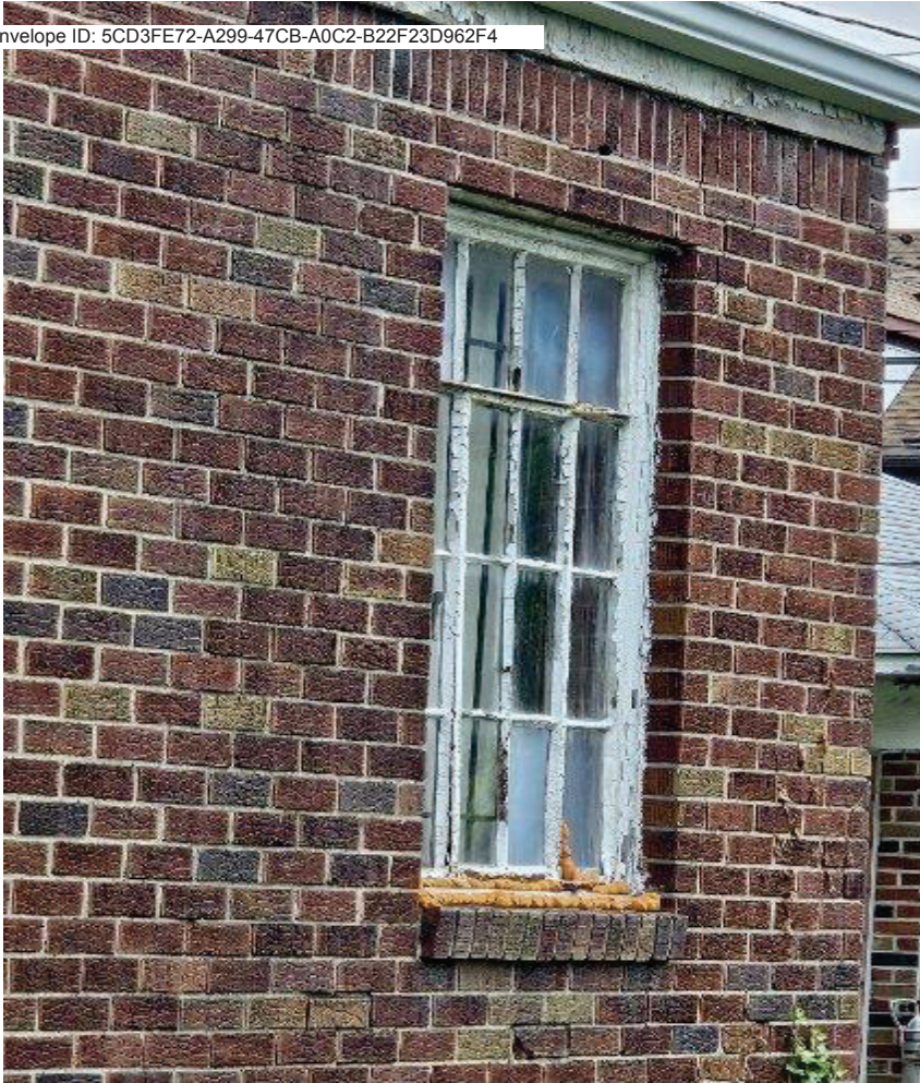
4031 Fullerton St Unit 107 – Replace with single casement window (Grille will be 4w x 4h to match)
