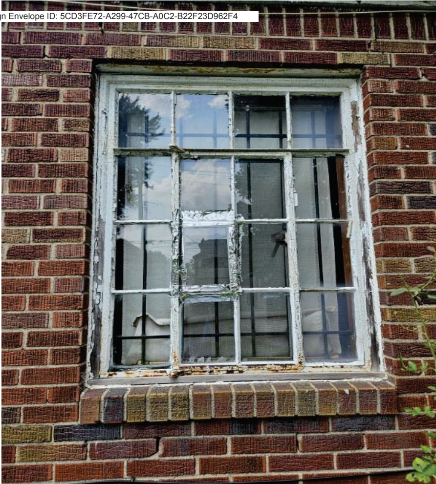
4031 Fullerton St Unit 108 – Replace with single casement window (Grille will be 4w x 4h to match)
