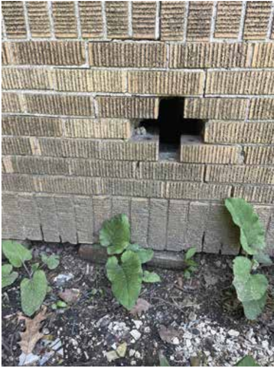
Replace missing bricks from the side.
