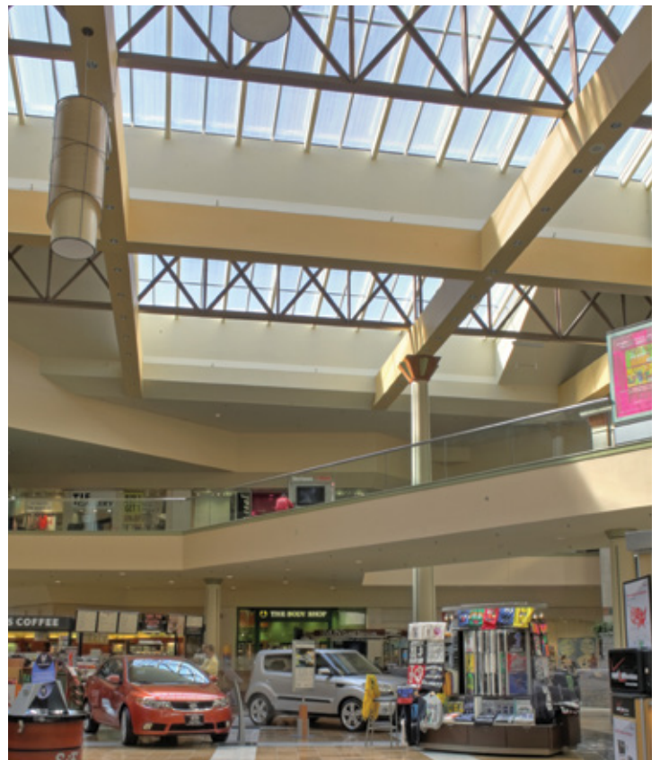
Single Pitch, Rockaway Town Center, Rockaway, NJ
