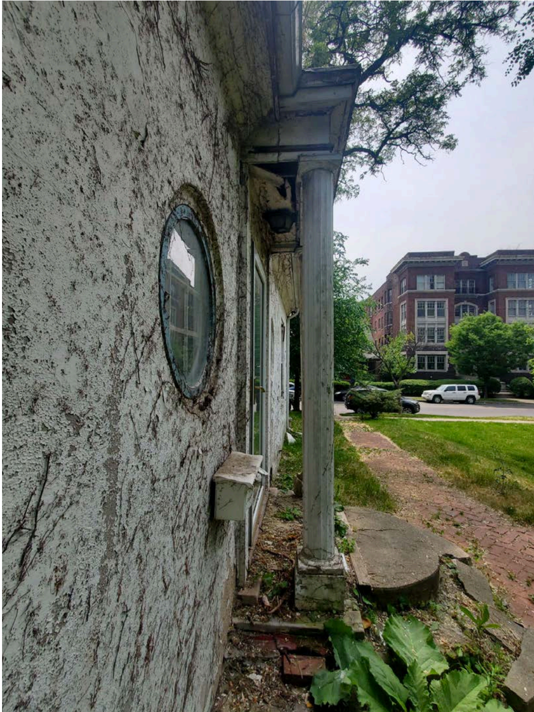
Existing Porch West Elevation
