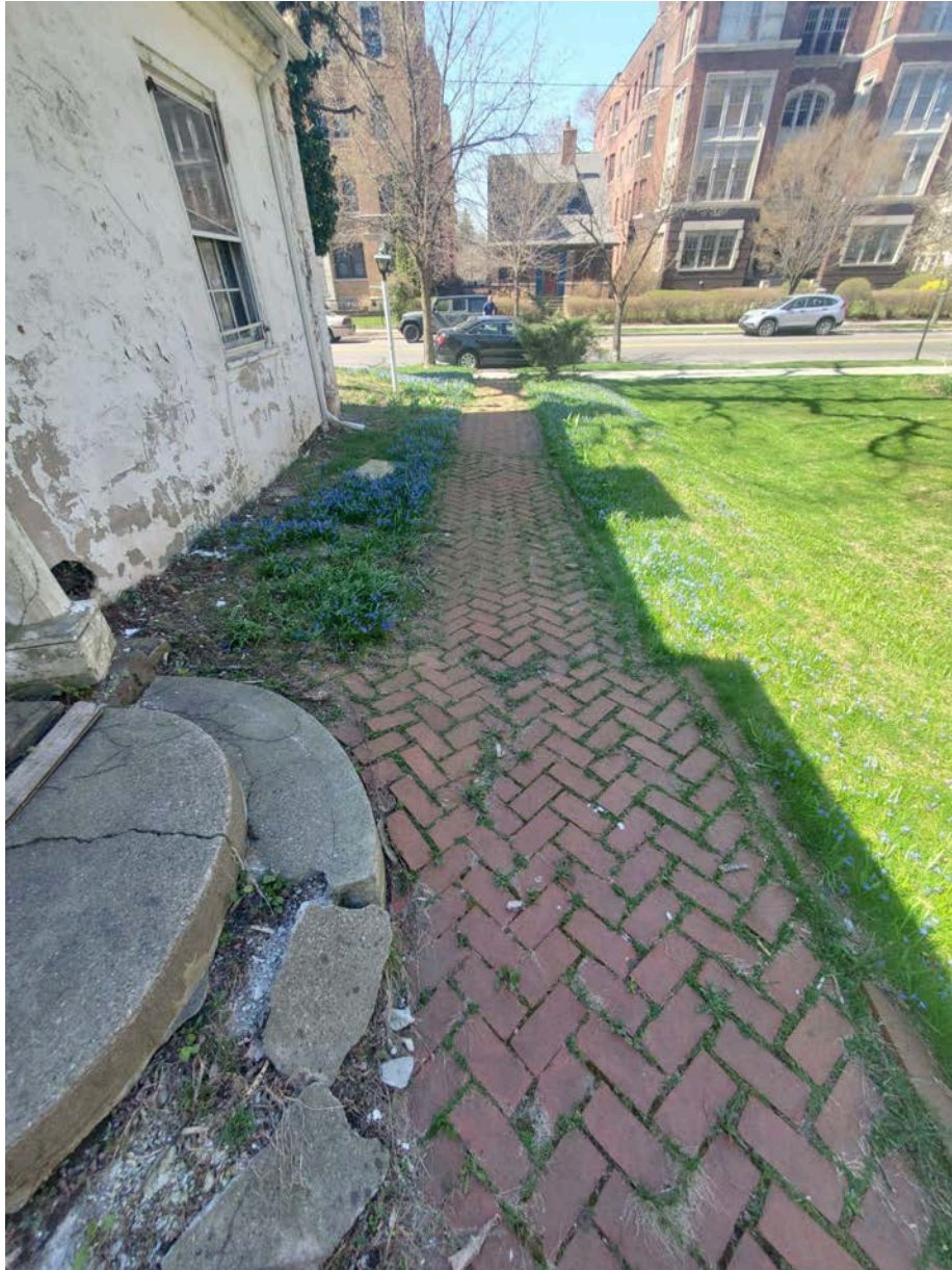
Existing Brick Path
