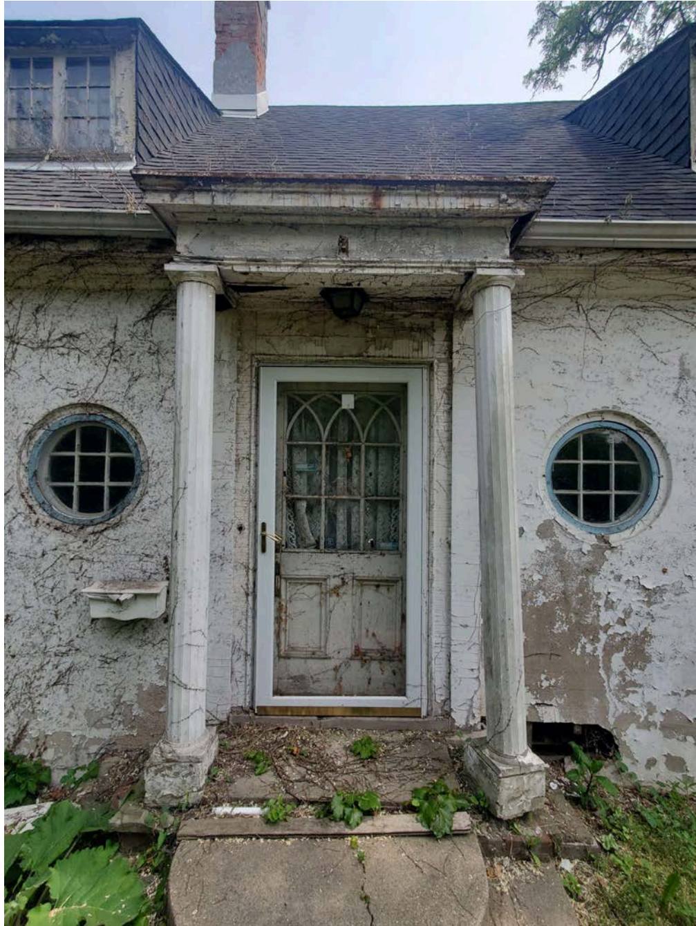
Existing Porch Detail
