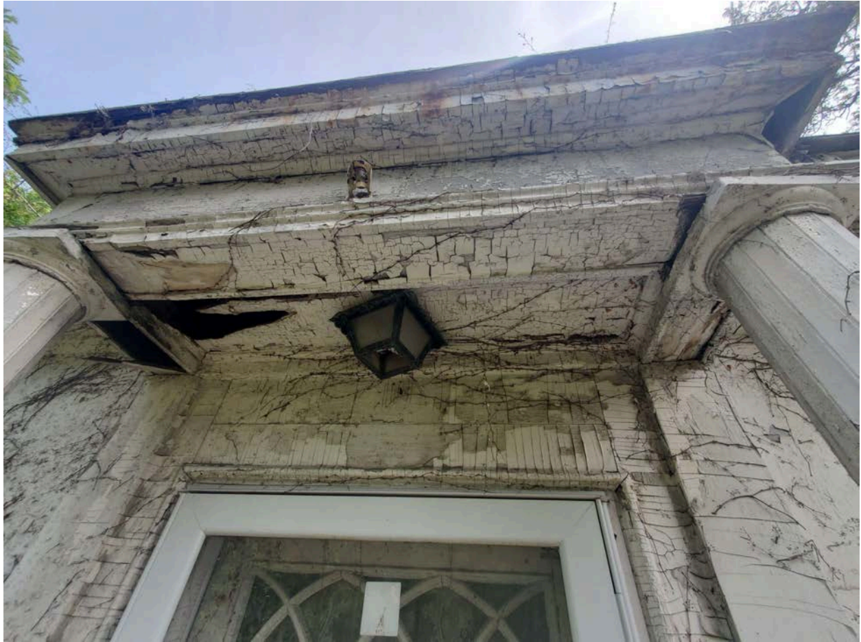
Existing Porch Canopy Soffit
