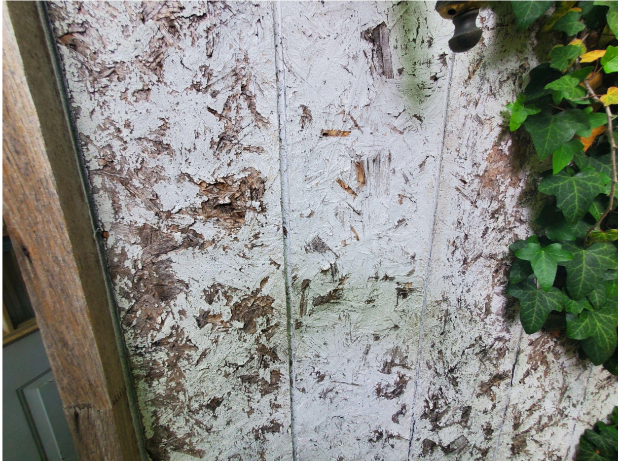
Garage South Elevation Detail
