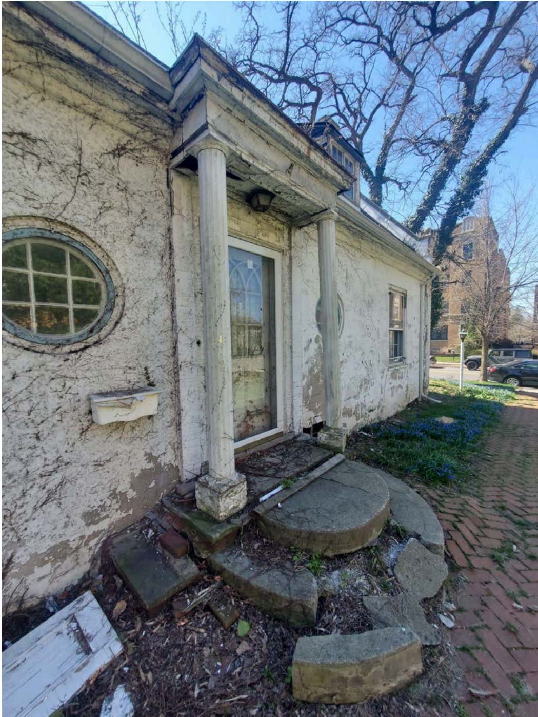
Existing Porch Detail
