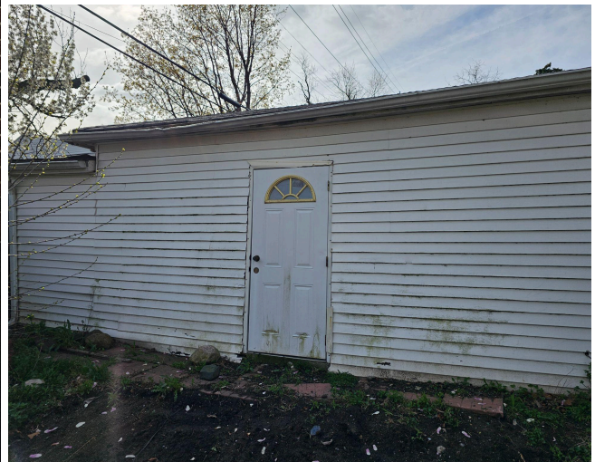
Fig. 12.0 - Existing Garage facing North
