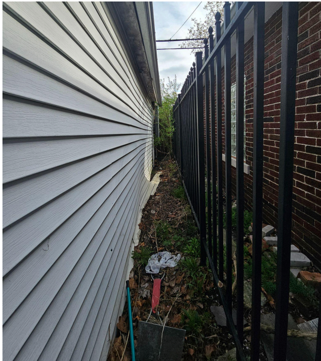
Fig. 11.0 - Existing Garage facing South
