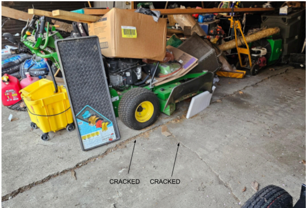
Fig. 10.0 - Existing Garage Slab
