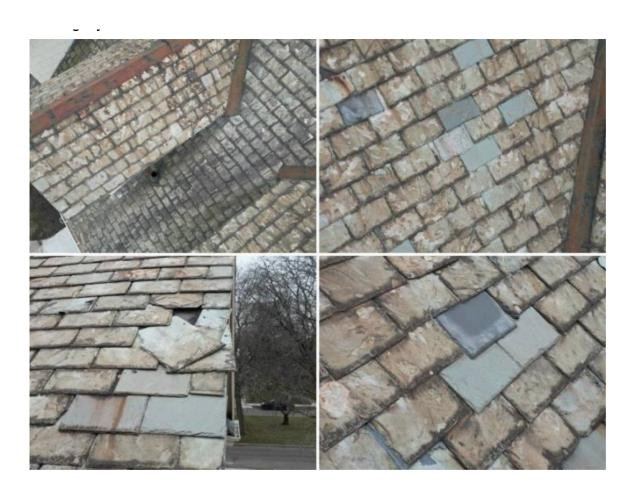
A drone was used to examine the roof surface. No walking on the roof was required. From the ground with a telescoping camera. and viewed from attic where damage can often be readily seen.
