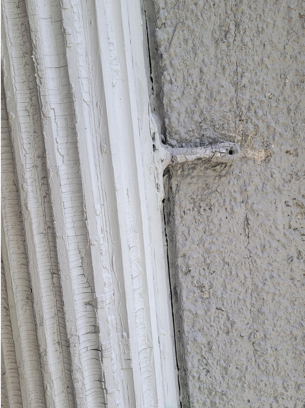
Existing Column B
