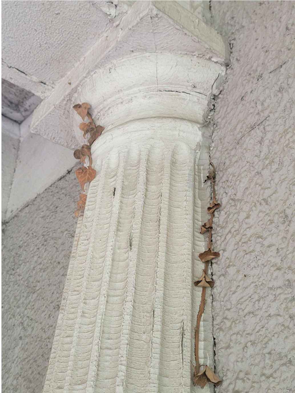
Existing Column A
