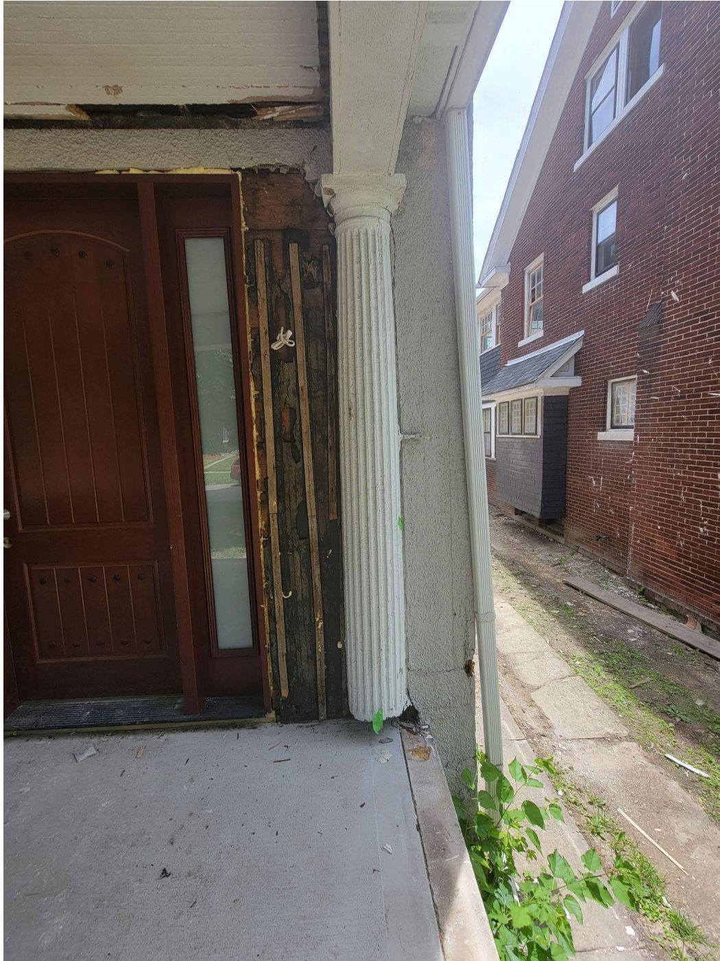
Existing Column B
