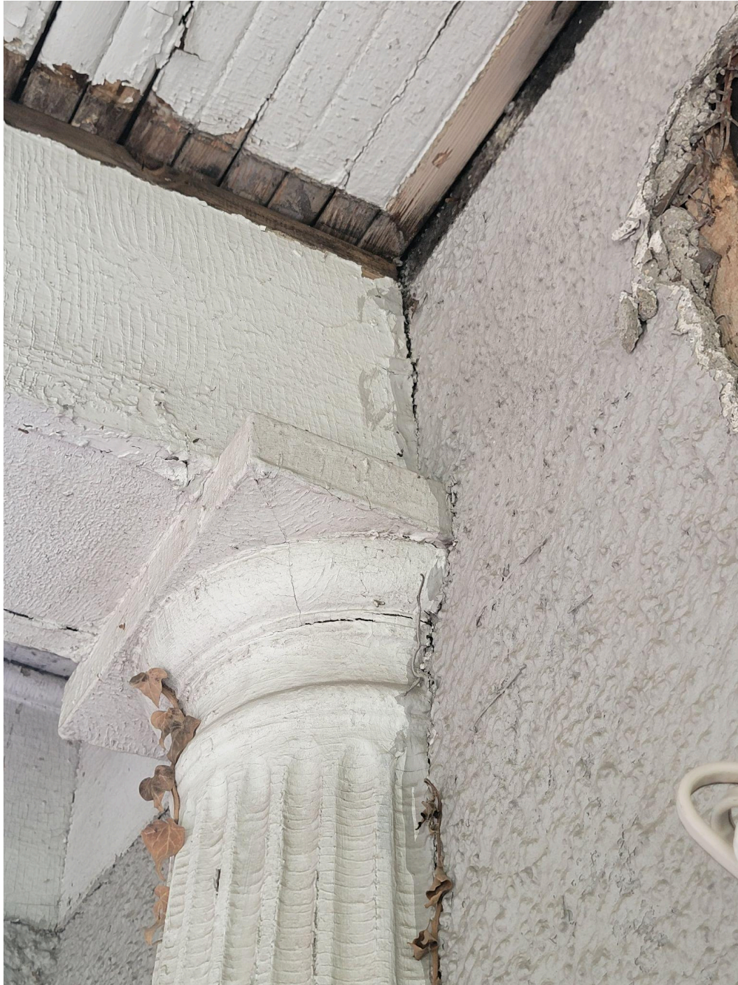
Existing Column A
