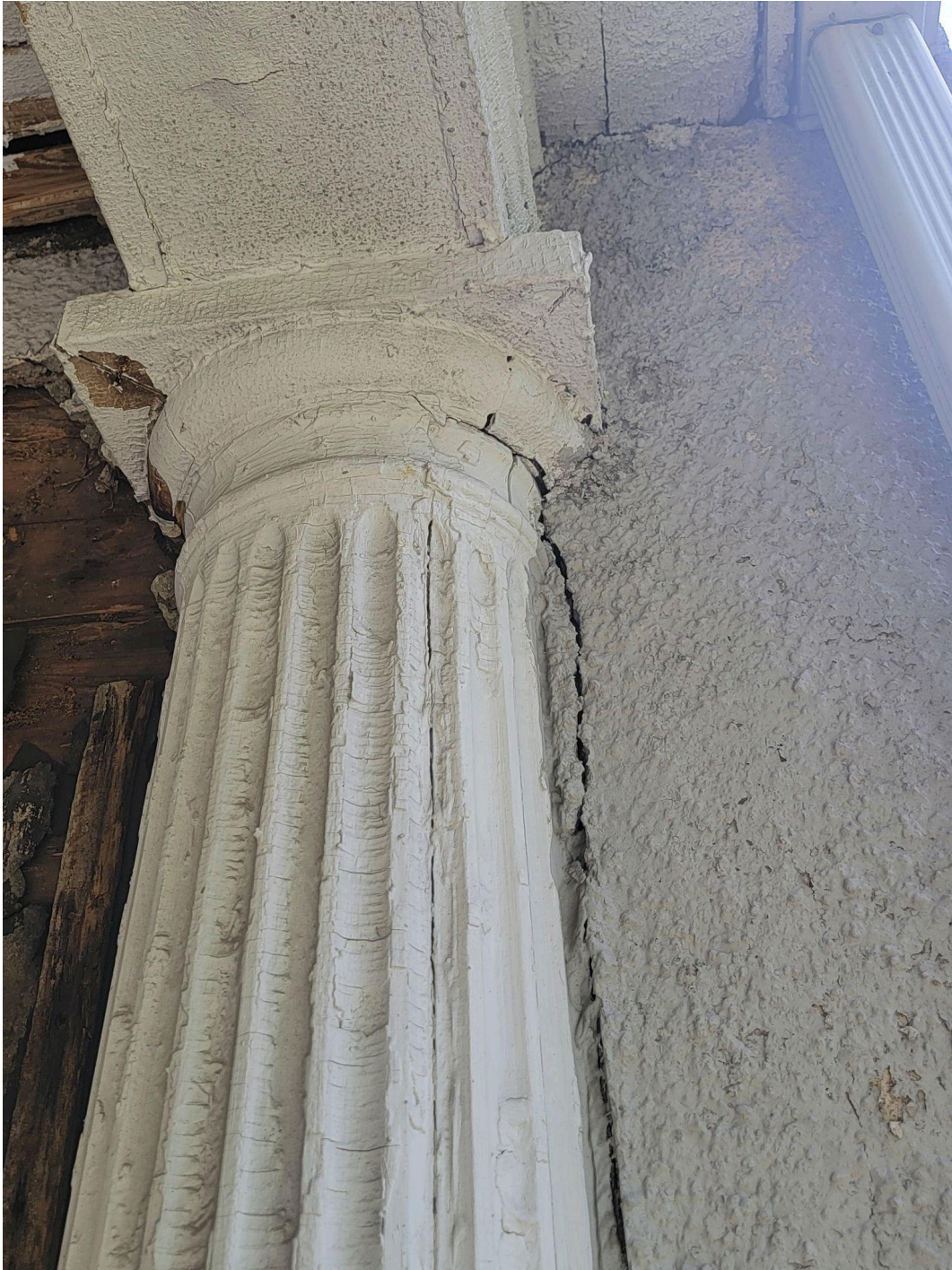
Existing Column B
