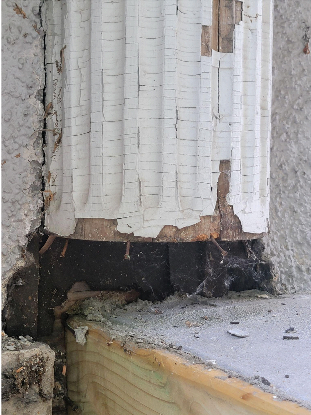
Existing Column A
