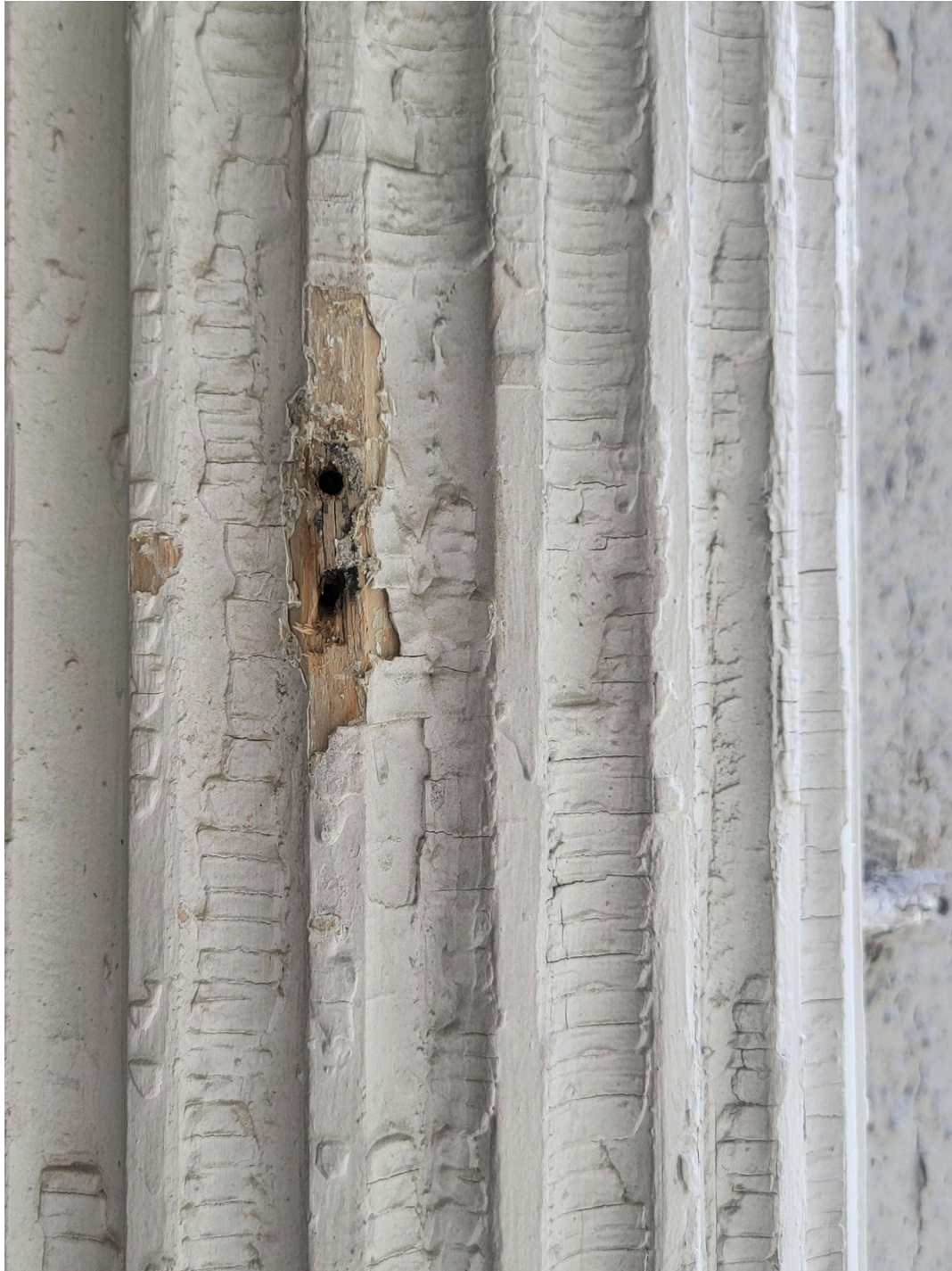
Existing Column B
