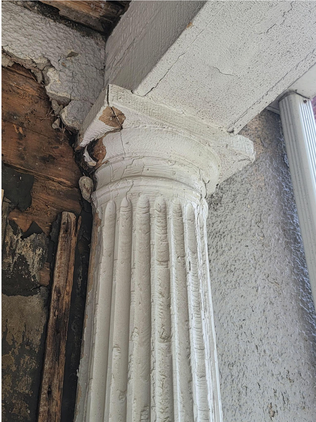
Existing Column B
