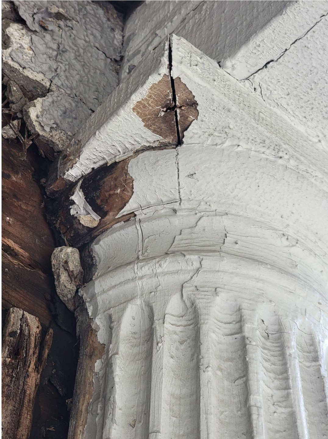
Existing Column B
