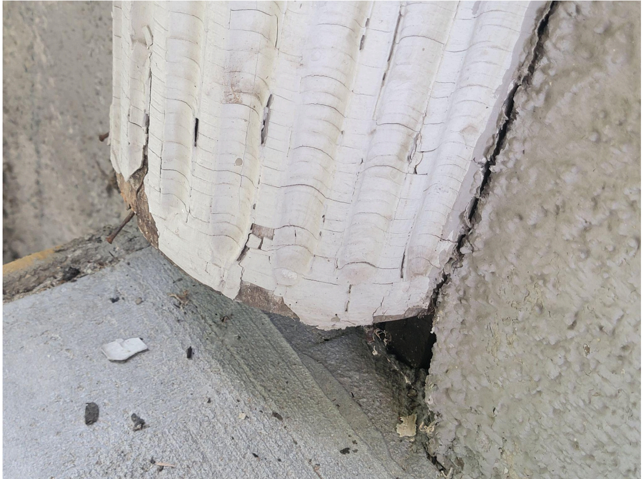
Existing Column A
