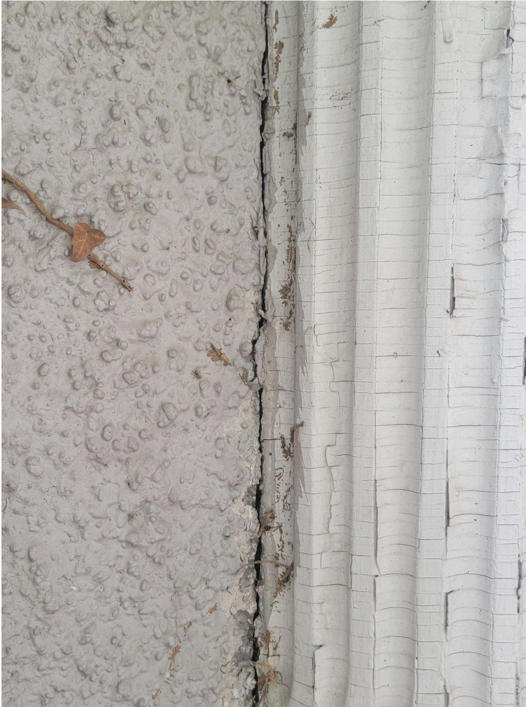
Existing Column A
