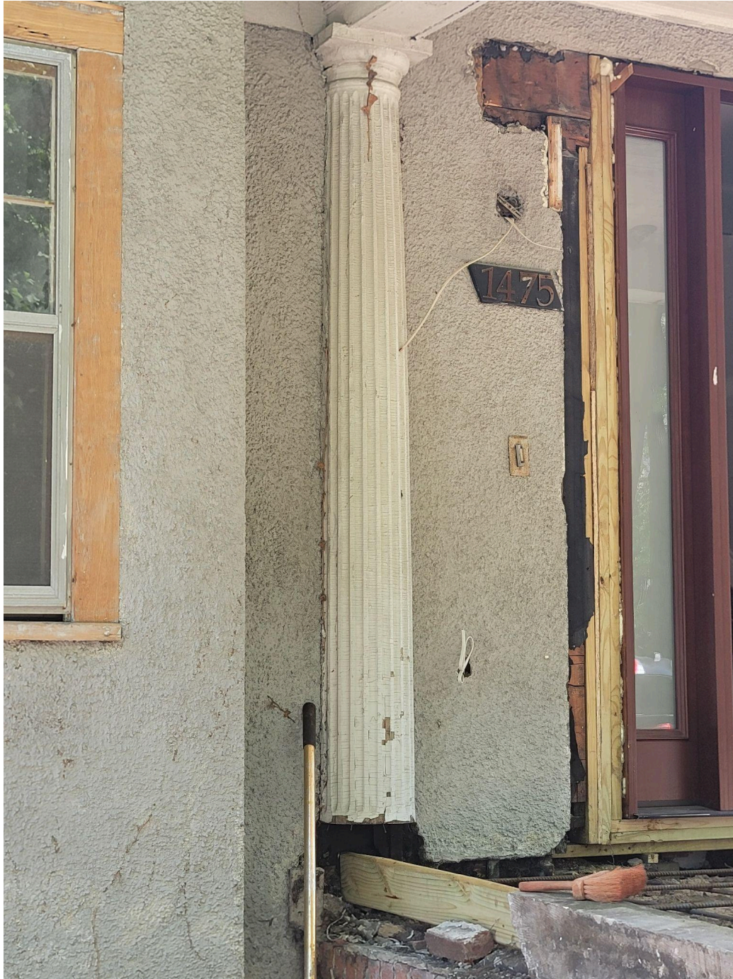
Existing Column A
