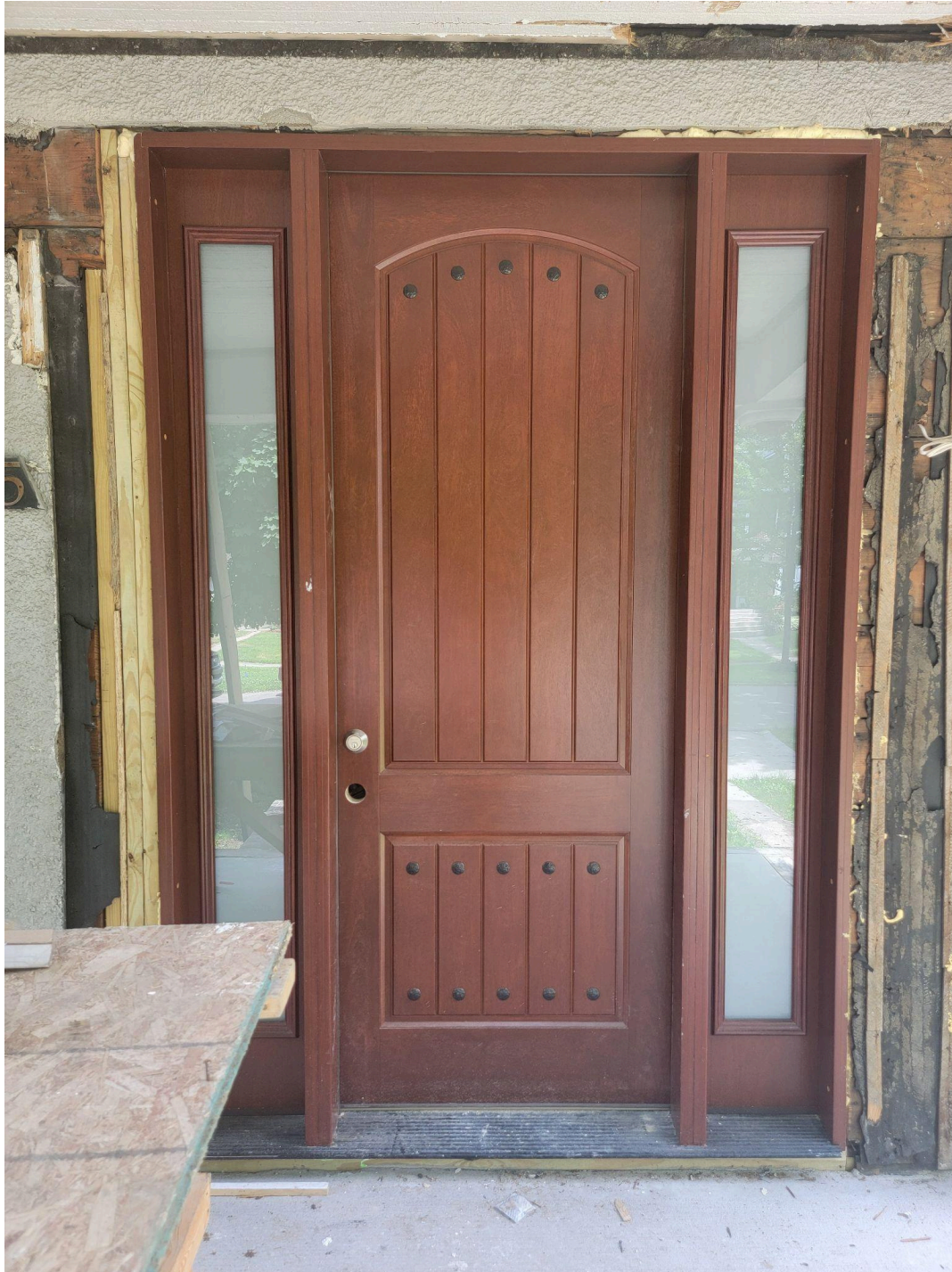
Current Front Door (to be replaced)
