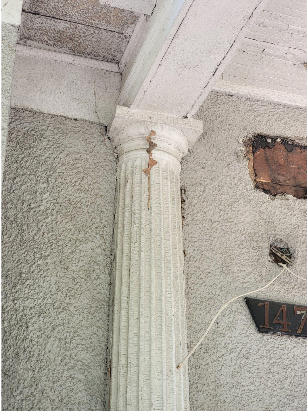
Existing Column A
