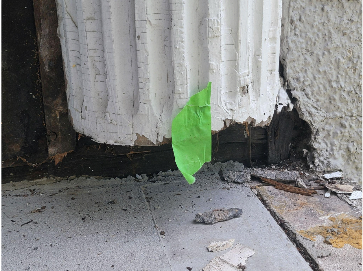
Existing Column B
