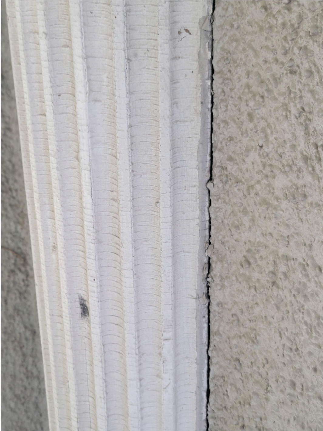
Existing Column A
