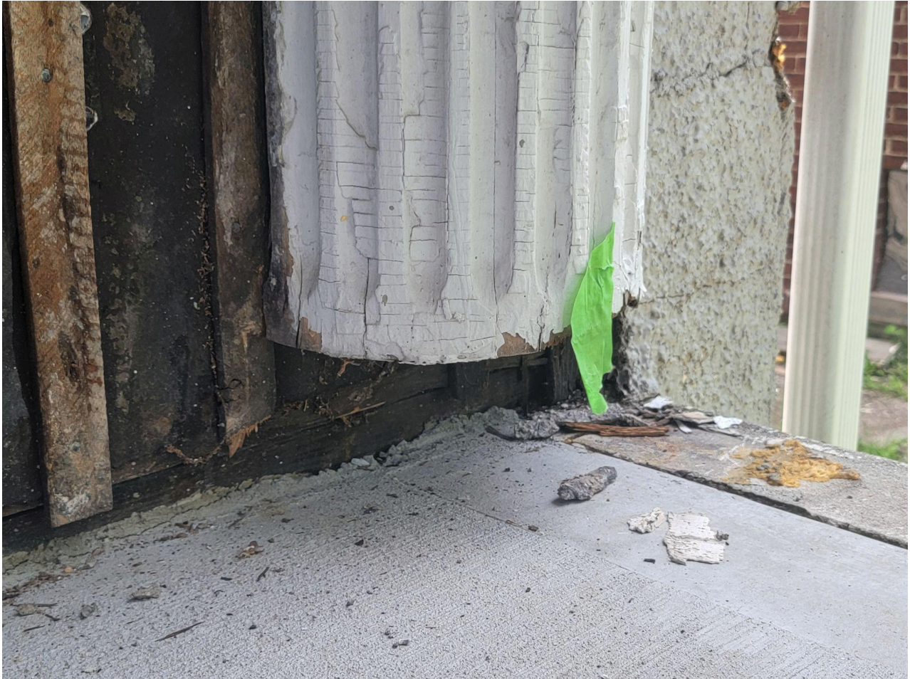
Existing Column B
