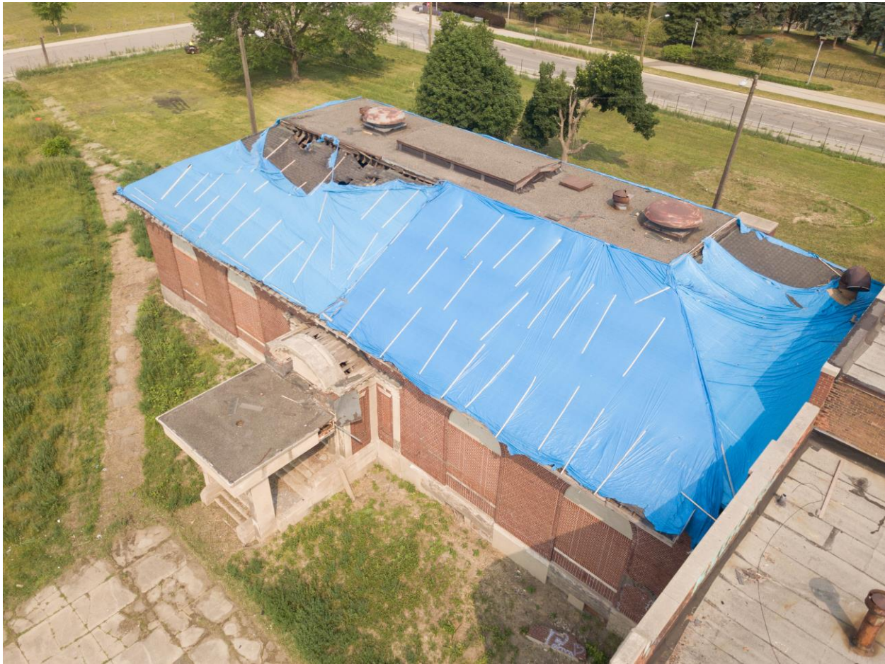
Existing Condition Photo 3: The canopy was added & decreased the height of the original entry.
