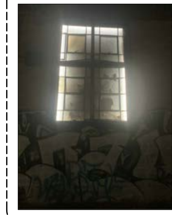
EXISTING HOT ROLLED STEEL WINDOW
