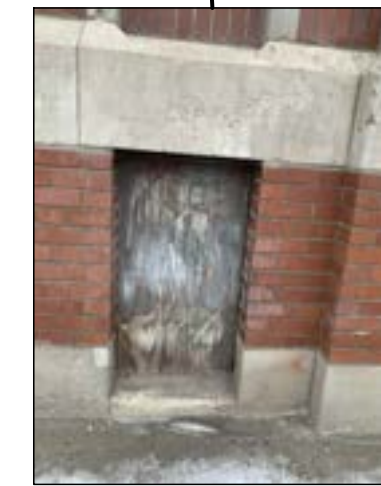
EXISTING BASEMENT WINDOW CONDITION - TYPICAL
