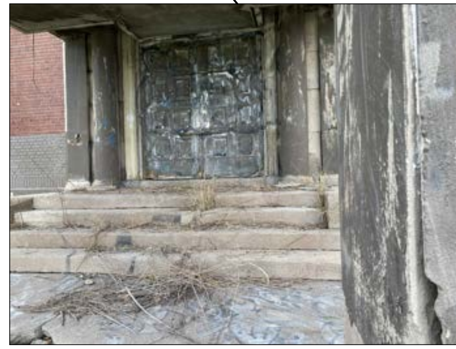
REPLACEMENT DOOR (ADDED W/ CANOPY DUE TO DECREASING CEILING HEIGHT) TO BE REMOVED AND RESTORED TO ORIGINAL DOOR & FRAME PER HISTORIC PHOTOS
