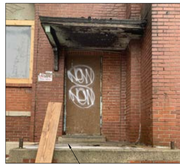
EXISTING RAIL IS CUT AND REMOVED EXISTING PHOTO
