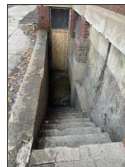
EXISTING WOOD DOOR FRAME W/ FLYWOOD INFILL
