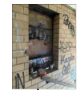
EXISTING HOT ROLLED STEEL WINDOW
