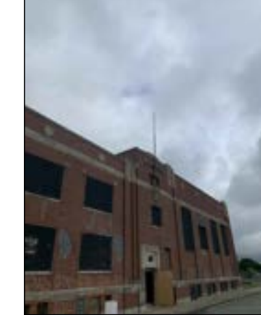
EXISTING TEMPORARY DOOR INFILL CONDITION - TYPICAL
