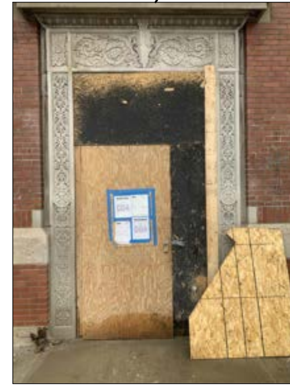
EXISTING TEMPORARY DOOR INFILL CONDITION - TYPICAL
