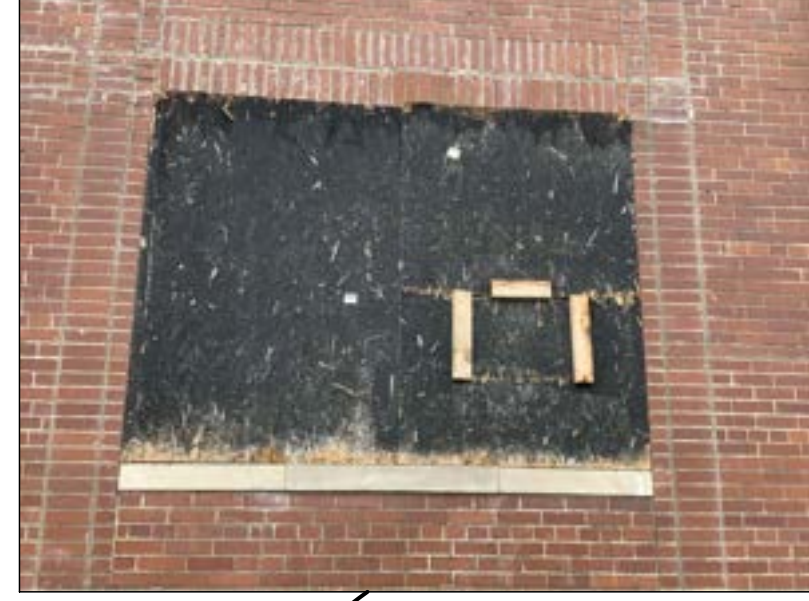
EXISTING INFILL - TYPICAL AT WOOD WINDOWS
