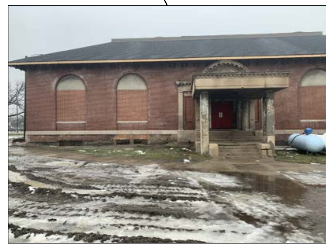
EXISTING BRICK INFILL TO REMAIN - TYPICAL
