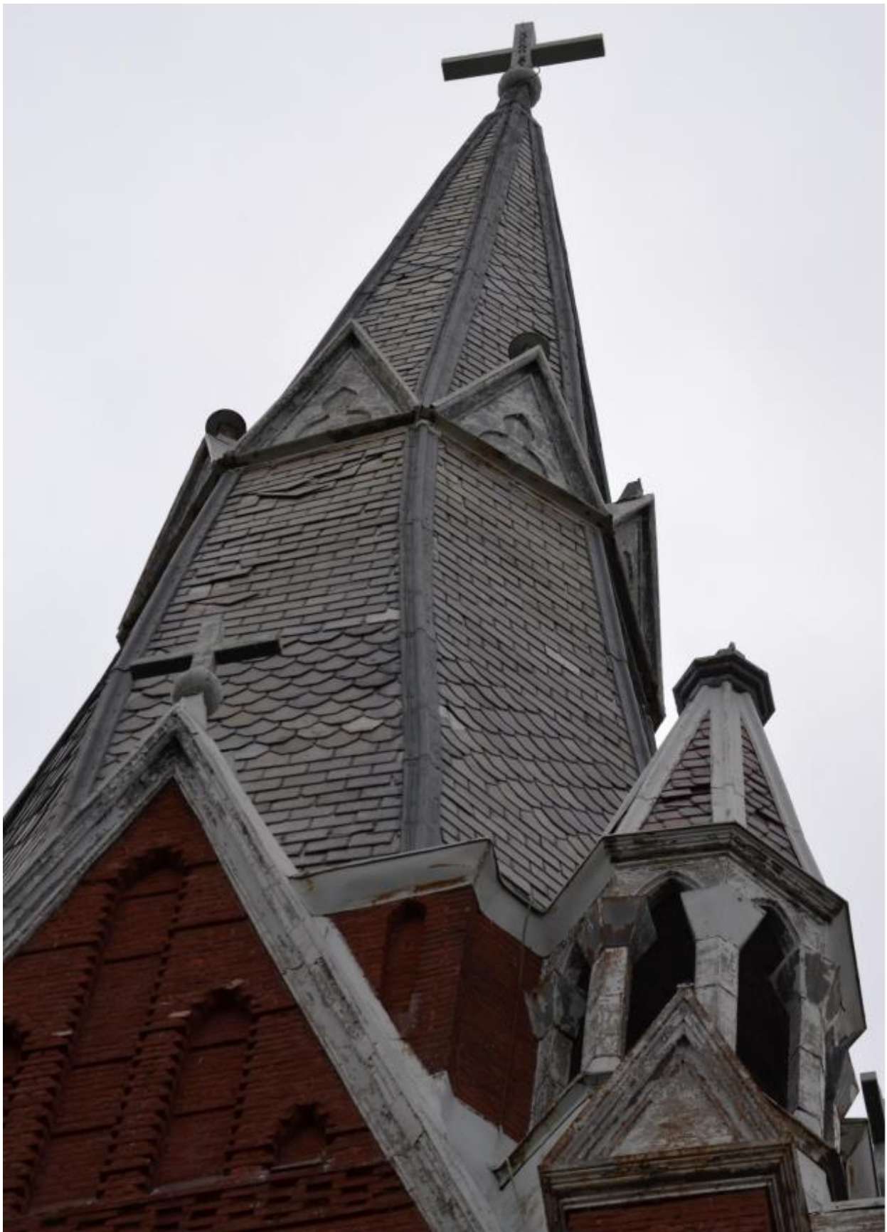
Photo provided by applicant, 2017, prior to steeple repair
