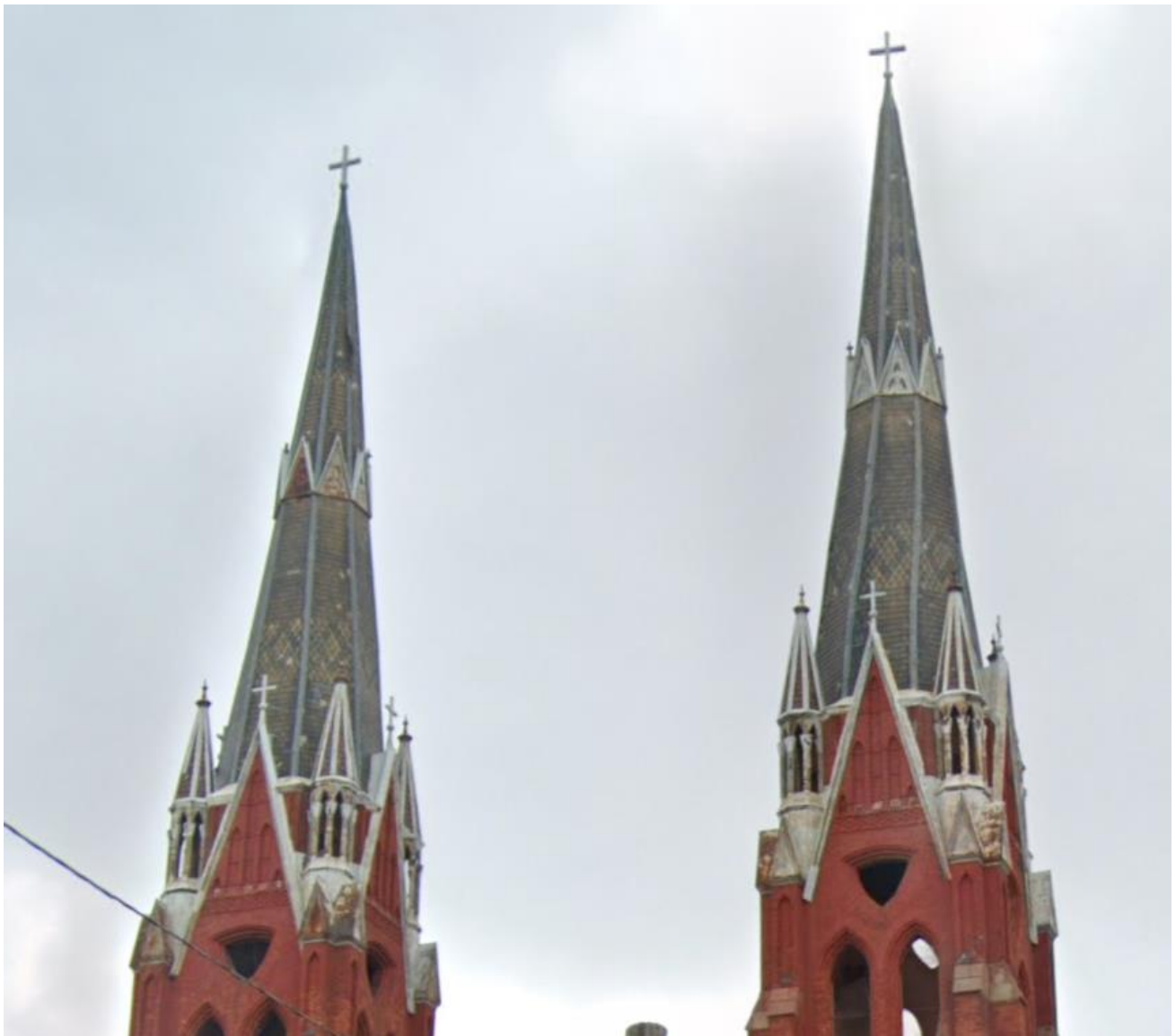
Google Streeview, August 2018, prior to steeple repair
