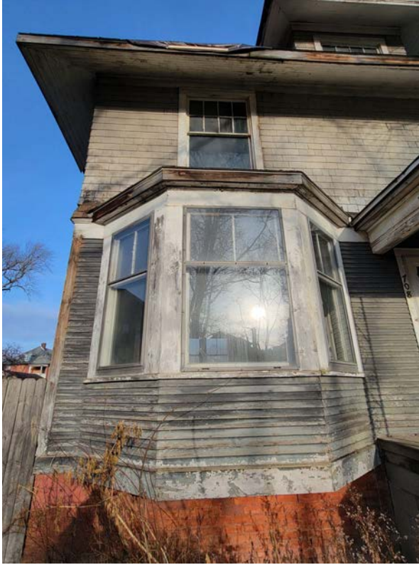
Front Bay Window Detail
