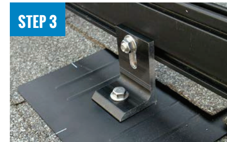
STEP 3 ATTACH L-FOOT TO RAIL
