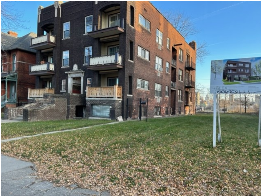
VIEW OF APARTMENT BUILDING 467 W ALEXANDRINE
