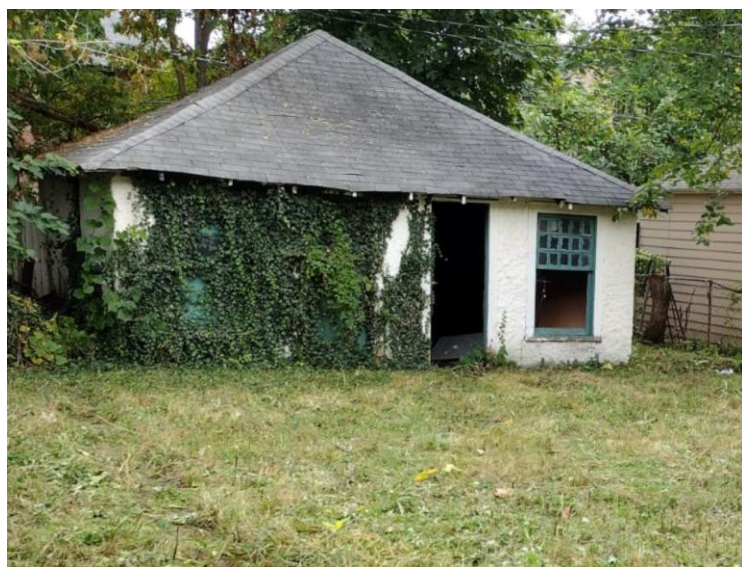
Current State of Garage
