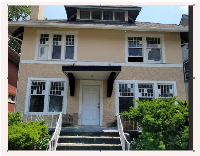
Current State of Front of House
