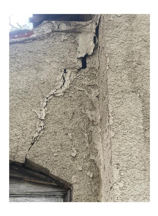
2. Clay blocks have fallen multiple inches and are resting on the window jambs and door. Failed attempts to block large air gaps in the past can be seen here.
