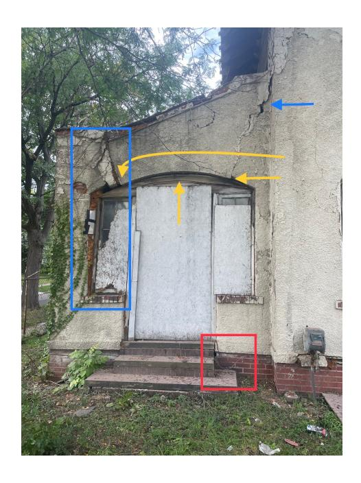
1. Masonry separated from the main house, clay blocks are sagging 1"+. The masonry above the doorway and window jambs is being held up by the wood framing below, causing the framing to buckle inwards.
