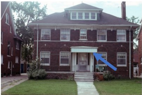
Photo 5 – 1974 image. Non-Historical materials and changes already made to the home
