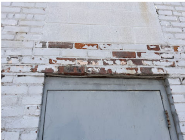
Steel lintel angle - over door exterior
