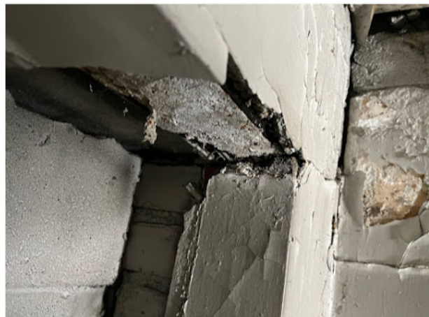
Steel lintel beam - over infilled vehicle door interior
