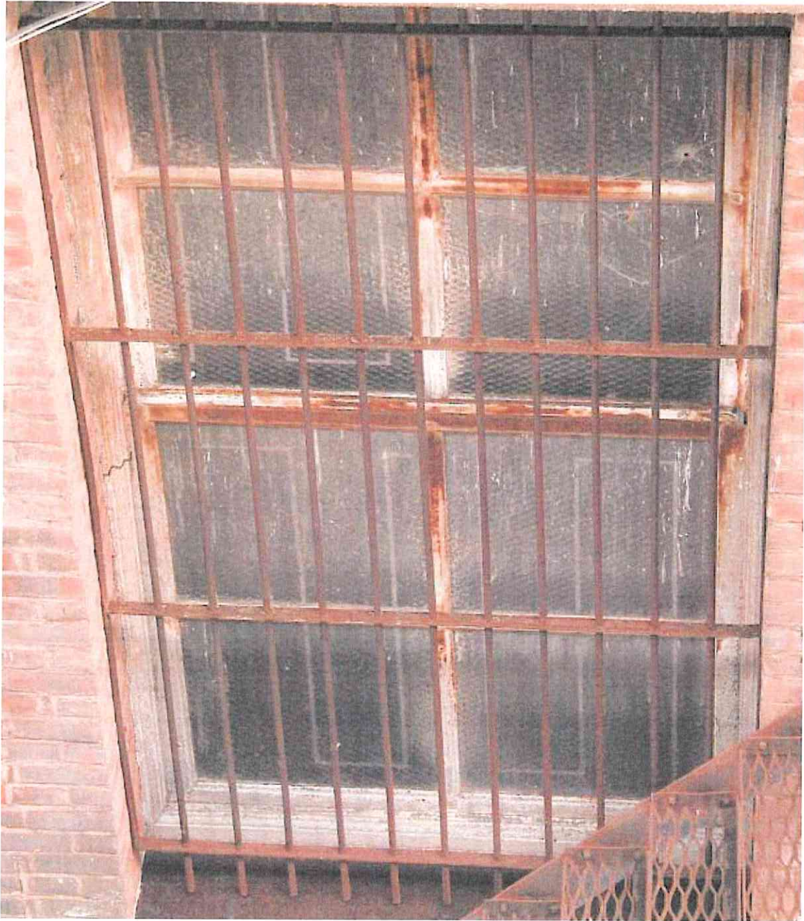
Exterior View of typical steel window
