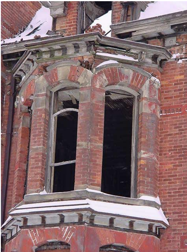
96-104 Edmund Place, the one remaining and visible sash. Notice the arched top.
