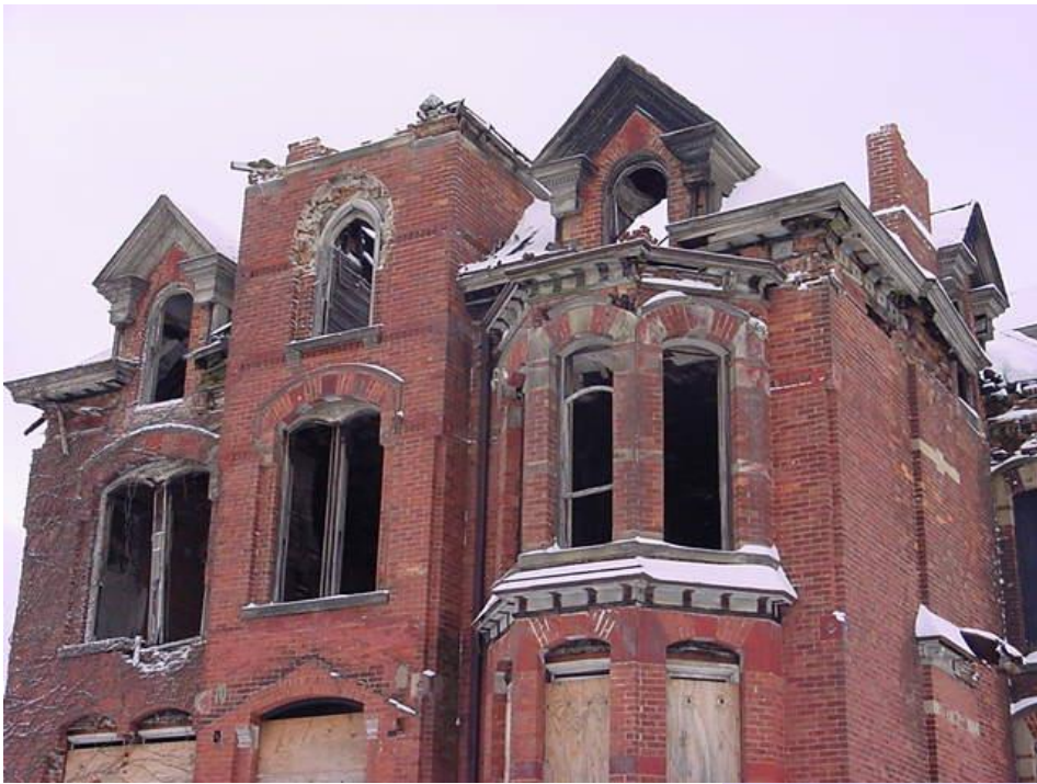
96-104 Edmund Place, detail of the second and third stories. Windows are proposed to be installed, masonry
