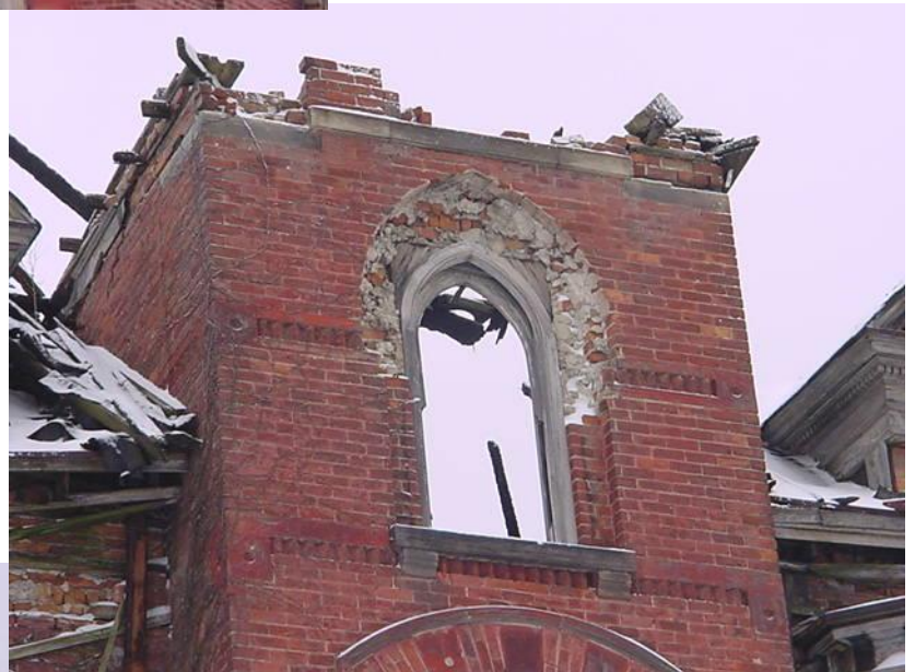
96-104 Edmund Place, third story tower that is proposed to be rebuilt with a convex roof and round window. Notice the brick detailing.
