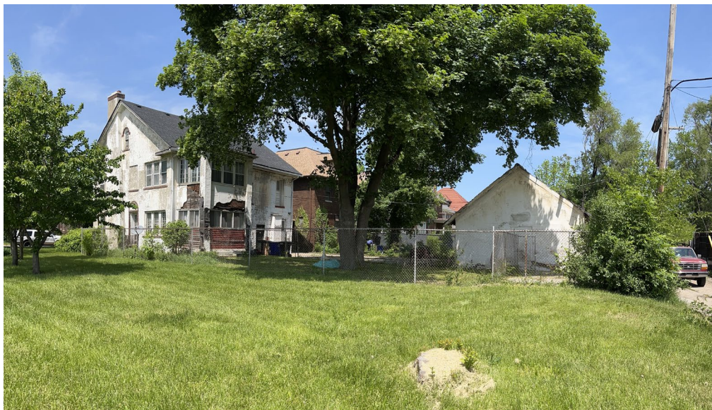
Side view of residence and existing garage from West
