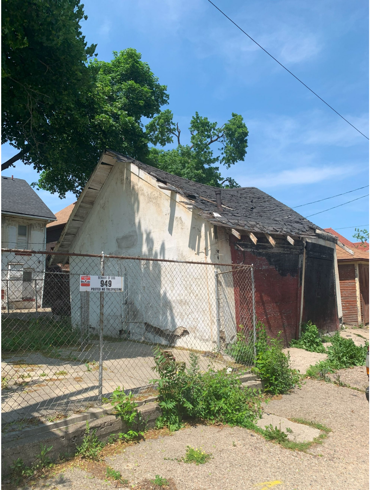
Rear / Side view of existing garage from South-West
