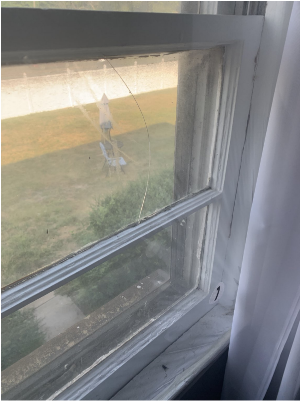
Interior view. Reel spring sash balance.
