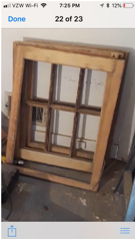
Stripped to bare wood
