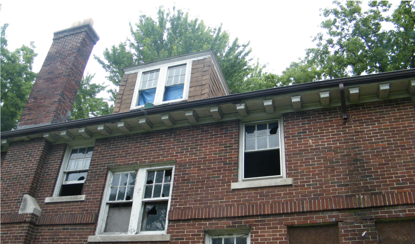
Exhibit Three: Dormer with Asphalt Shingle, 2013
