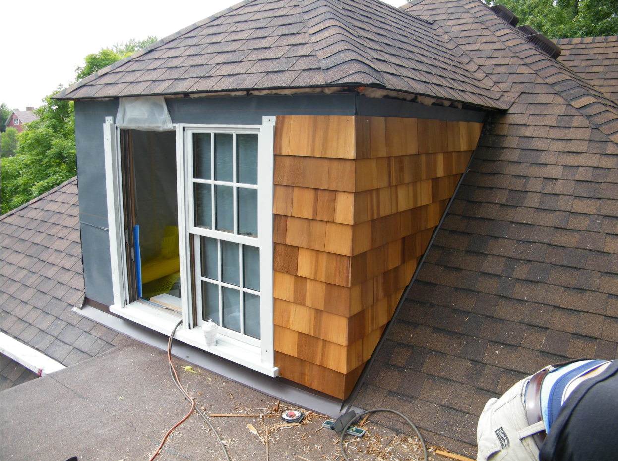
Exhibit Four: Cedar Shake Being Installed on Dormers, 2013
