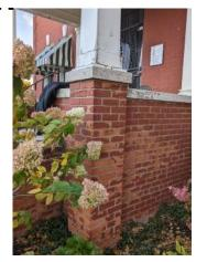
EXISTING COLUMN BASE SPALLING MASONRY PAINT
