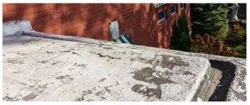
MULTIPLE LAYERS OF DECAYED ROOFING, LEAKING INTEGRAL GUTTER, INADEQUATE GUTTER DEPTH, DECAYED WALL COUNTERFLASH
