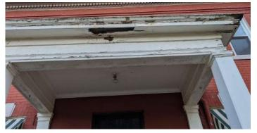
MODIFIED OVERHANGS WITH DECAYED SOFFITS AND FASCIA, EXISTING PORCH CEILING AND LIGHT
