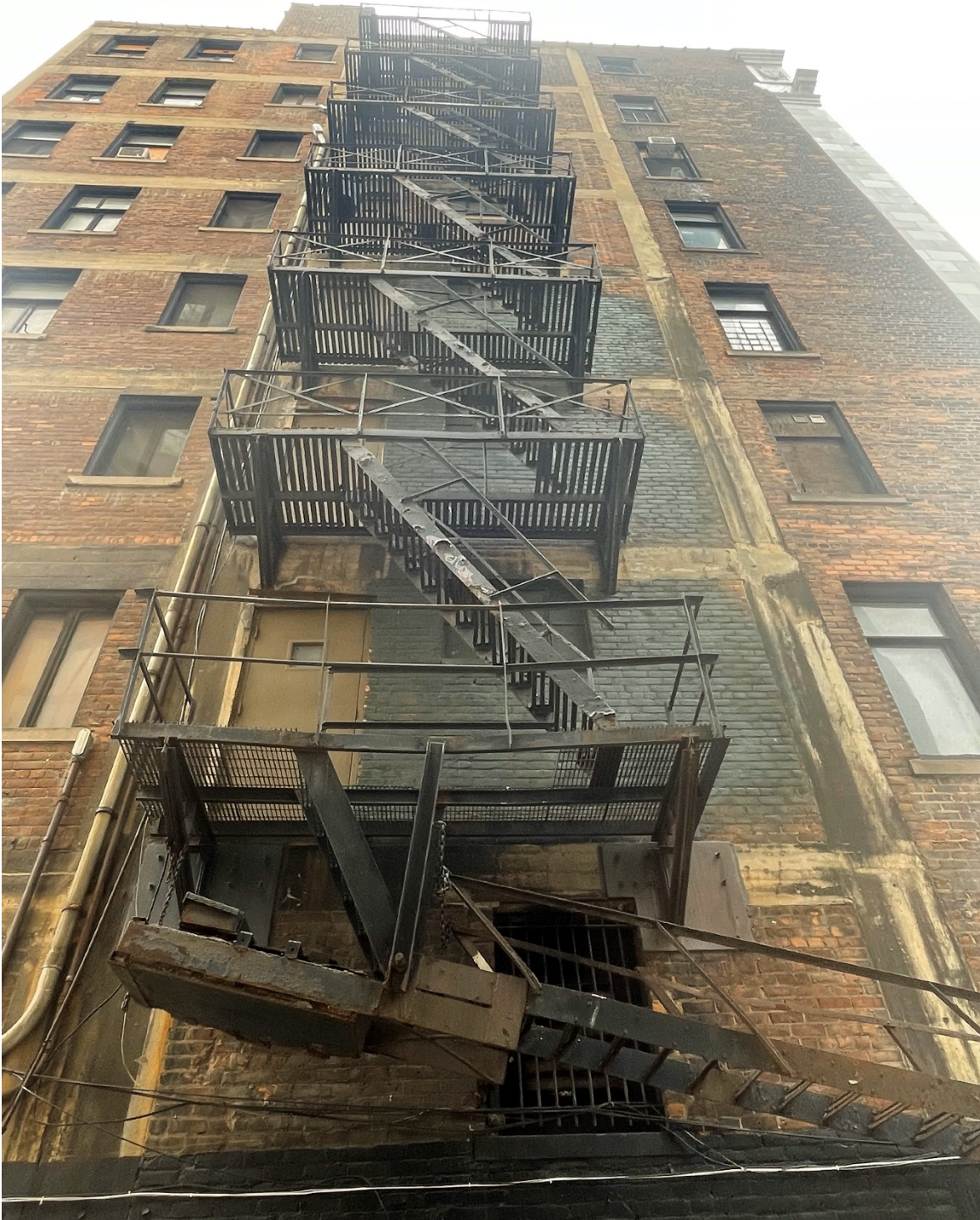
5. Exterior, East elevation, Detail of Existing Fire Escape, Looking northwest. 4/17/23.
