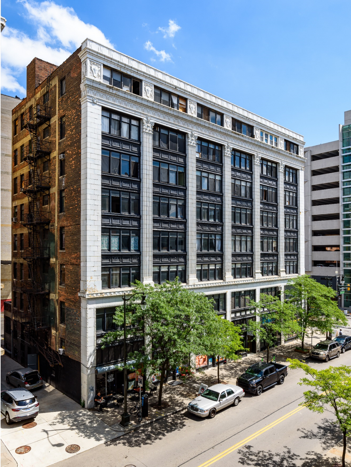
2. Exterior, North elevation, Looking southwest. c. 2022.
