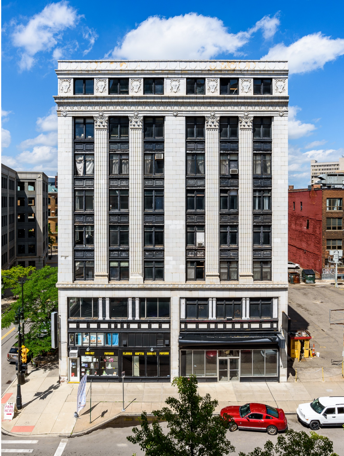
1. Exterior, West Elevation, Looking East. c. 2022.
