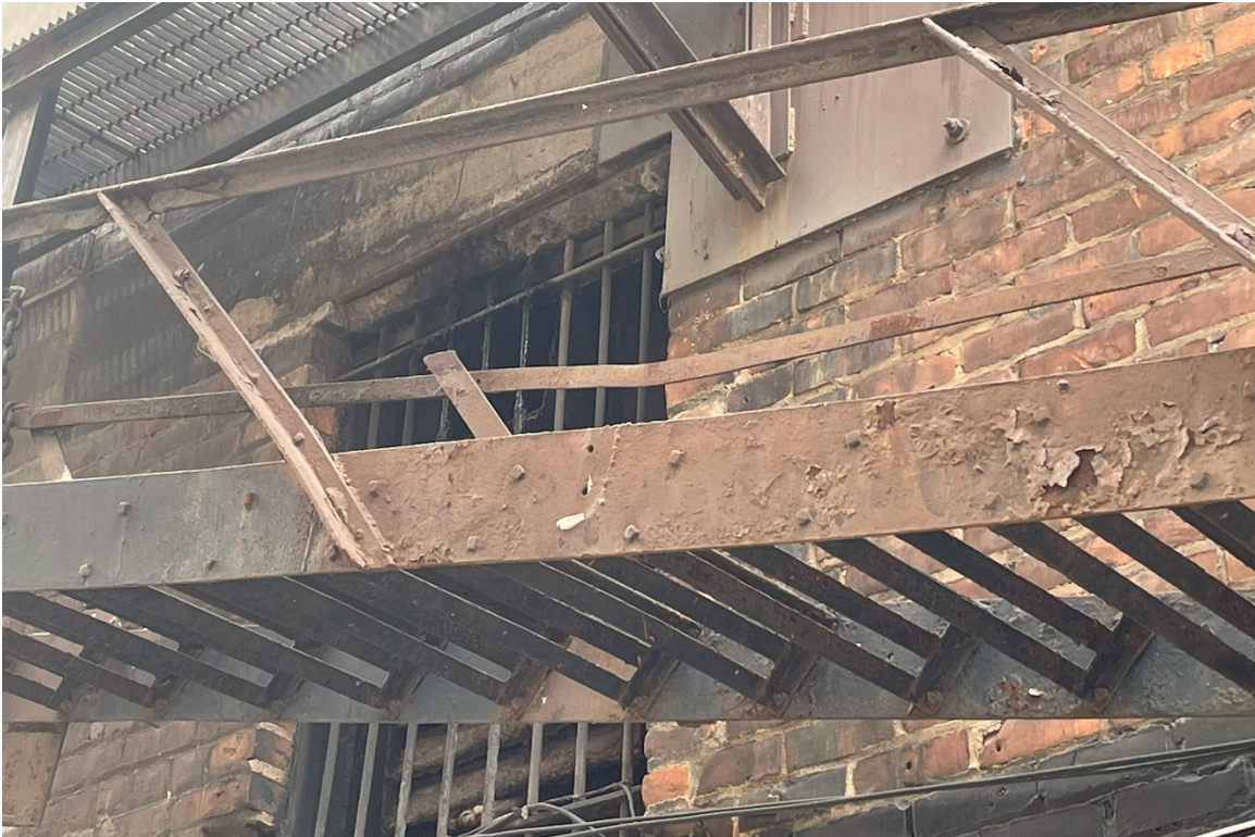
6. Exterior, Detail of Existing Fire Escape, Looking west. 4/17/23.
