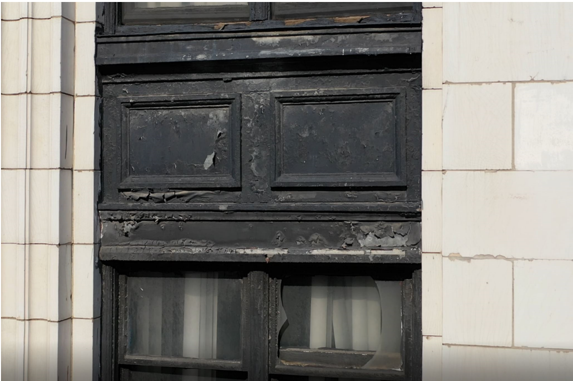
7. Exterior, North Elevation, Typical spandrel panel condition. 4/5/23.
