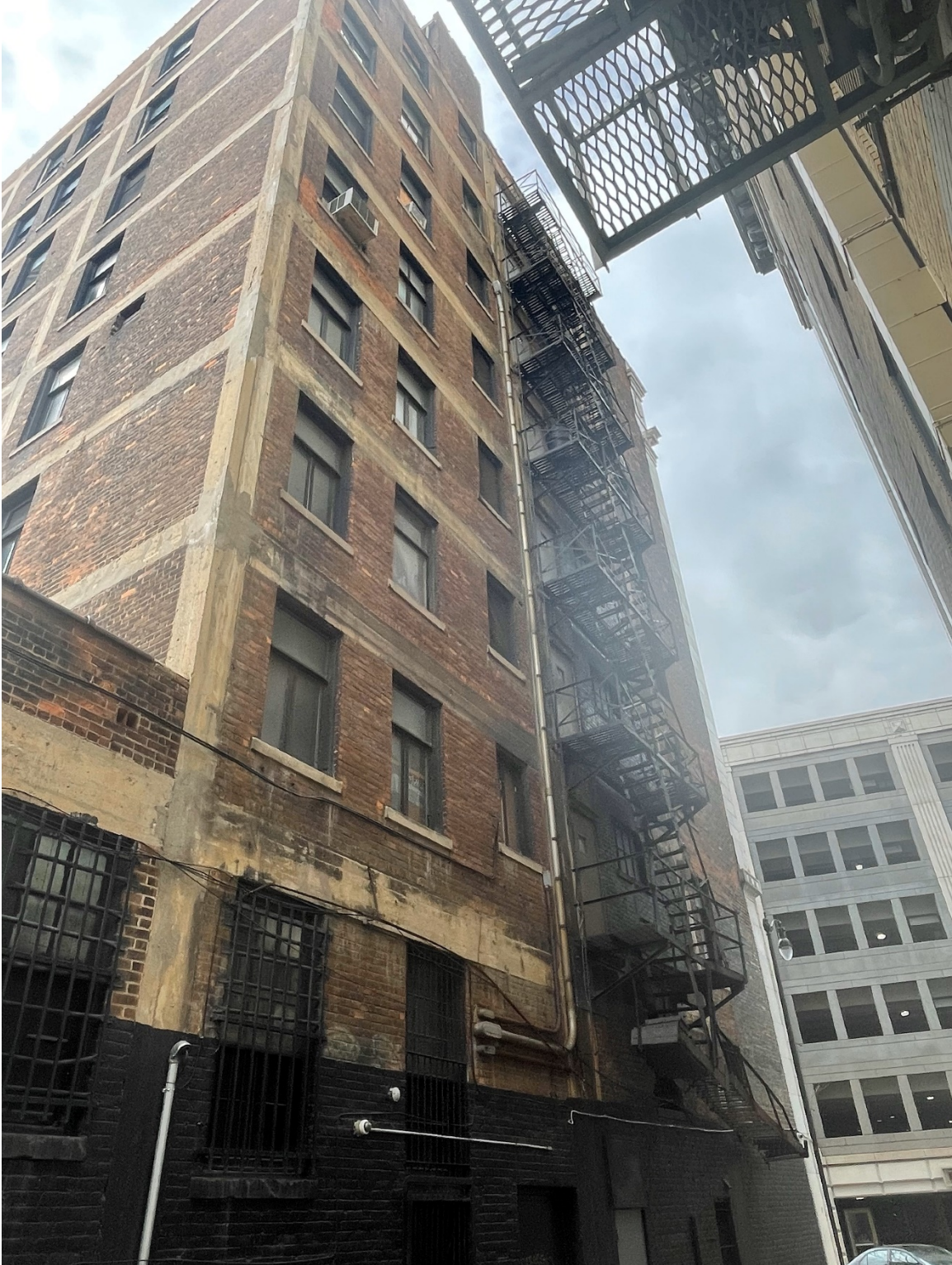
4. Exterior, East elevation, Looking northwest. c. 2022.
