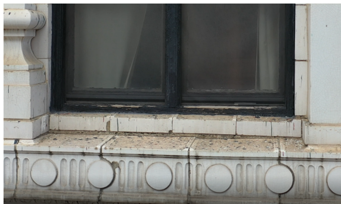
P-5 Lower water table in good condition along Broadway Street
