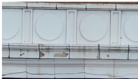
P-3 Spalling and cracking terra-cotta at upper water table
