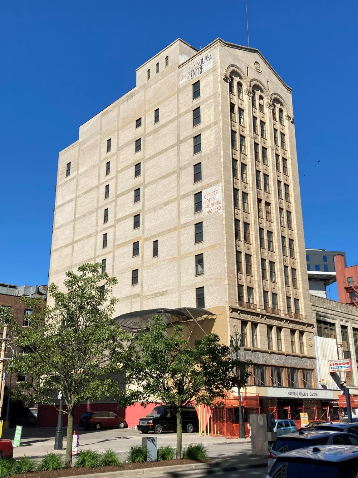
South and west elevations from Broadway
