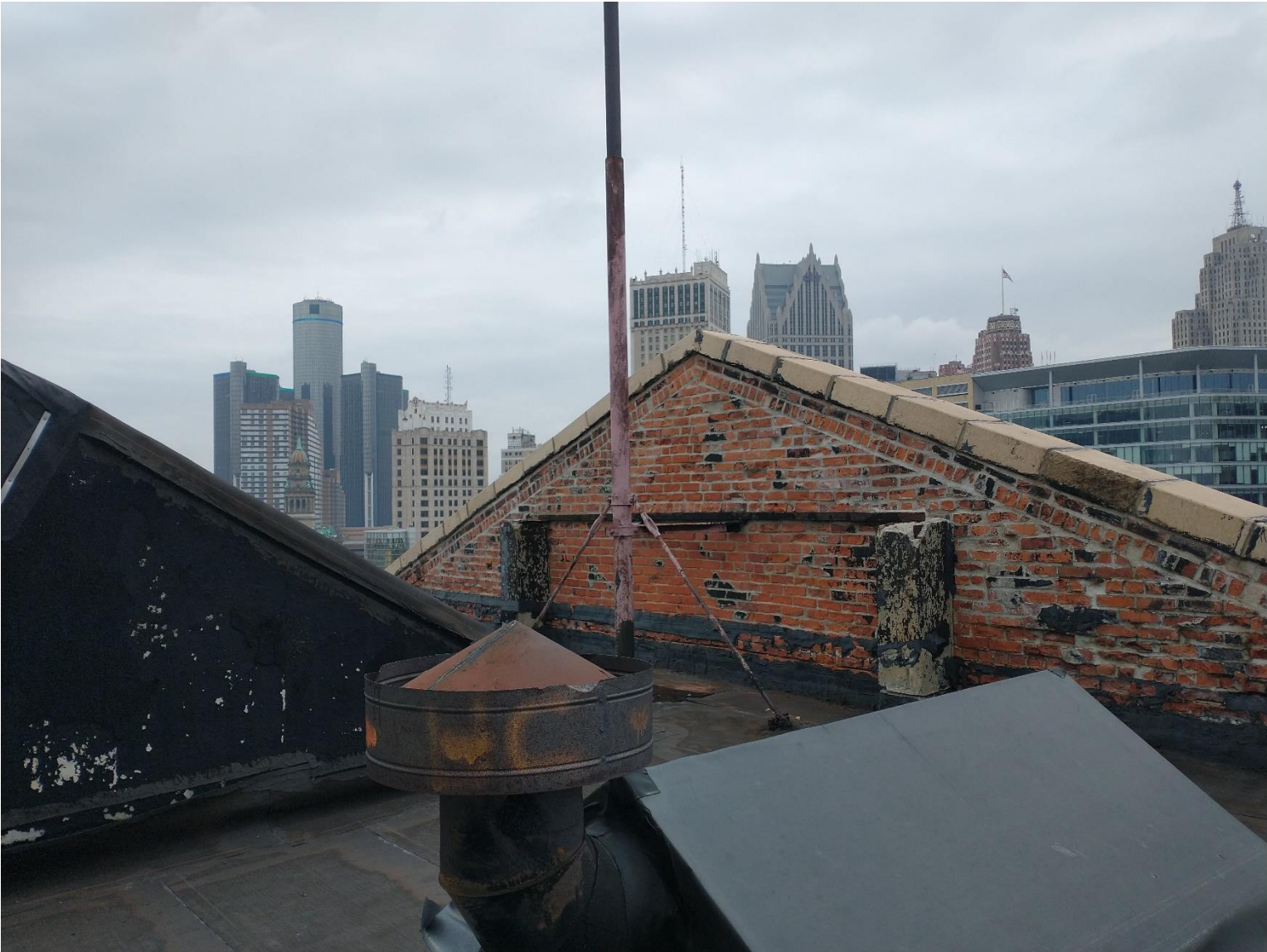
Masonry parapet above façade, looking south
