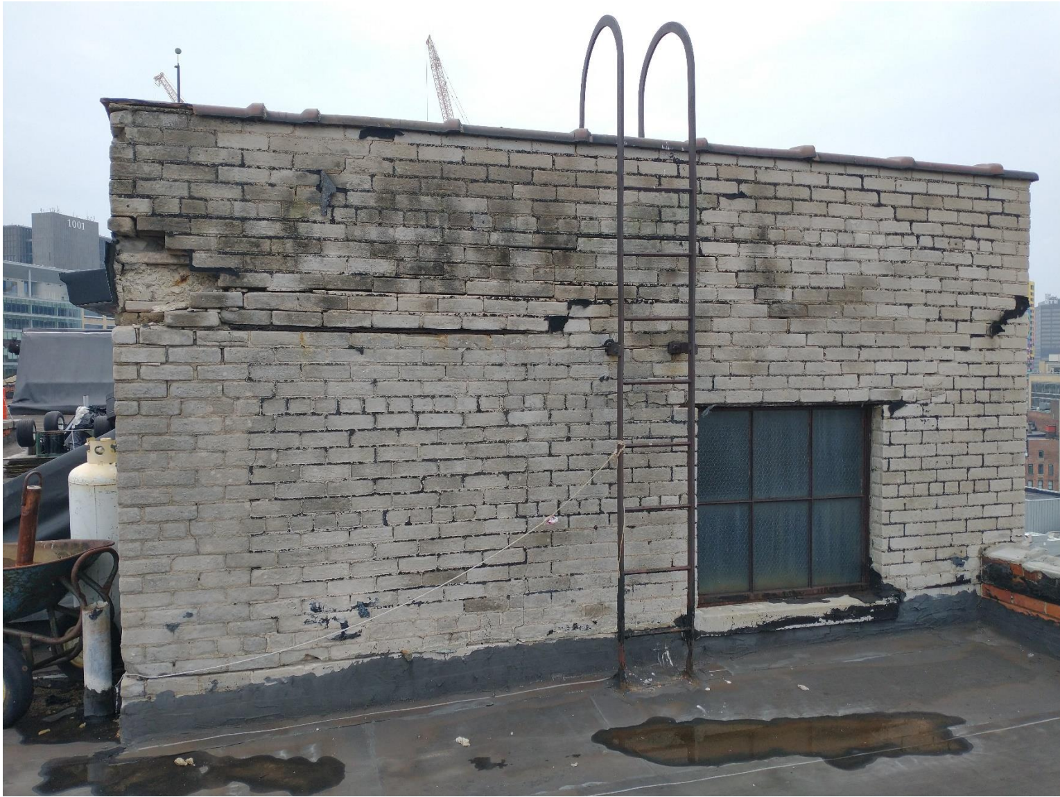
View of rear of penthouse, looking south
