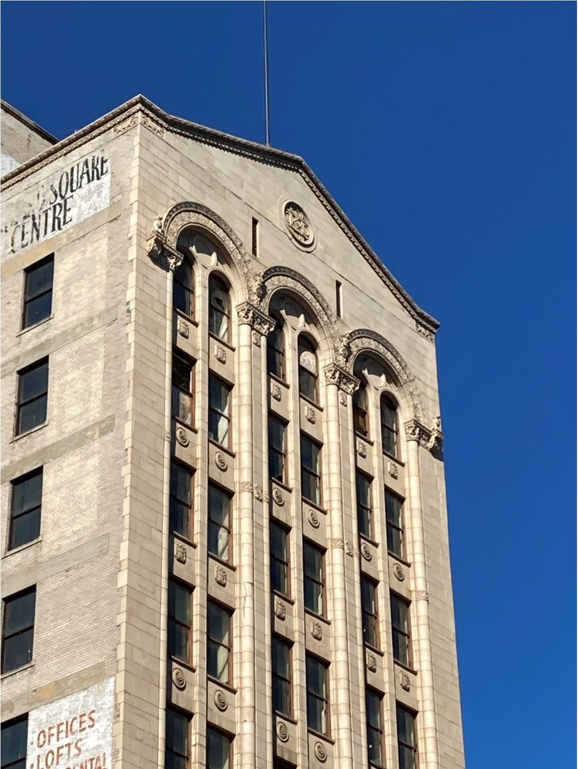
Upper portion of façade
