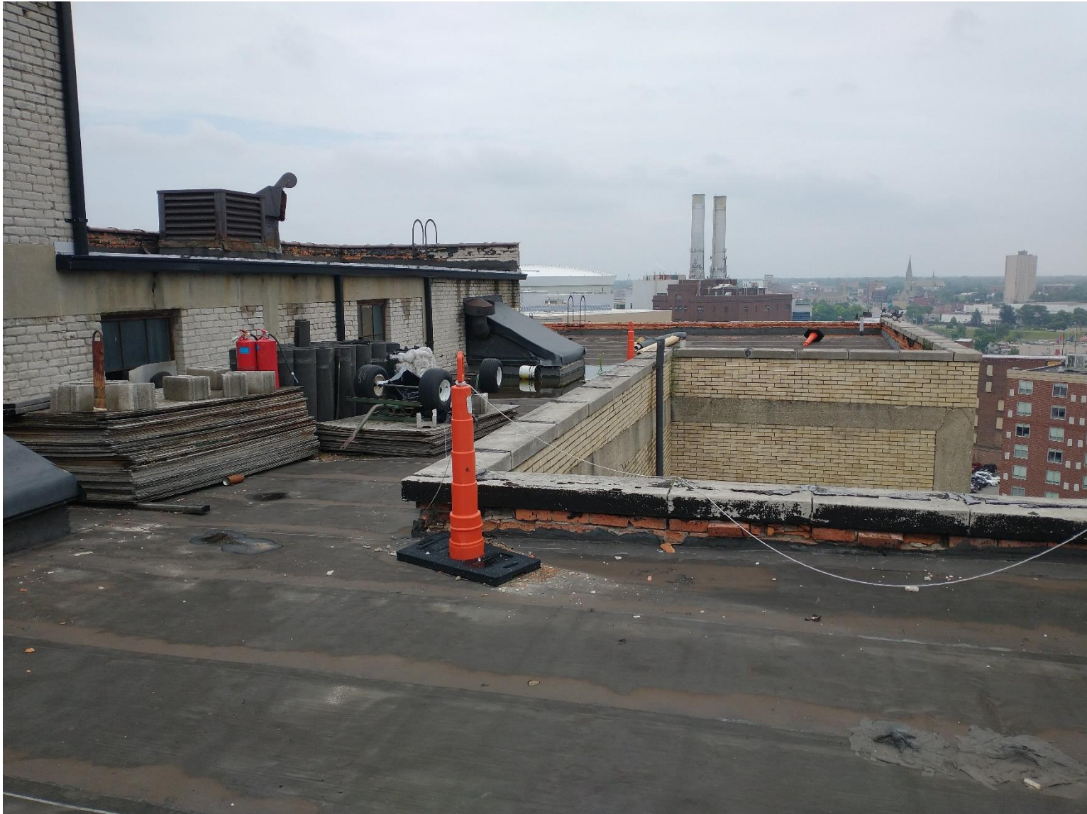
View of roof and penthouse, looking north
