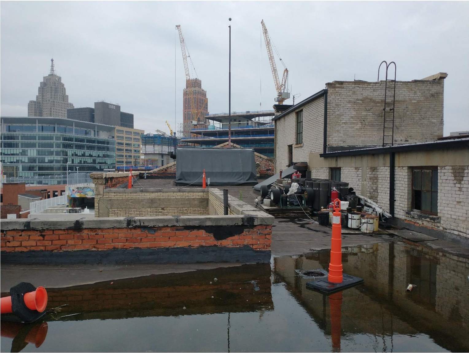
View of roof and penthouse, looking south
