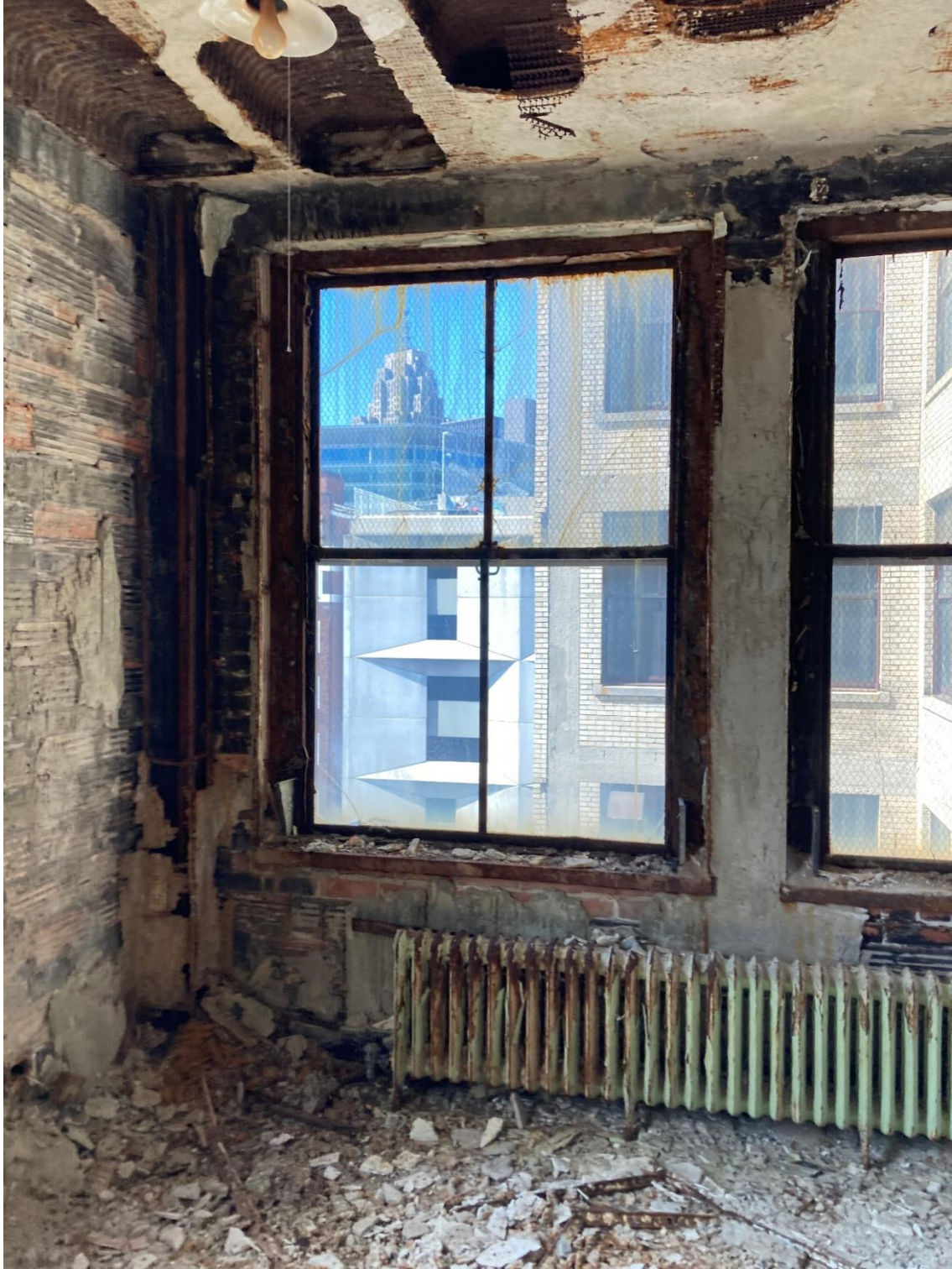
Interior view of typical cold rolled steel double-hung frame and sash, to be replaced
