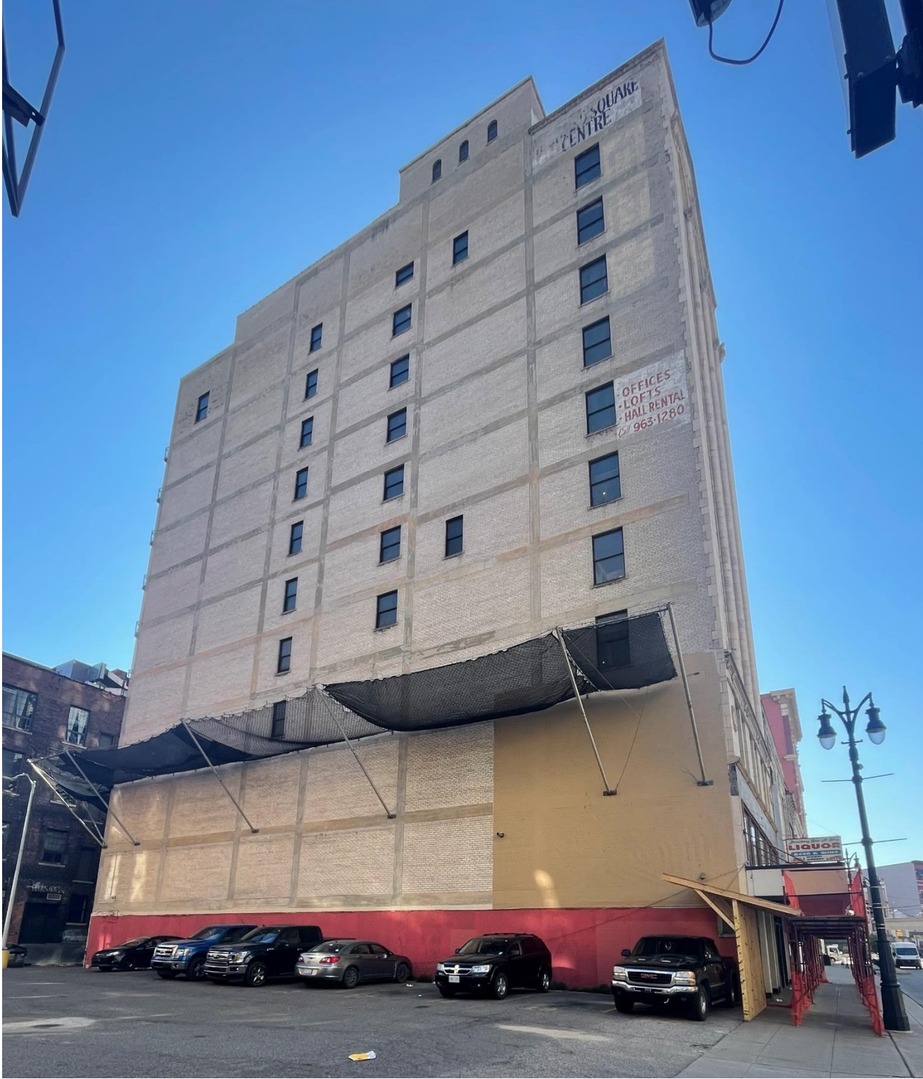
West elevation from parking lot to the west of the building
