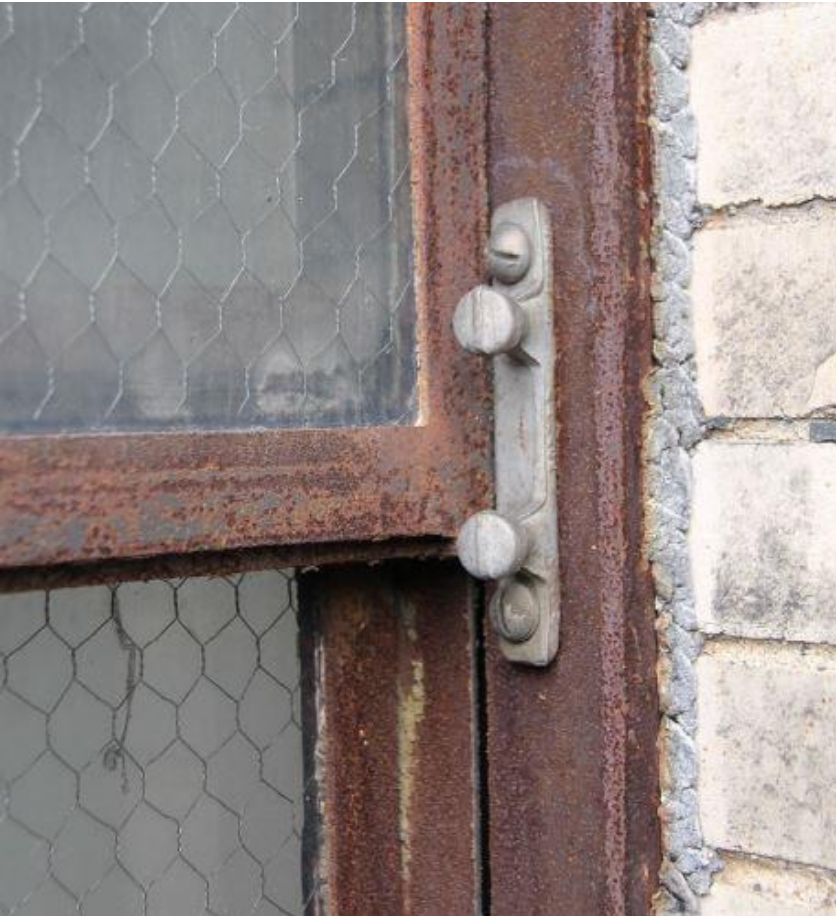
Typical cold rolled steel double-hung frame and sash, to be replaced
