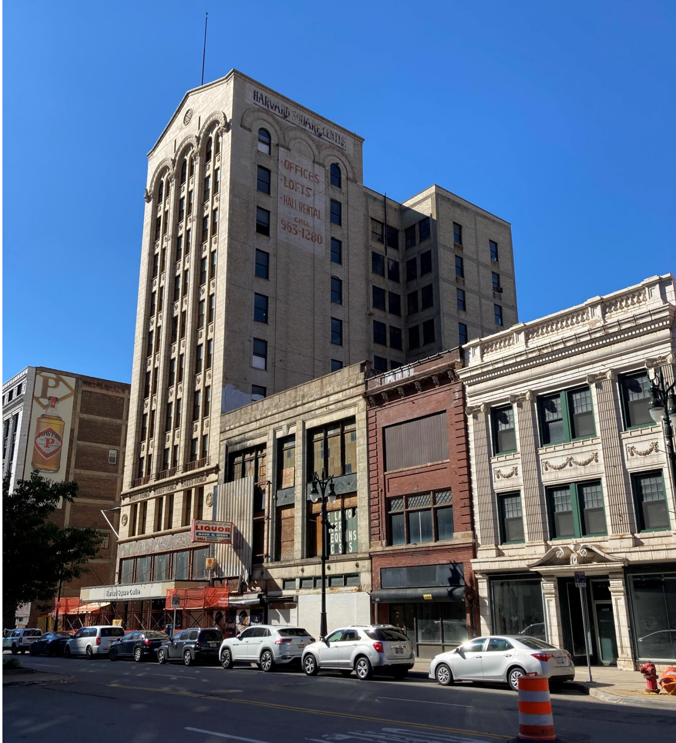
South and east elevations from Broadway
