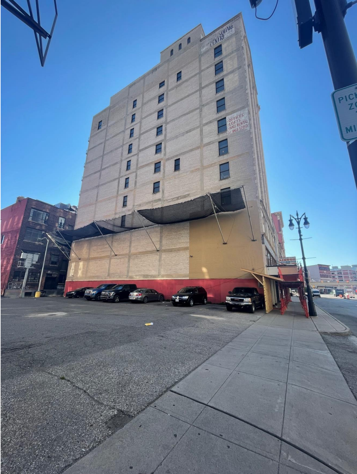
2. West elevation, Looking east. 06/23/22.
