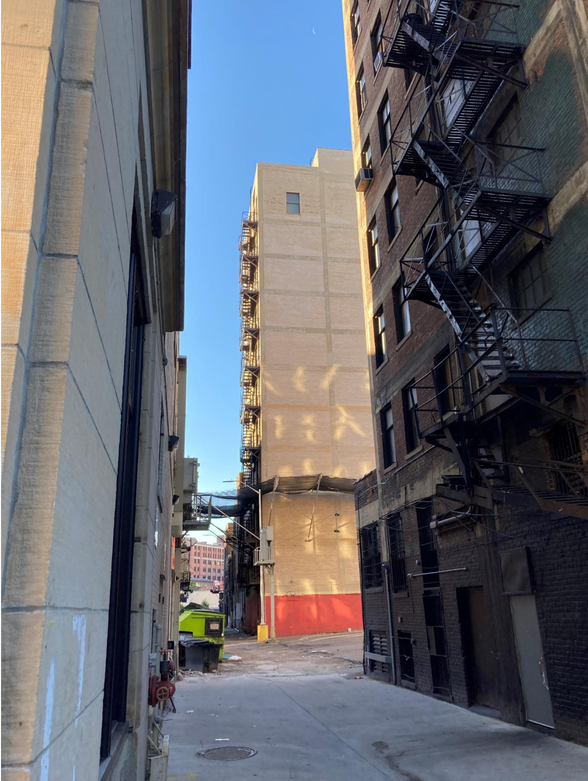
5. West elevation from alley, Looking east. 06/23/22.
