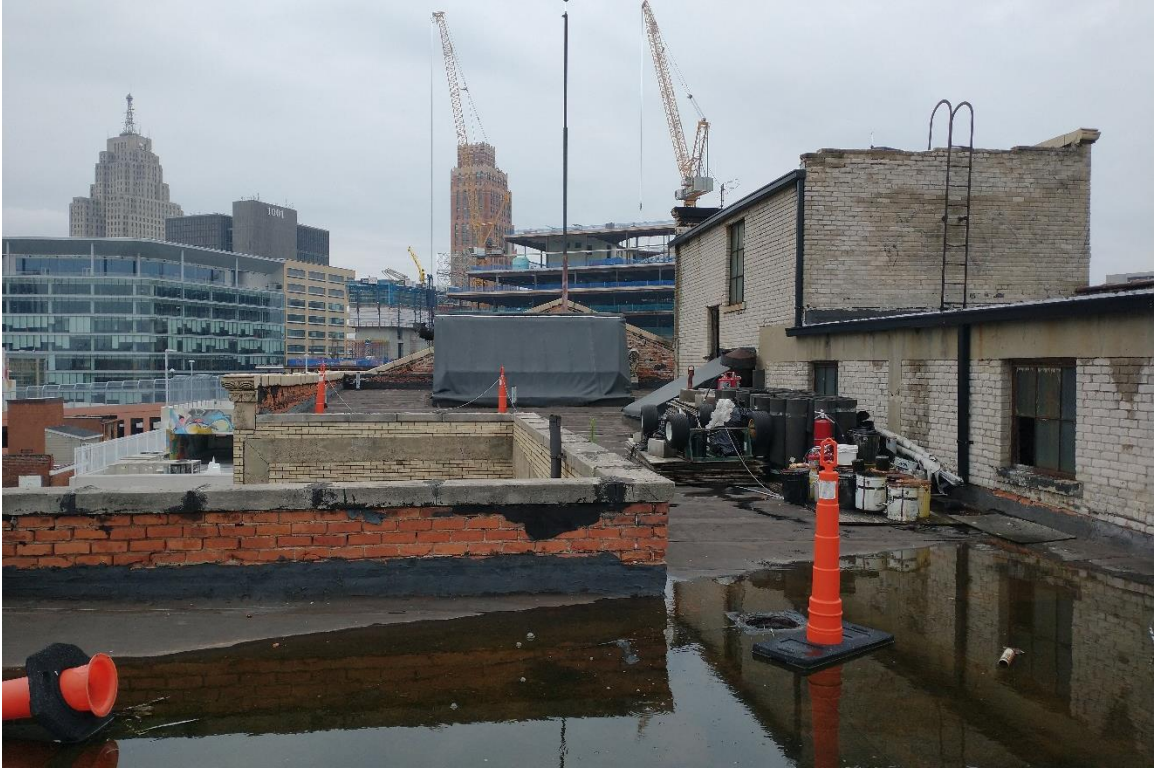
16. Rooftop and penthouse, Looking south. 06/23/22.
