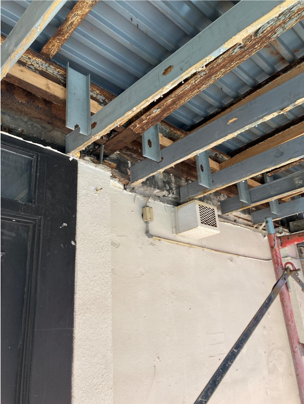
11. Underside of canopy on façade, Looking northeast. 06/23/22.
