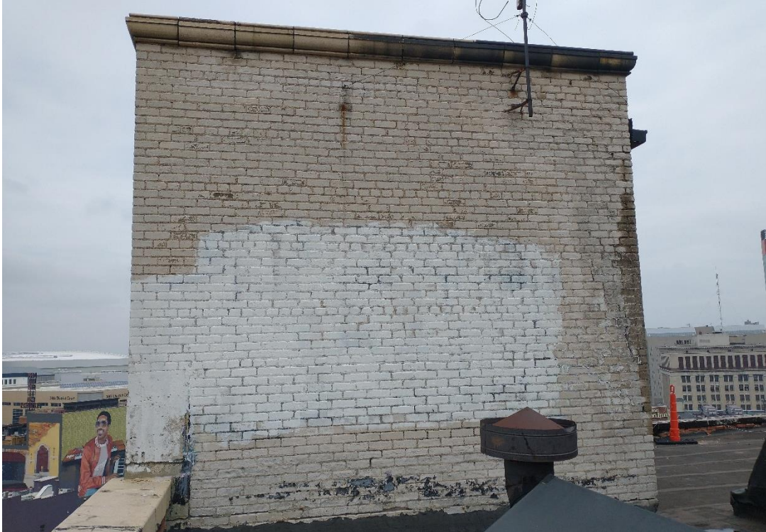
13. South elevation of rooftop penthouse, Looking north. 06/23/22.
