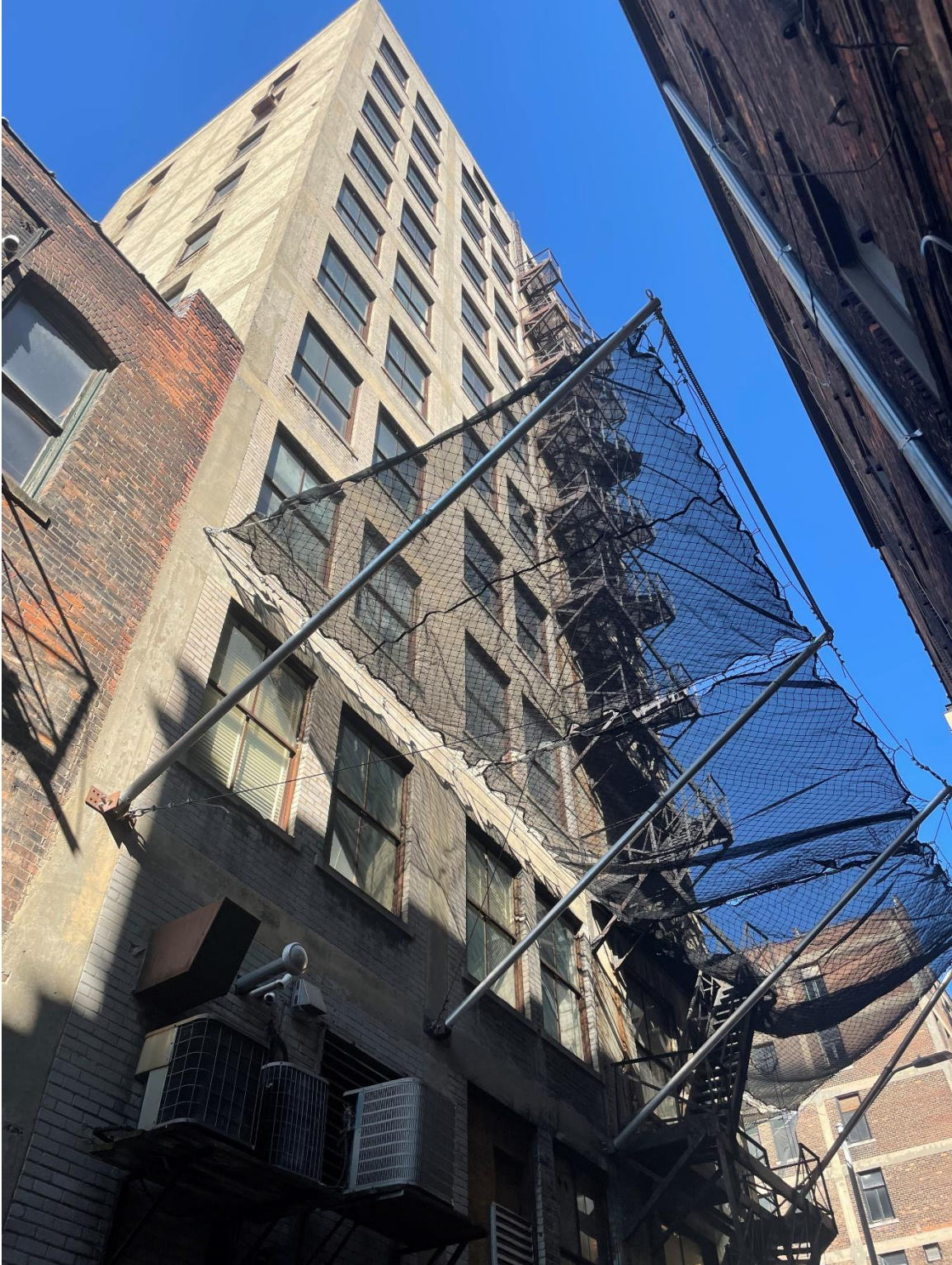
4. North elevation, Looking southwest. 06/23/22.
