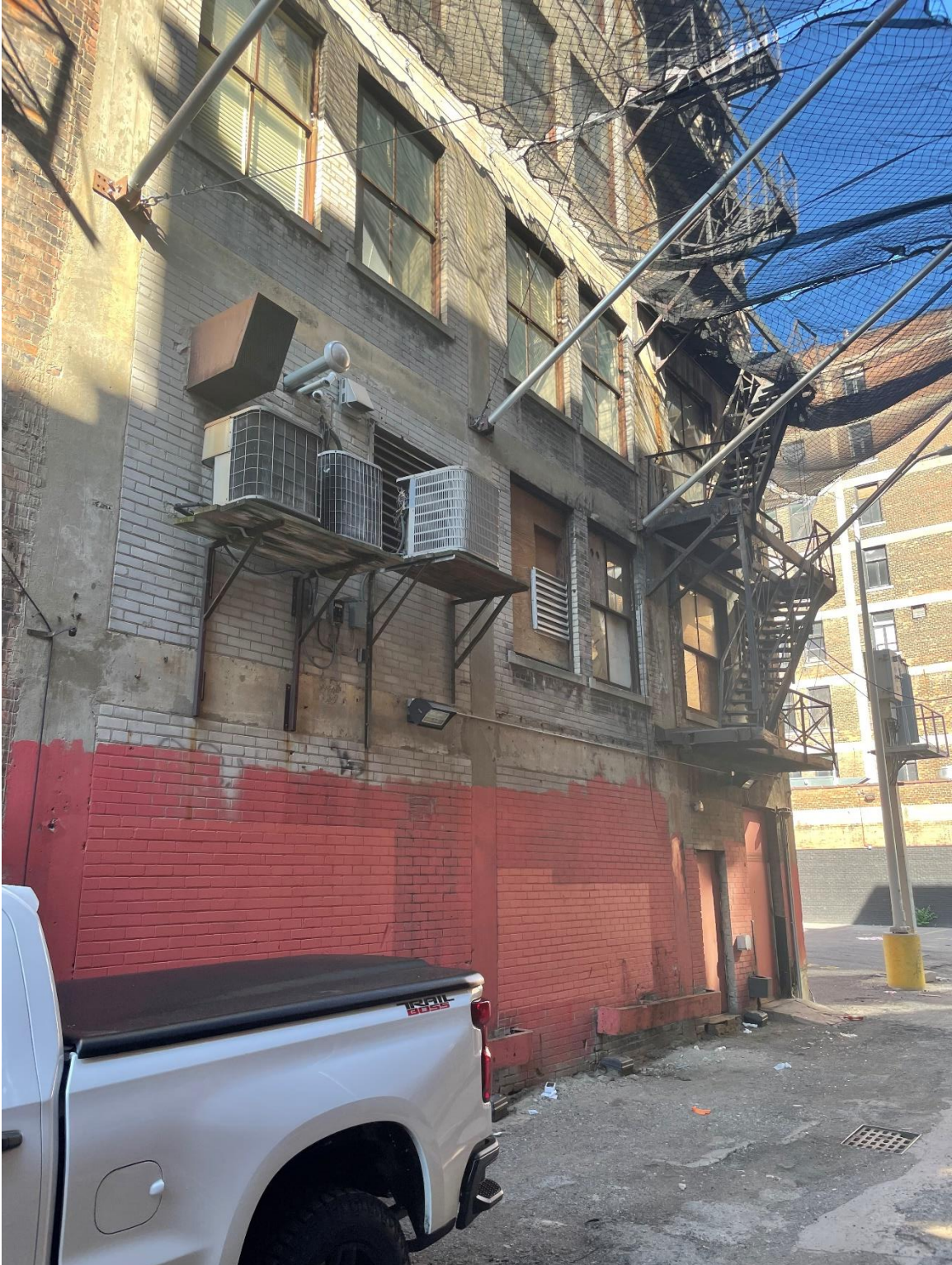
6. North elevation, Looking southwest. 06/23/22.
