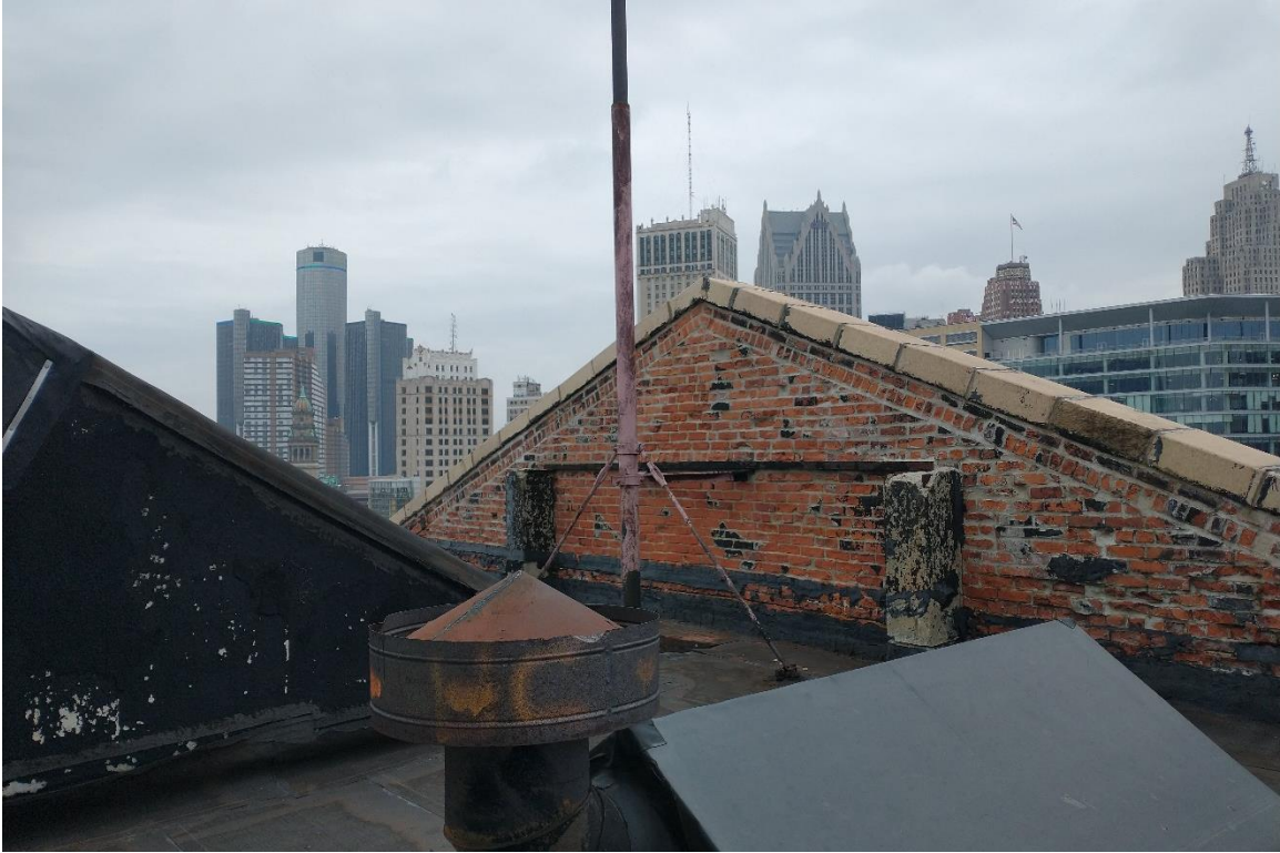
12. Rooftop and gabled masonry parapet above south facade, Looking southeast. 06/23/22.
