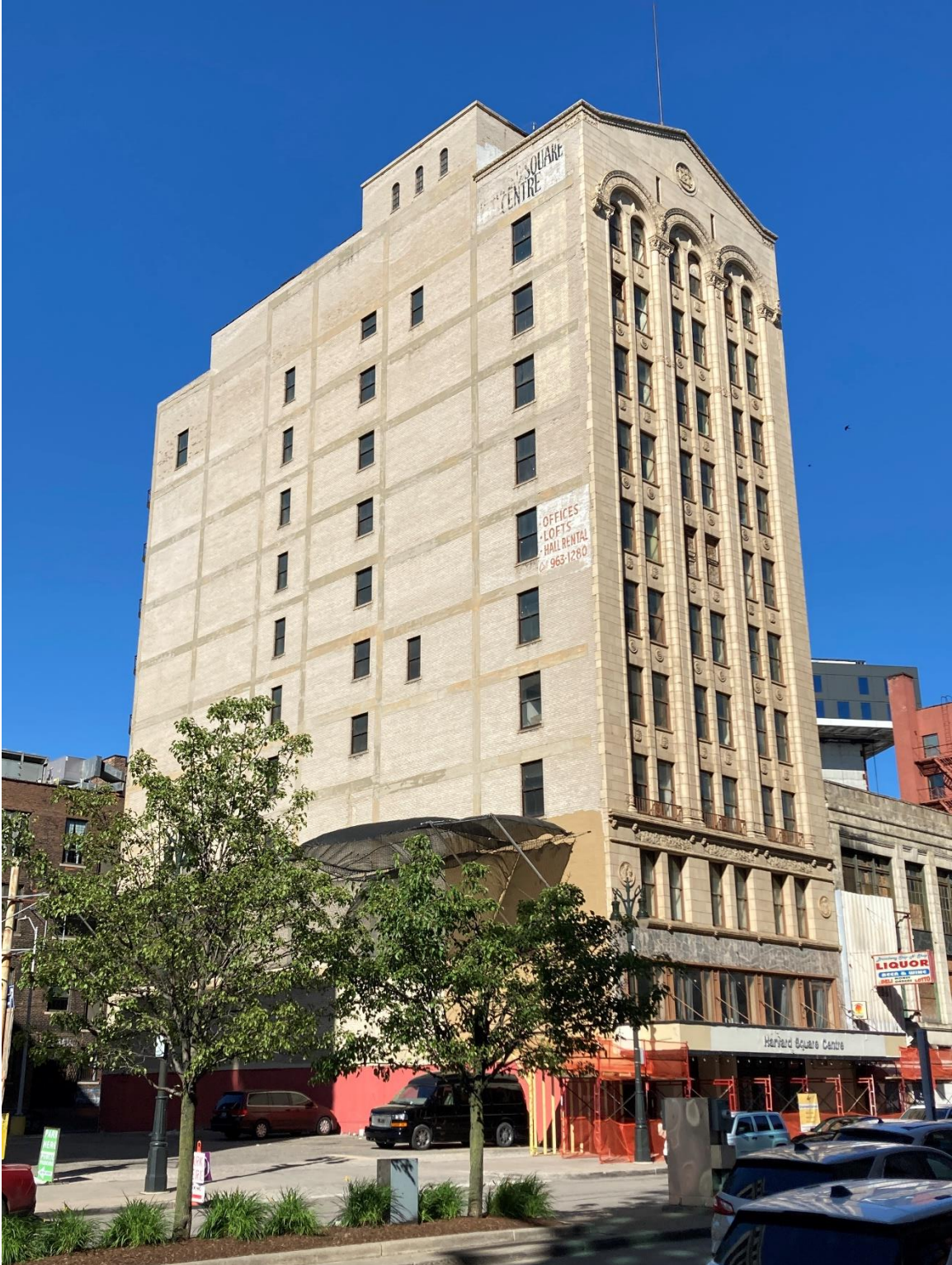
1. South and west elevations, Looking northeast. 06/23/22.
