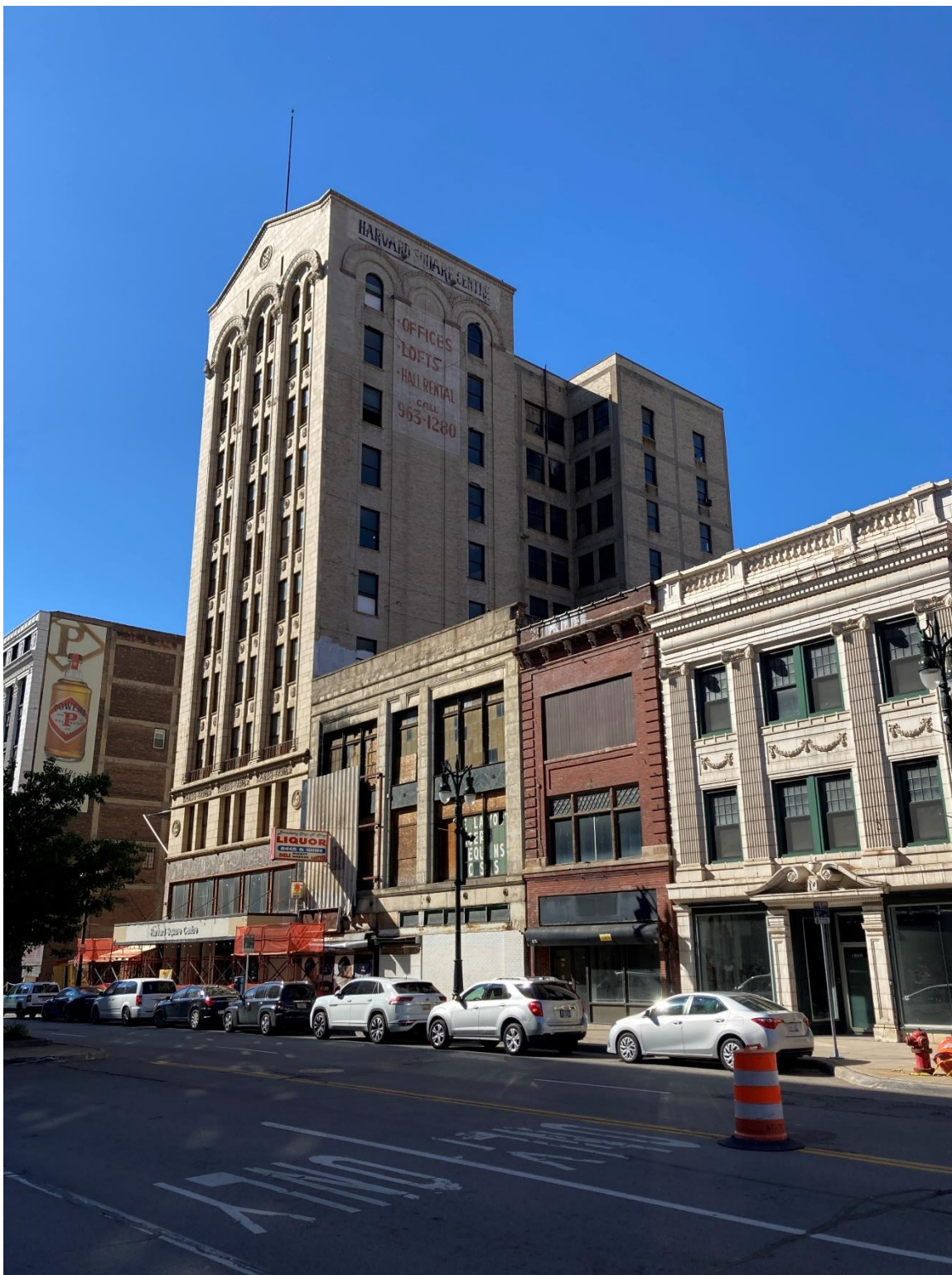
3. South and east elevations, Looking northwest. 06/23/22.
