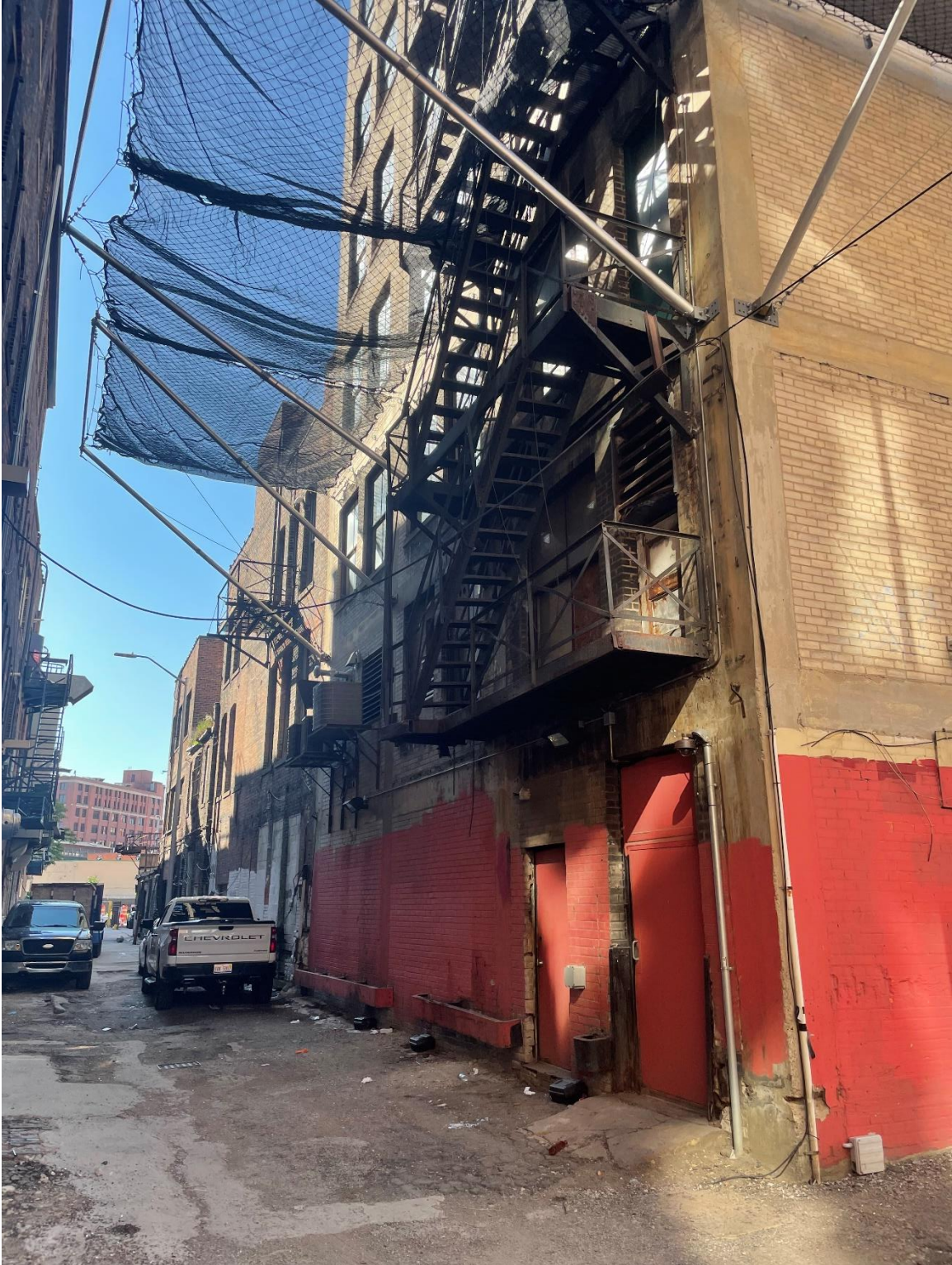
7. North elevation, Looking southeast. 06/23/22.
