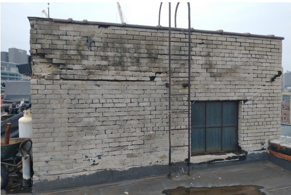
17. North elevation of rooftop penthouse, Looking south. 06/23/22.
