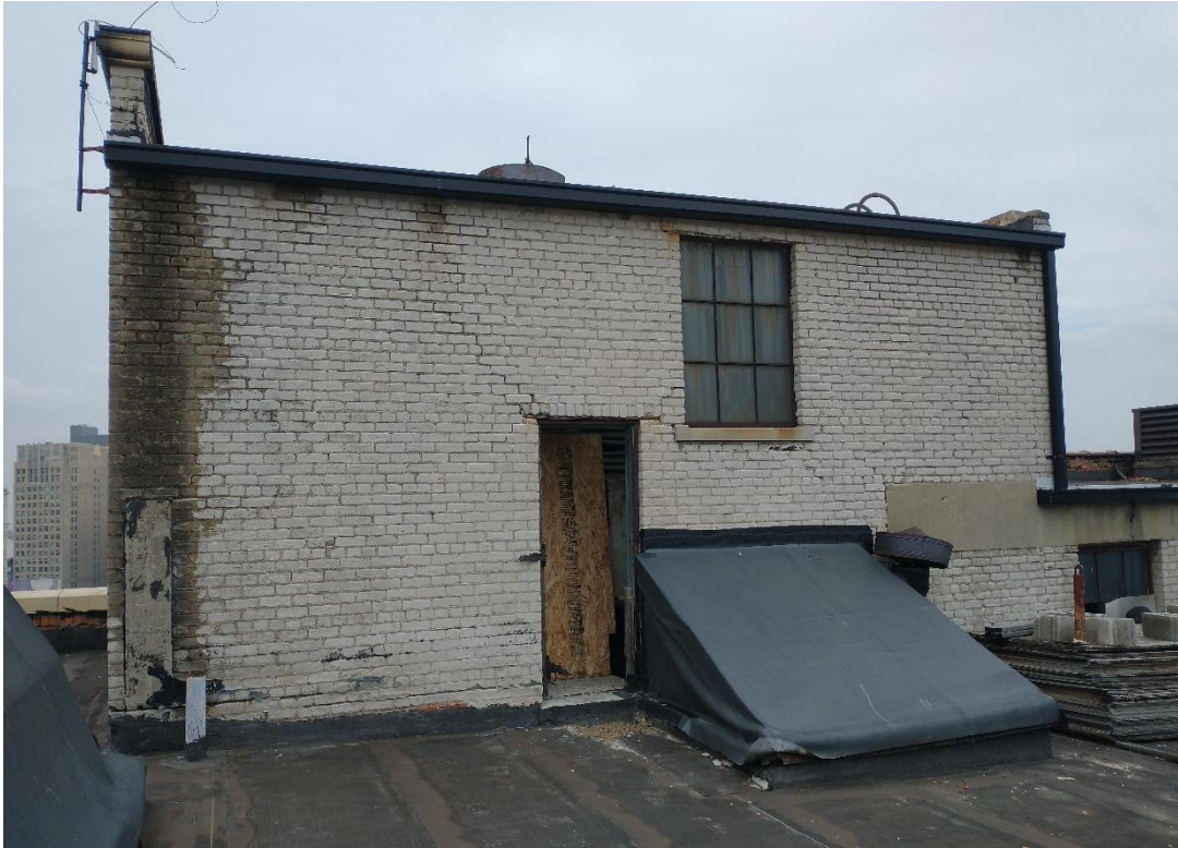
14. East elevation of rooftop penthouse, Looking west. 06/23/22.
