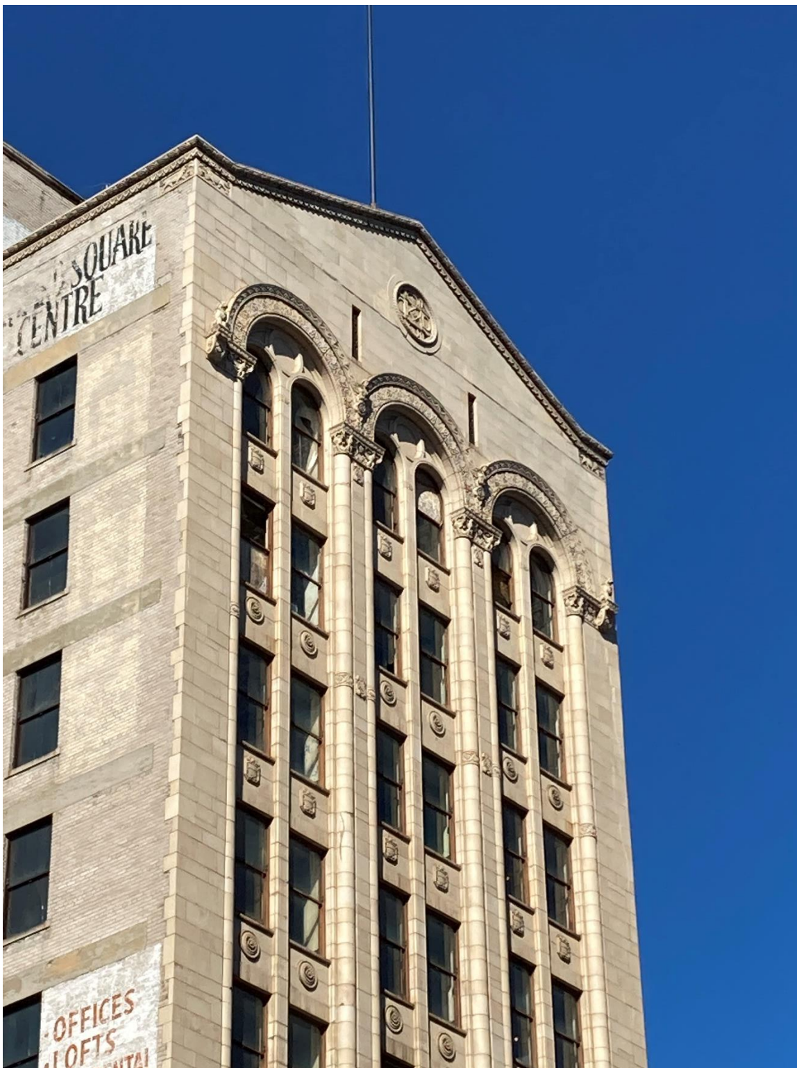
10. Upper portion of south elevation (facing Broadway), Looking northeast. 06/23/22.
