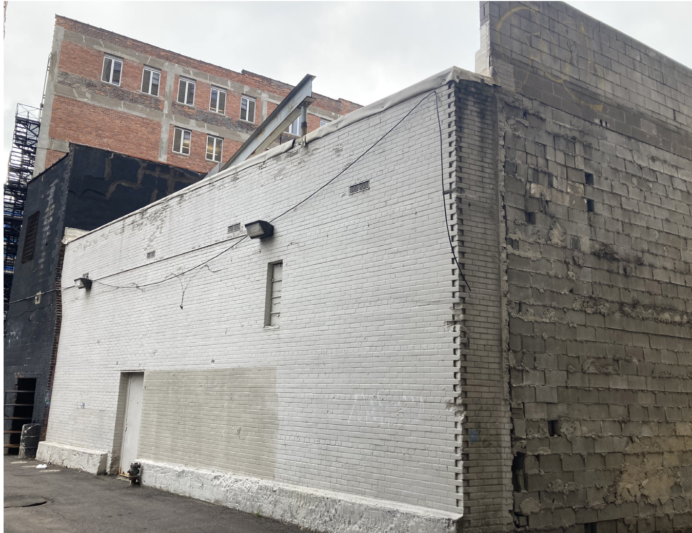
EAST FACADE (ALLEY)
