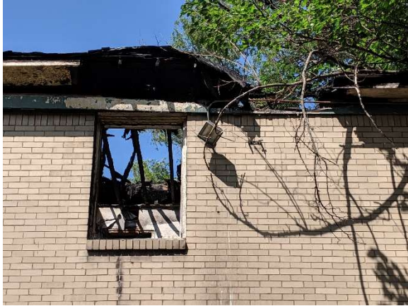
Photo 18: Roof at the northeast wing of the building.
