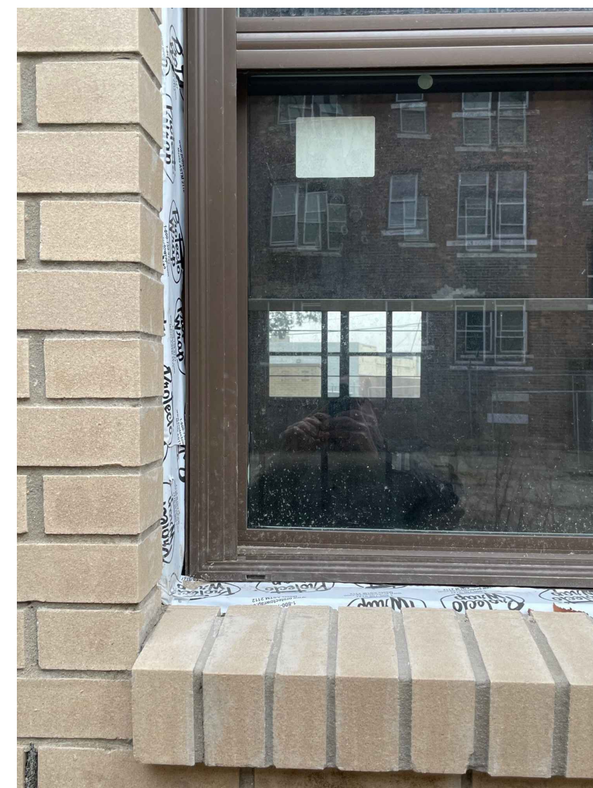
window view at rebuilt areas
