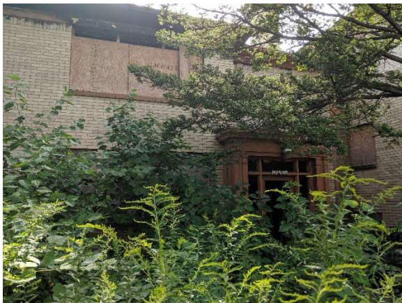
Photo 13: Partial east elevation at west courtyard
