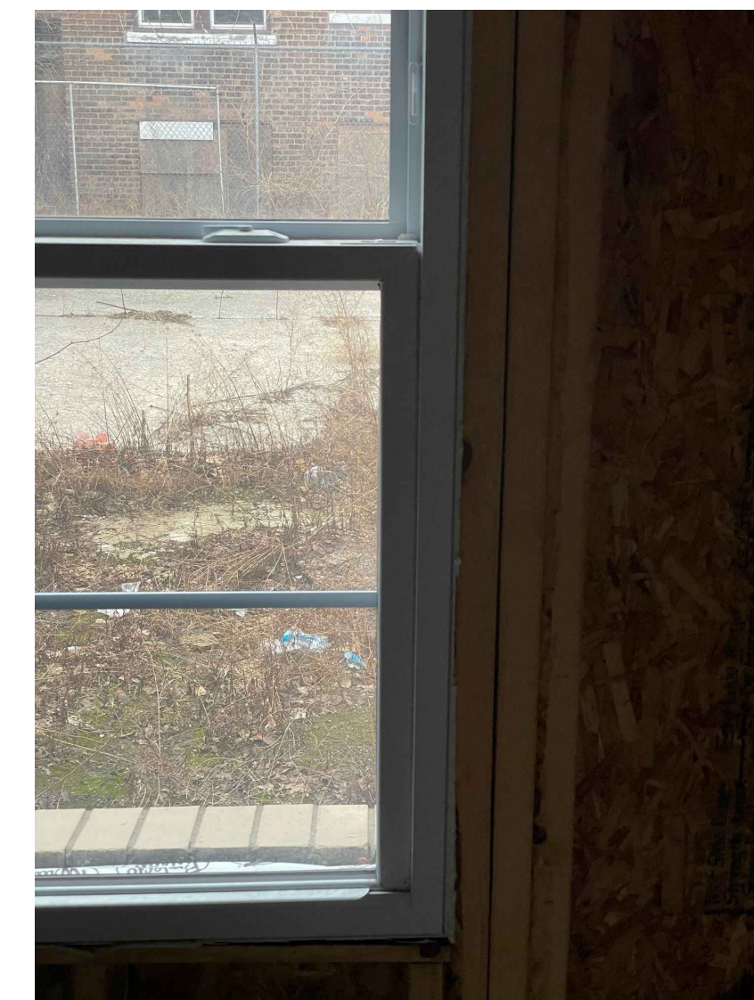
window interior view at rebuilt areas
