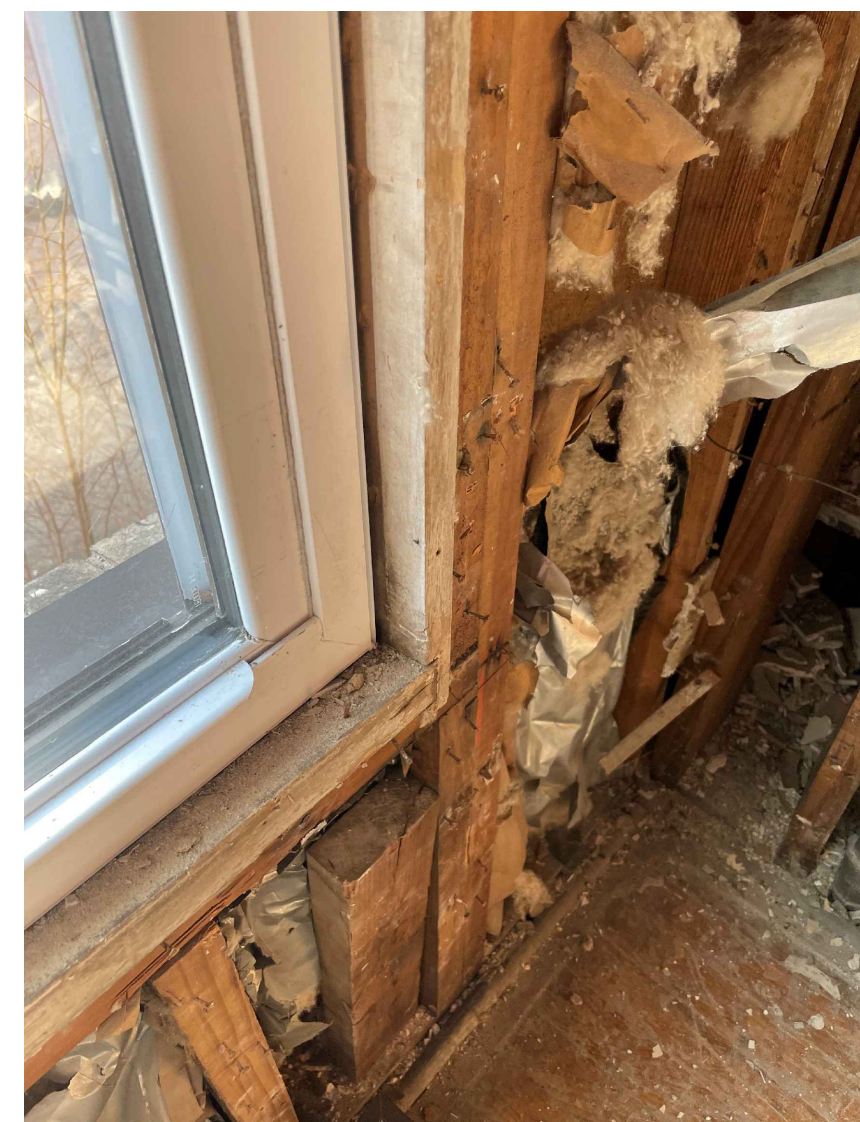
window interior view
