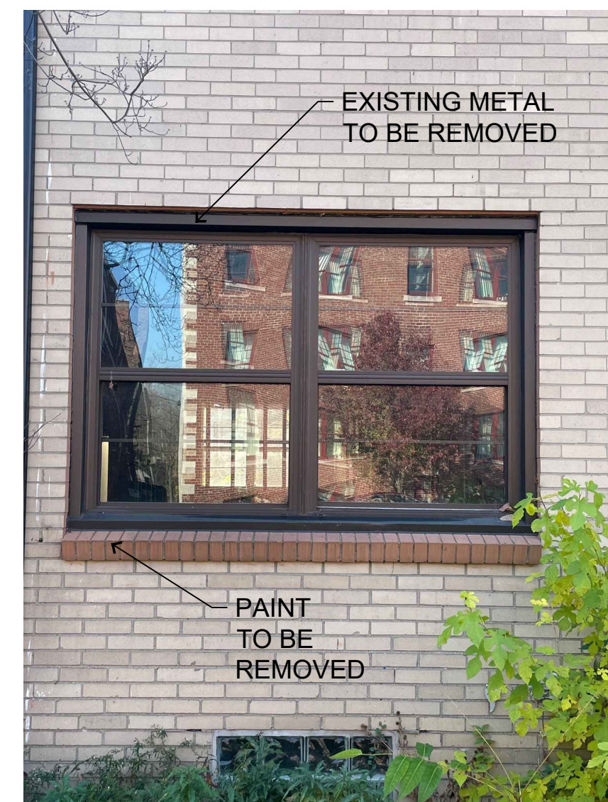
current window condition (typical for 160 windows)
