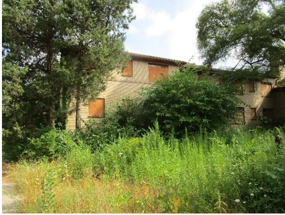
Photo 11: North elevation at west courtyard
