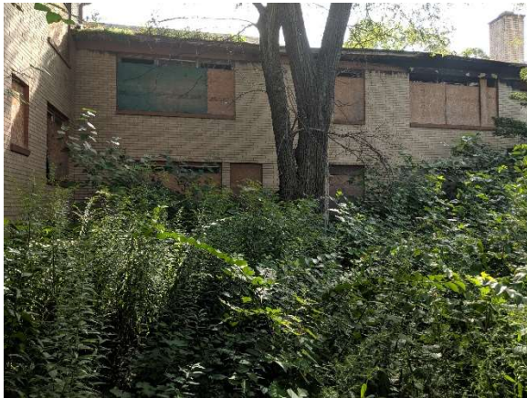
Photo 12: Partial east elevation at west courtyard
