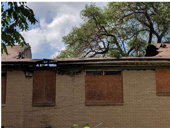
Photo 20: Roof at the center of the building.
