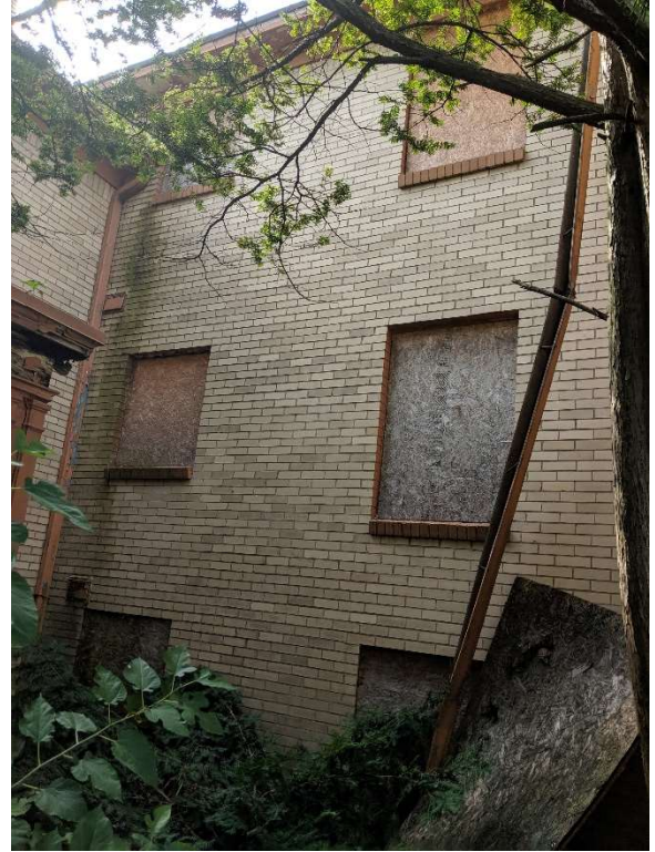
Photo 14: Partial south elevation at west courtyard
