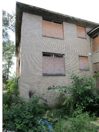
Photo 3: South elevation of east courtyard
