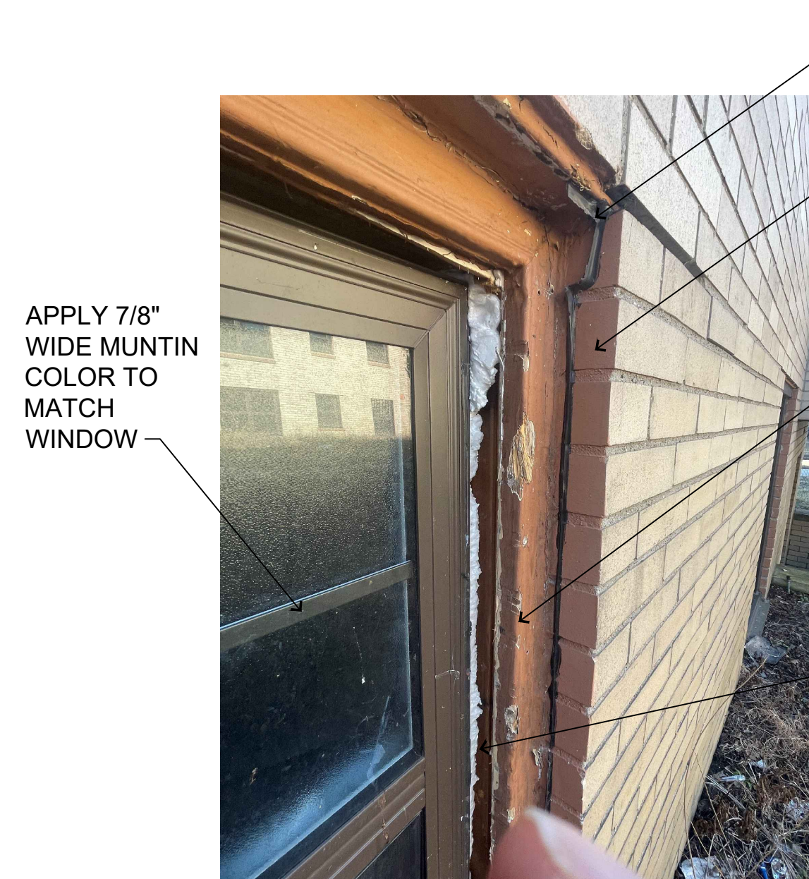
window with metal removed (top right view)
