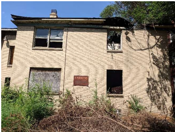
Photo 19: Roof at northeast wing of the building
