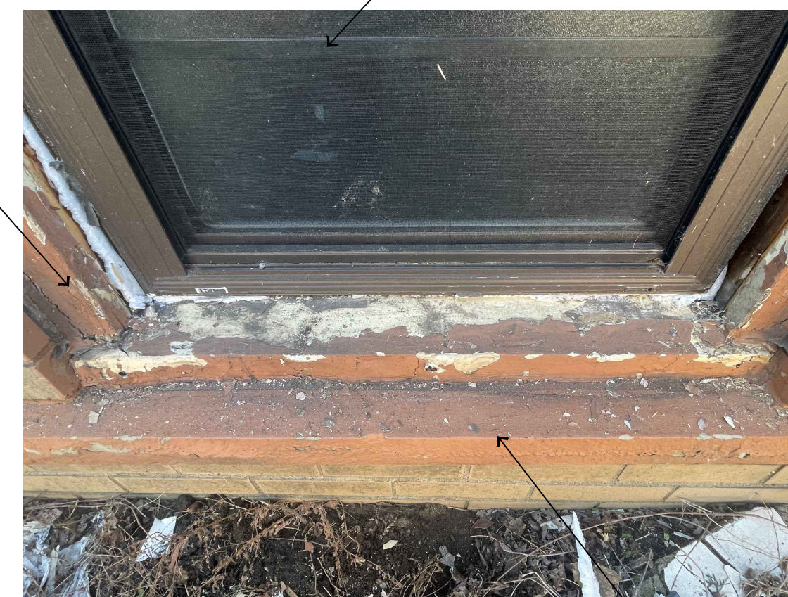
window with metal removed (bottom stool view)
