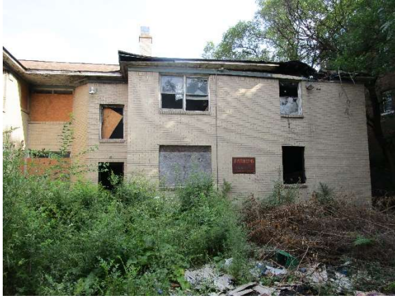
Photo 5: North elevation at east courtyard
