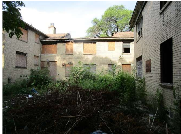
Photo 4: West elevation of East courtyard
