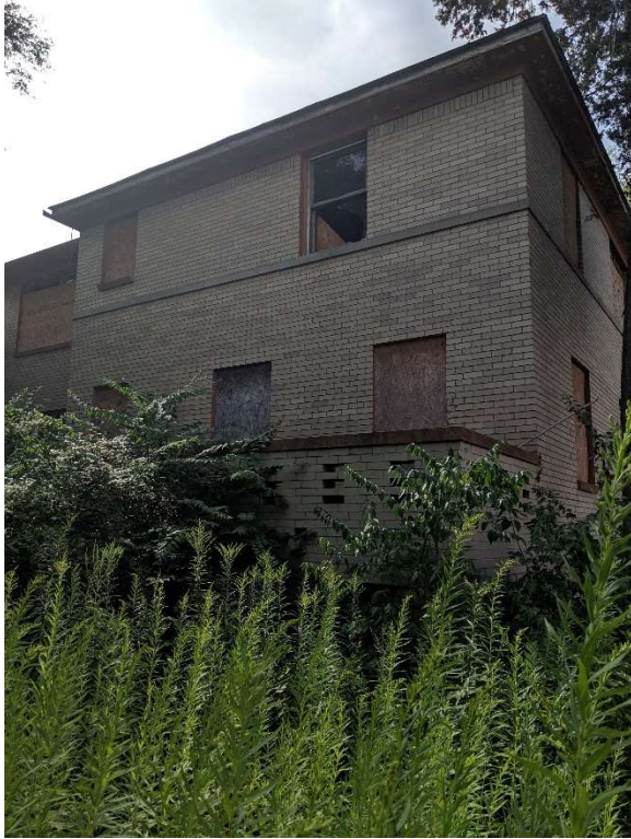
Photo 16: Partial south elevation at West courtyard
