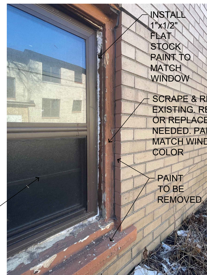
window with metal removed (bottom right view)
