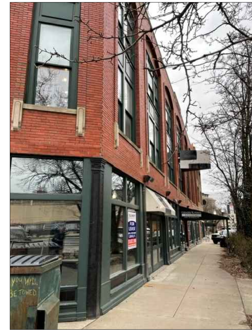
VIEW LOOKING NORTH
