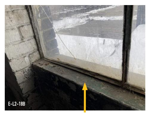
NOTE THAT STEEL SILL WAS ORIGINALLY SET ON MASONRY OPENING AND CONCRETE SILL WAS POURED TO ENCASE WINDOW.
