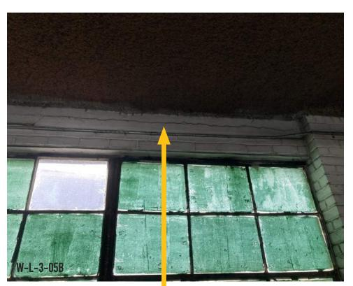
NOTE CRACKING IN STRUCTURAL PERIMETER BEAM WHICH MUST BE REPAIRED.
