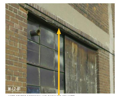
NOTE SEVERE CORRSION AND BUCKLING OF LINTEL.
