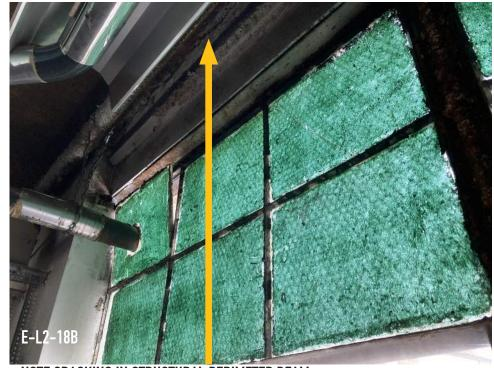
NOTE CRACKING IN STRUCTURAL PERIMETER BEAM WHICH MUST BE REPAIRED AS WELL AS CORROSION OF LINTEL.
