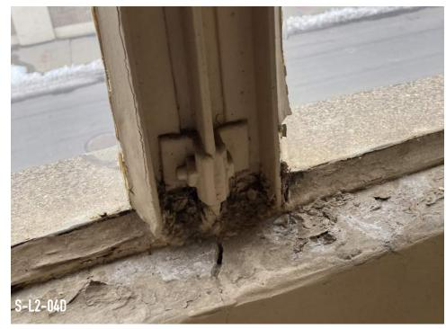
NOTE CORROSION AT EMBEDDED SILL IN CONCRETE
