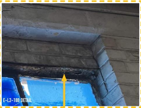
NOTE SEVERE CORROSION OF LINTEL – ALL LINTELS MUST BE REPLACED AND WINDOW FRAME IS INTEGRALLY ATTACHED TO LINTEL
