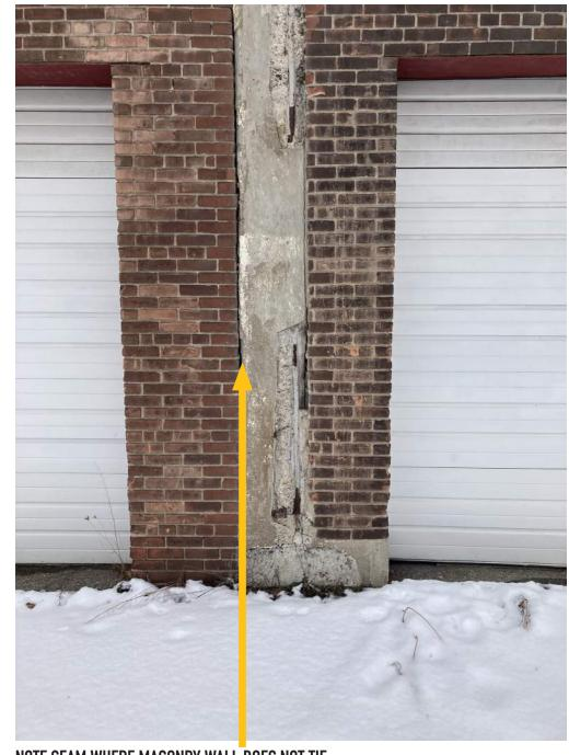
NOTE SEAM WHERE MASONRY WALL DOES NOT TIE INTO HISTORIC BUILDING
