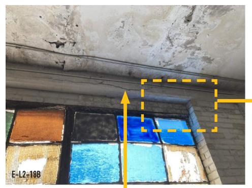
NOTE CRACKING IN STRUCTURAL PERIMETER BEAM WHICH MUST BE REPAIRED.
