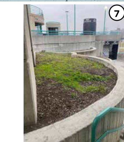
7 Remove grass from bed, plant new juniper shrubs and add mulch.
