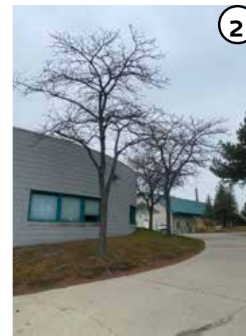
2 Fill landscape area with topsoil and reseed. Prune honeylocust branches away from building
