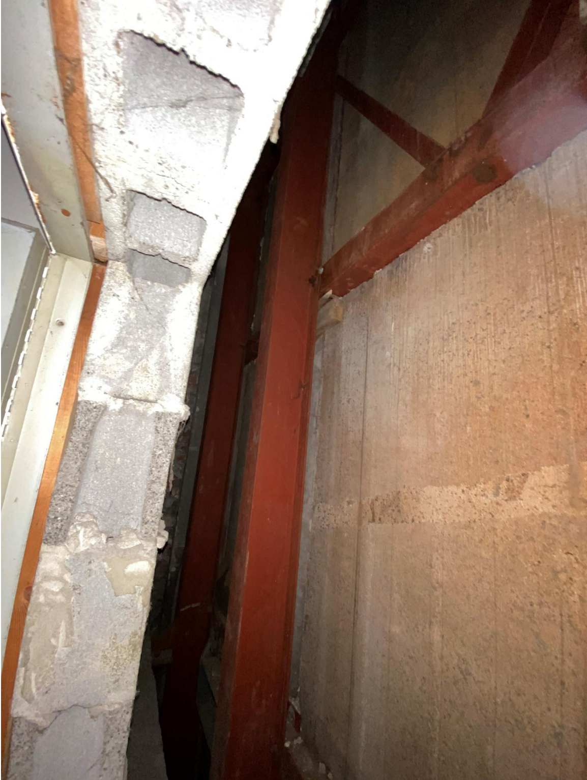
Figure #23: Interior, Looking into hatch at CMU structure with no limestone visible. 3/9/22
