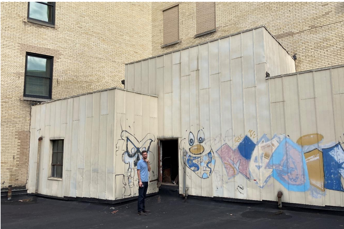
Figure #12: Exterior, Roof. 8/4/22
