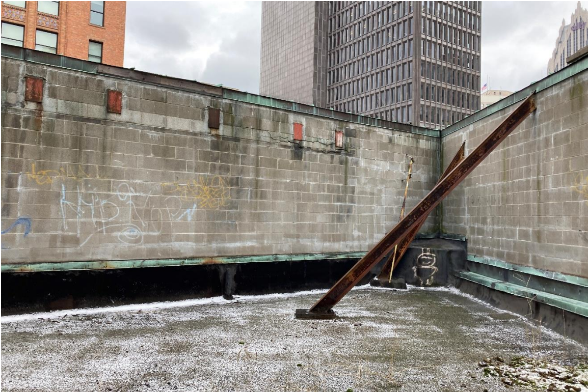
Figure #13: Exterior, Roof. 12/7/21
