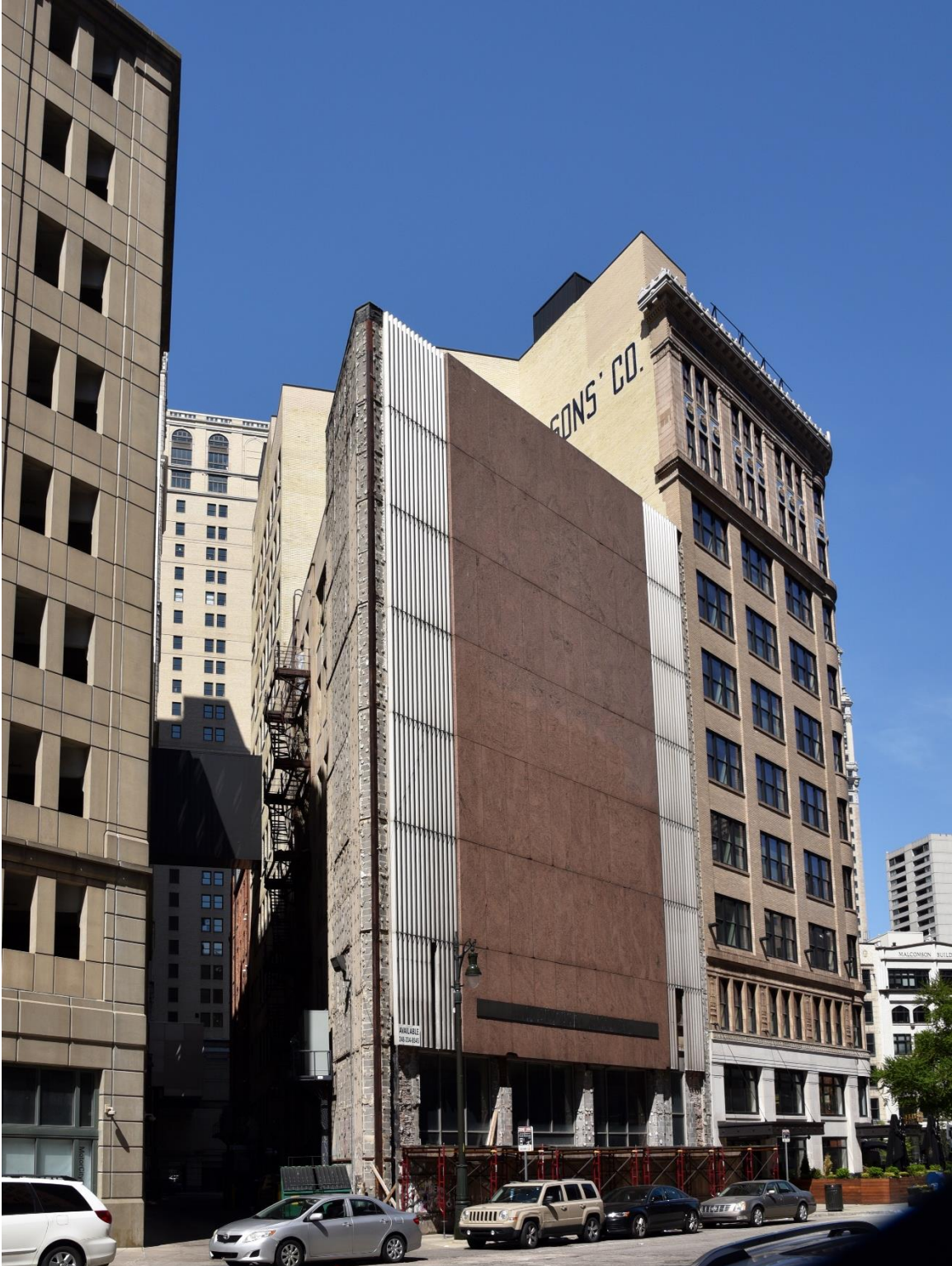
Figure #1: Exterior, Primary Façade. 5/15/22
