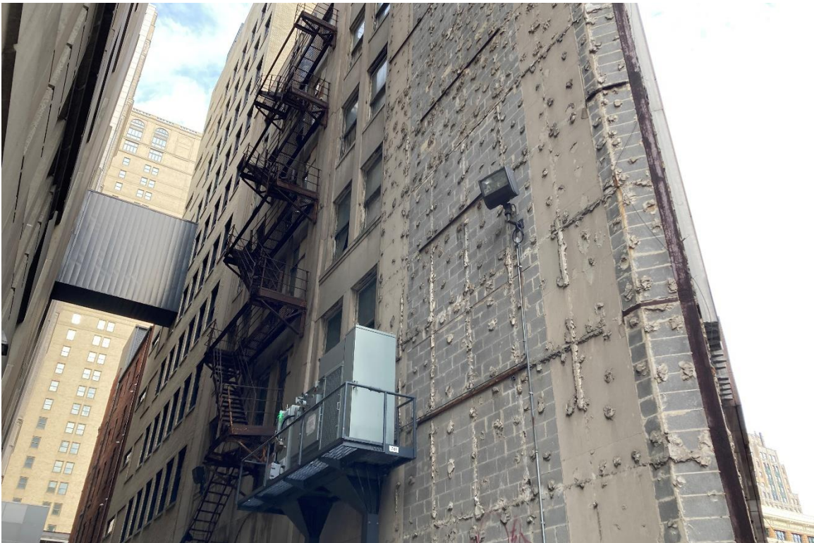
Figure #6: Exterior, Alley Façade. 8/4/22
