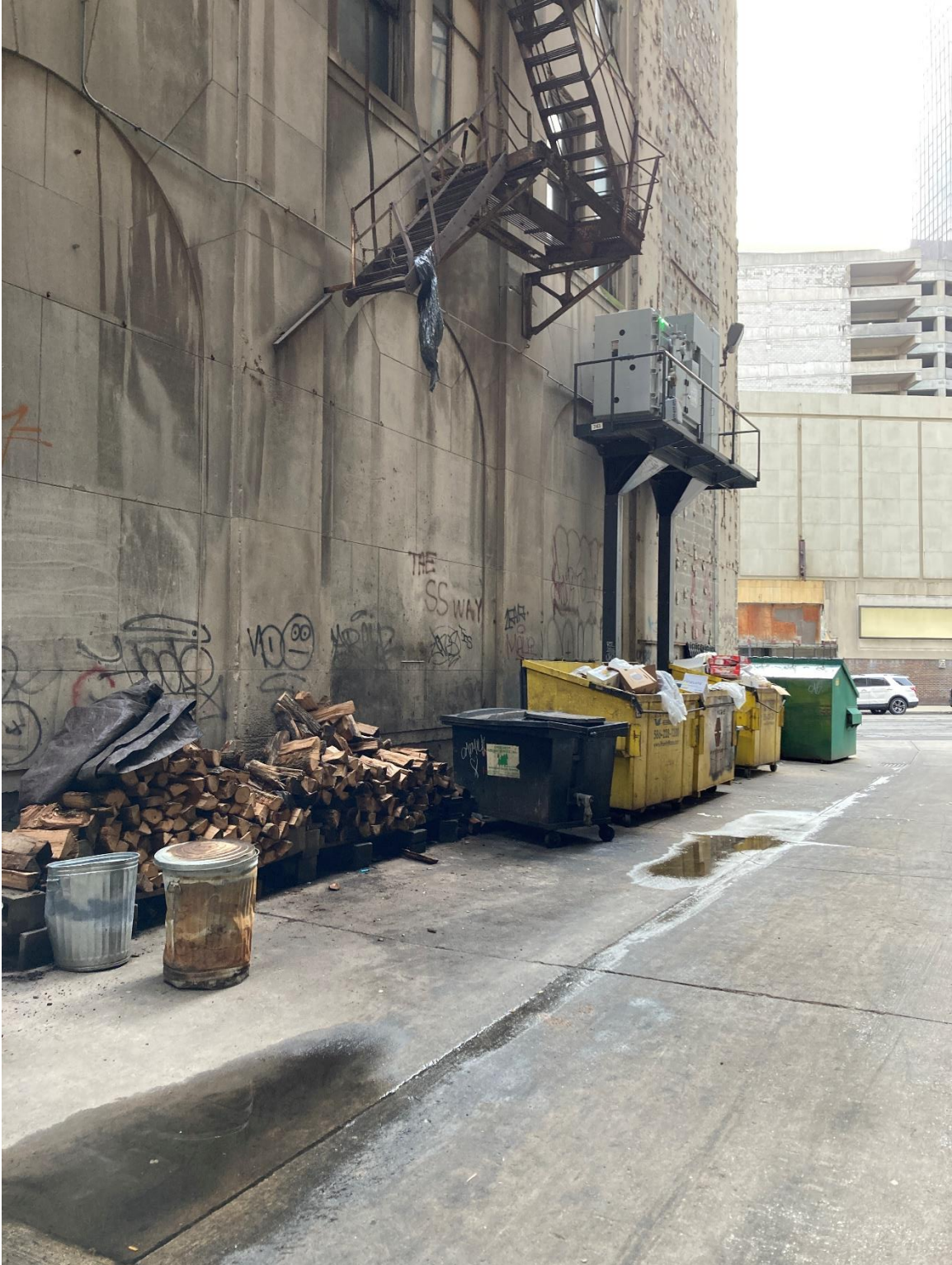
Figure #9: Exterior, Alley Façade. 8/4/22
