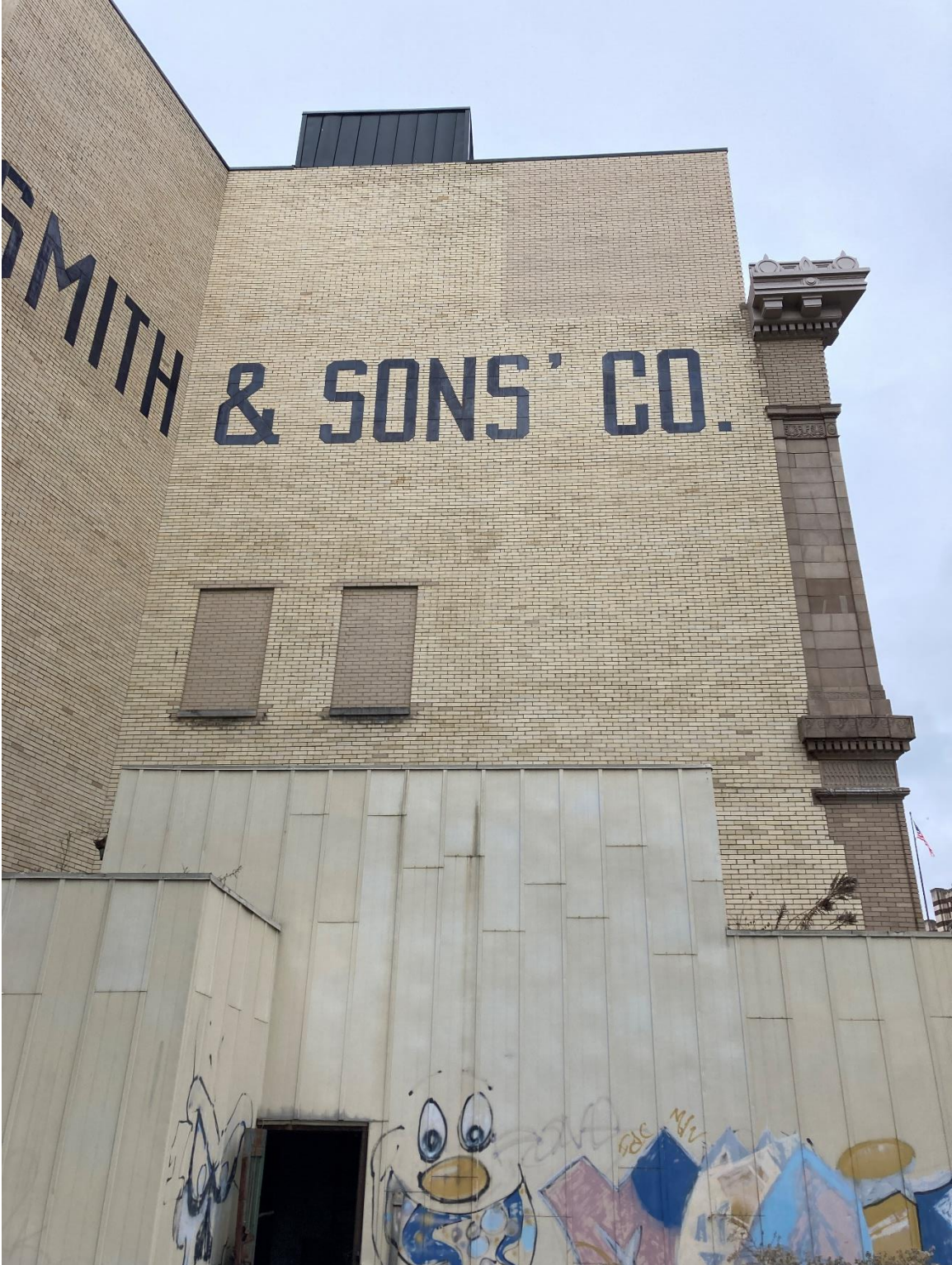
Figure #16: Exterior, Looking at the South Façade of 1145 Griswold. 12/7/21
