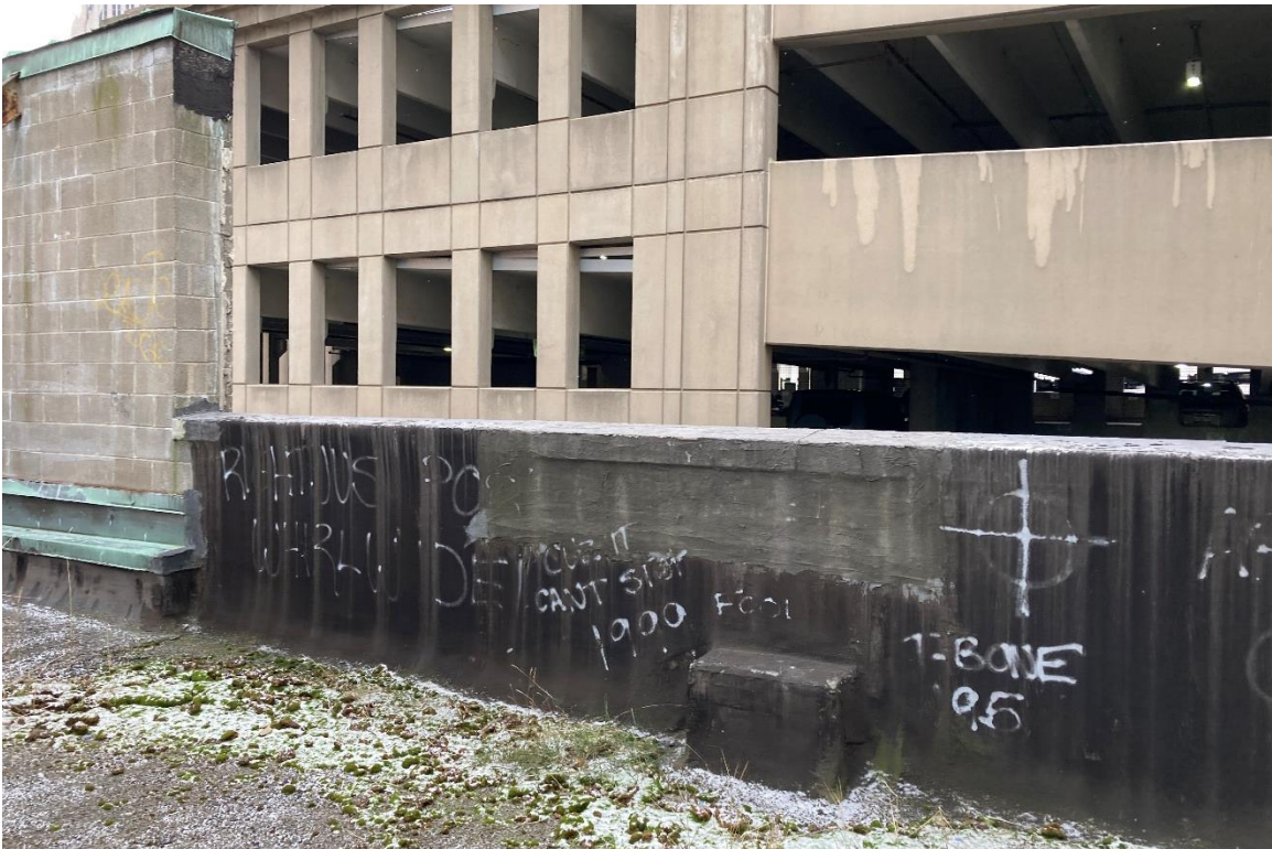
Figure #14: Exterior, Roof. 12/7/21
