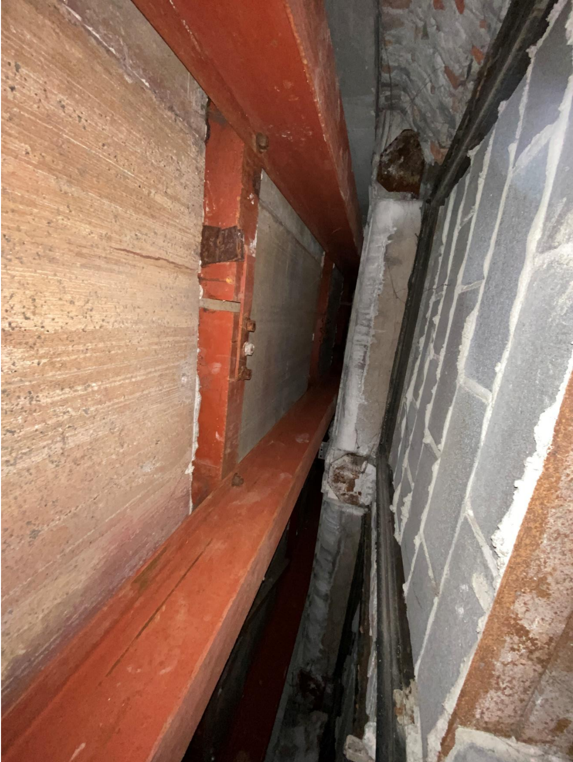
Figure #24: Interior, Looking into hatch with no limestone visible. 3/9/22
