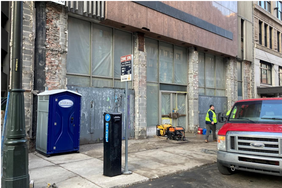
Figure #4: Exterior, Primary Façade. 2/8/23
