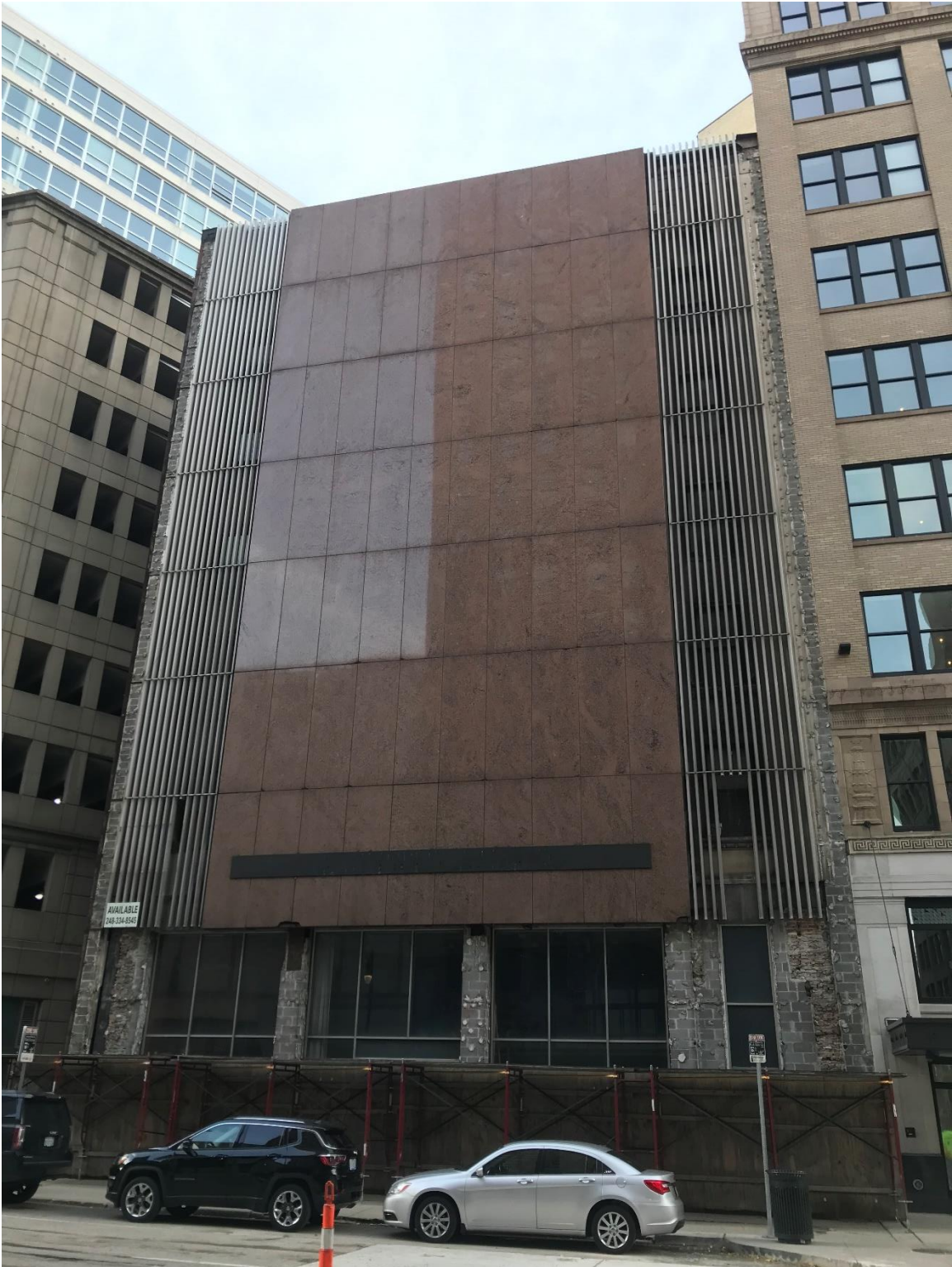
Figure #10: Exterior, Primary Façade. 11/18/21
