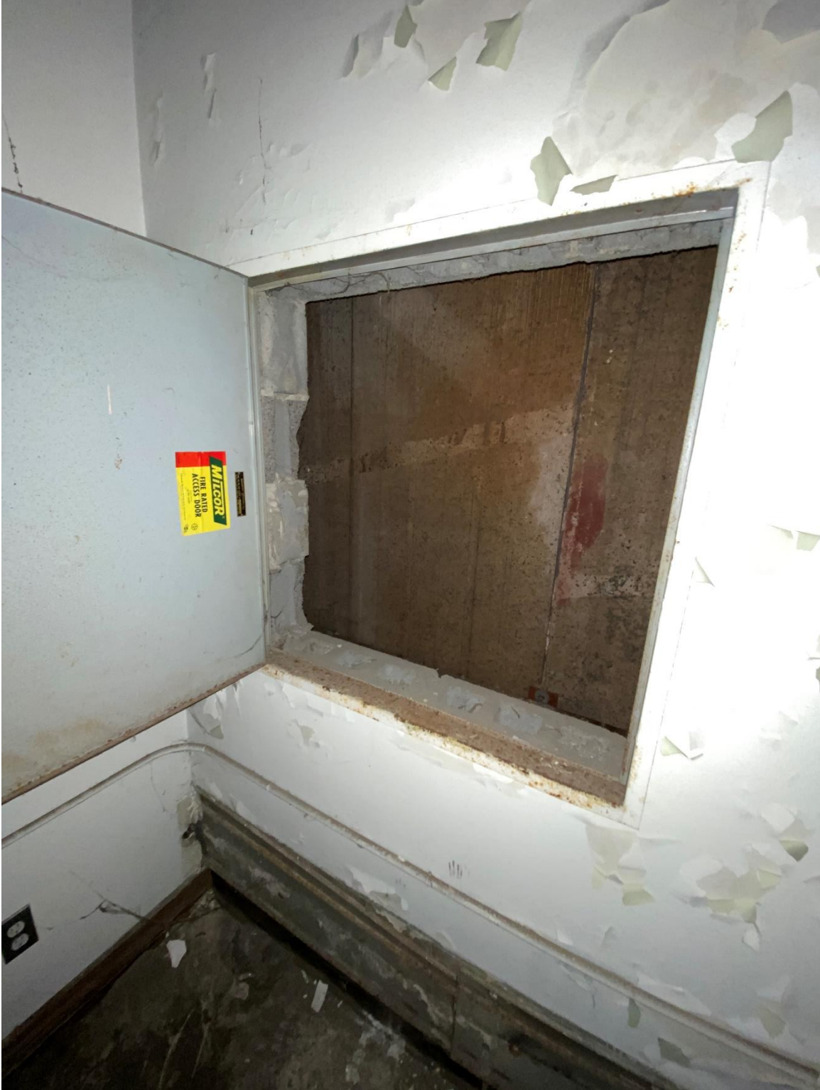
Figure #22: Interior, Hatch to view portion of façade. 3/9/22
