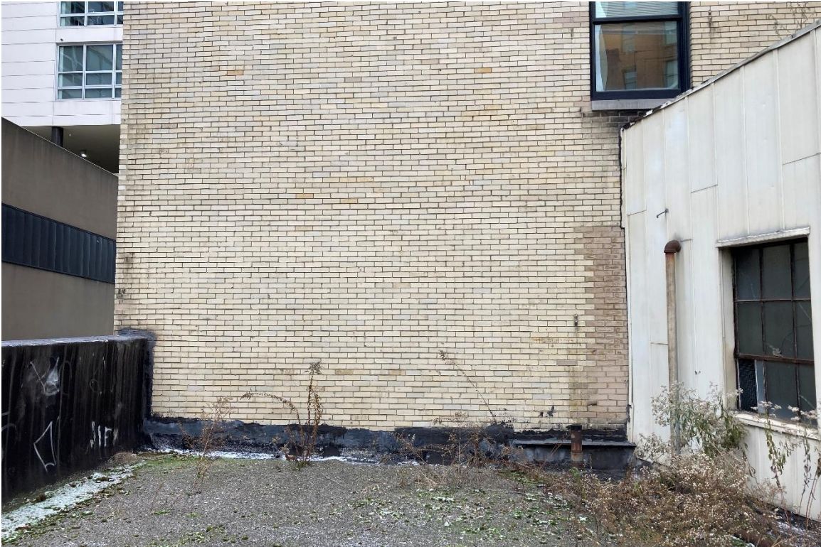
Figure #11: Exterior, Roof. 11/18/21
