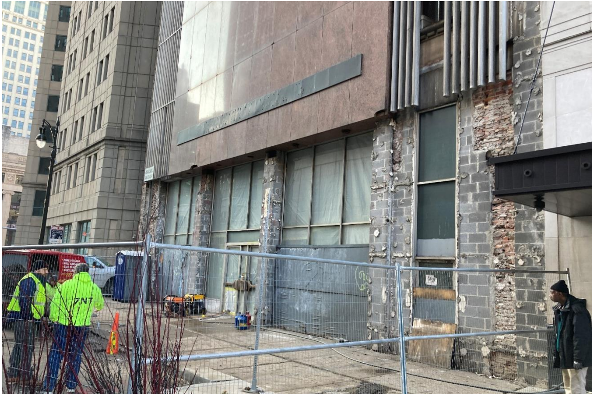
Figure #3: Exterior, Primary Façade. 2/8/23
