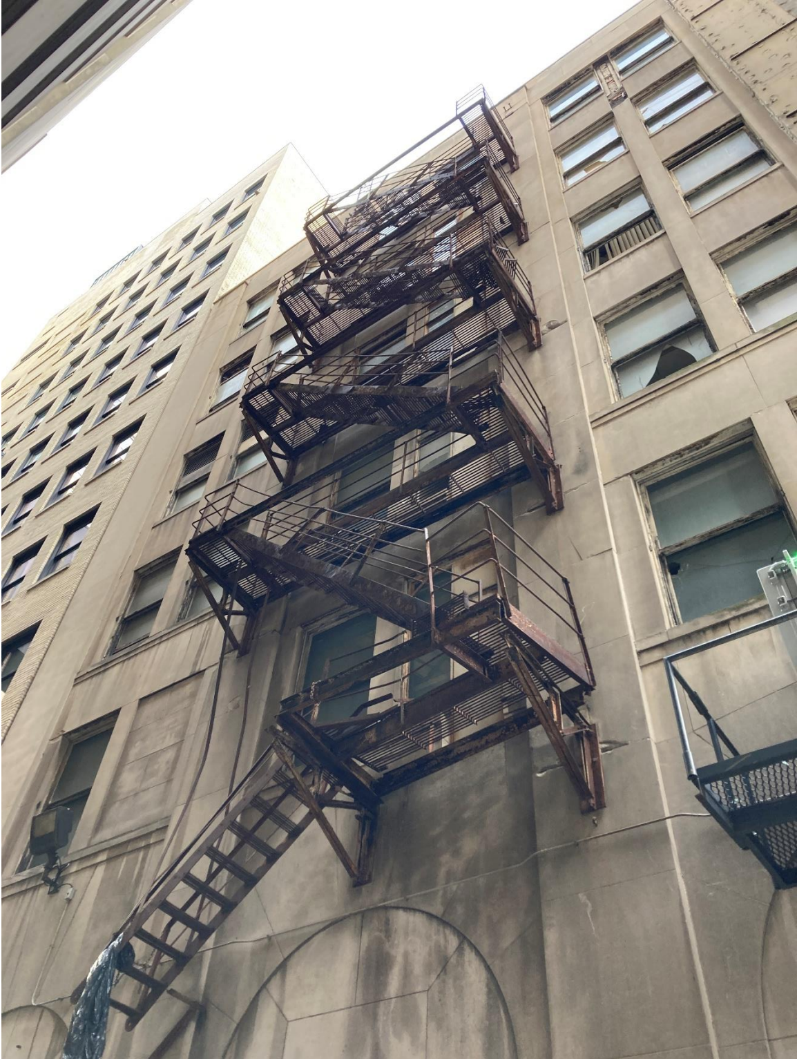
Figure #8: Exterior, Alley Façade. 8/4/22
