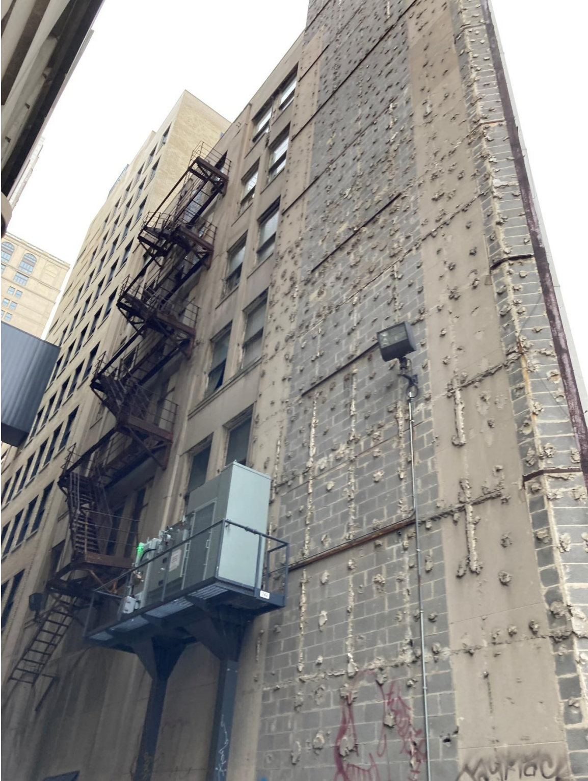
Figure #7: Exterior, Alley Façade. 12/7/21
