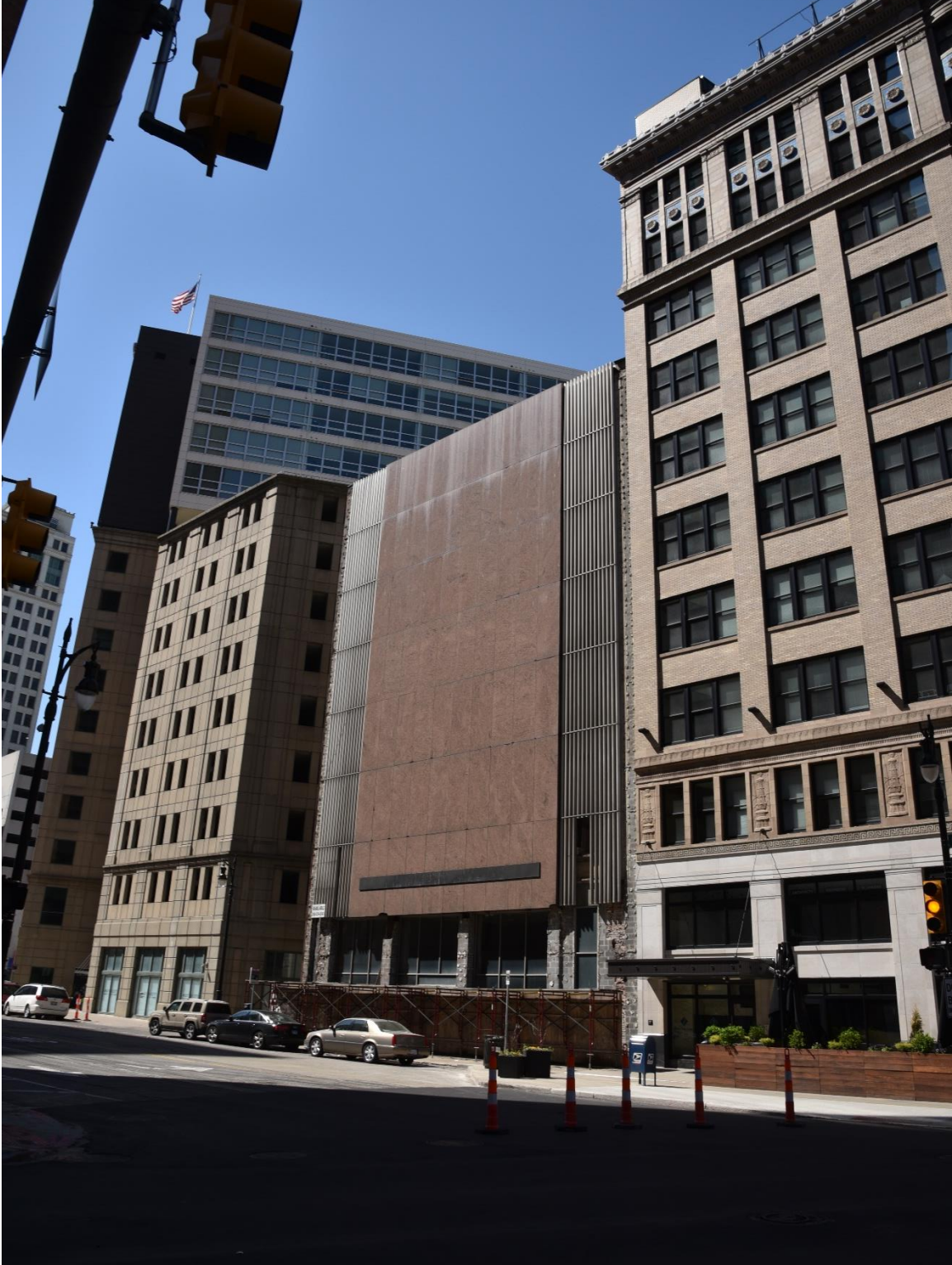
Figure #2: Exterior, Primary Façade. 5/15/22
