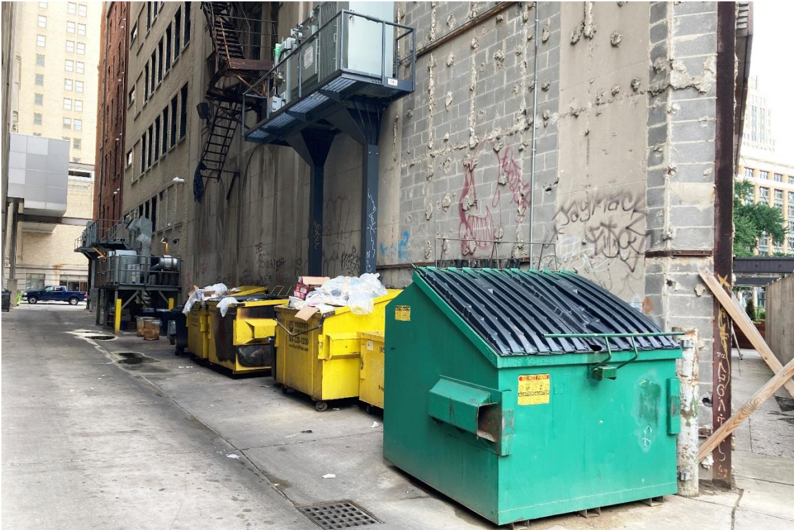
Figure #5: Exterior, Alley Façade. 8/4/22
