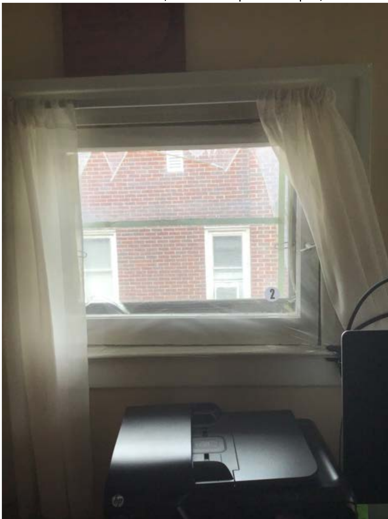
Window #2- Latch won't close; no available parts for repair; no storm window
