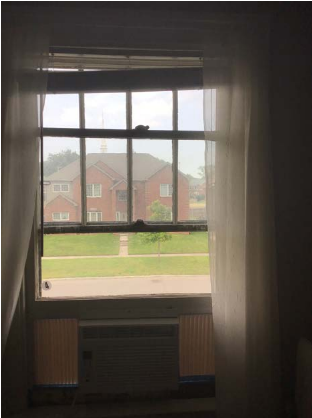
WINDOW #4 - No storm window, won't stay open on its own.
