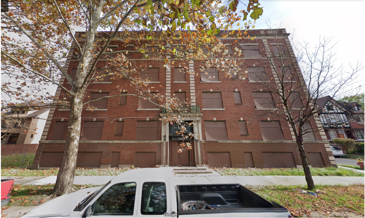
Front (West) Elevation - Vinewood Avenue
