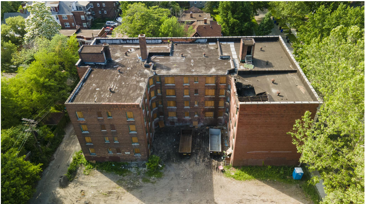
North Elevation - Side Yard from above
