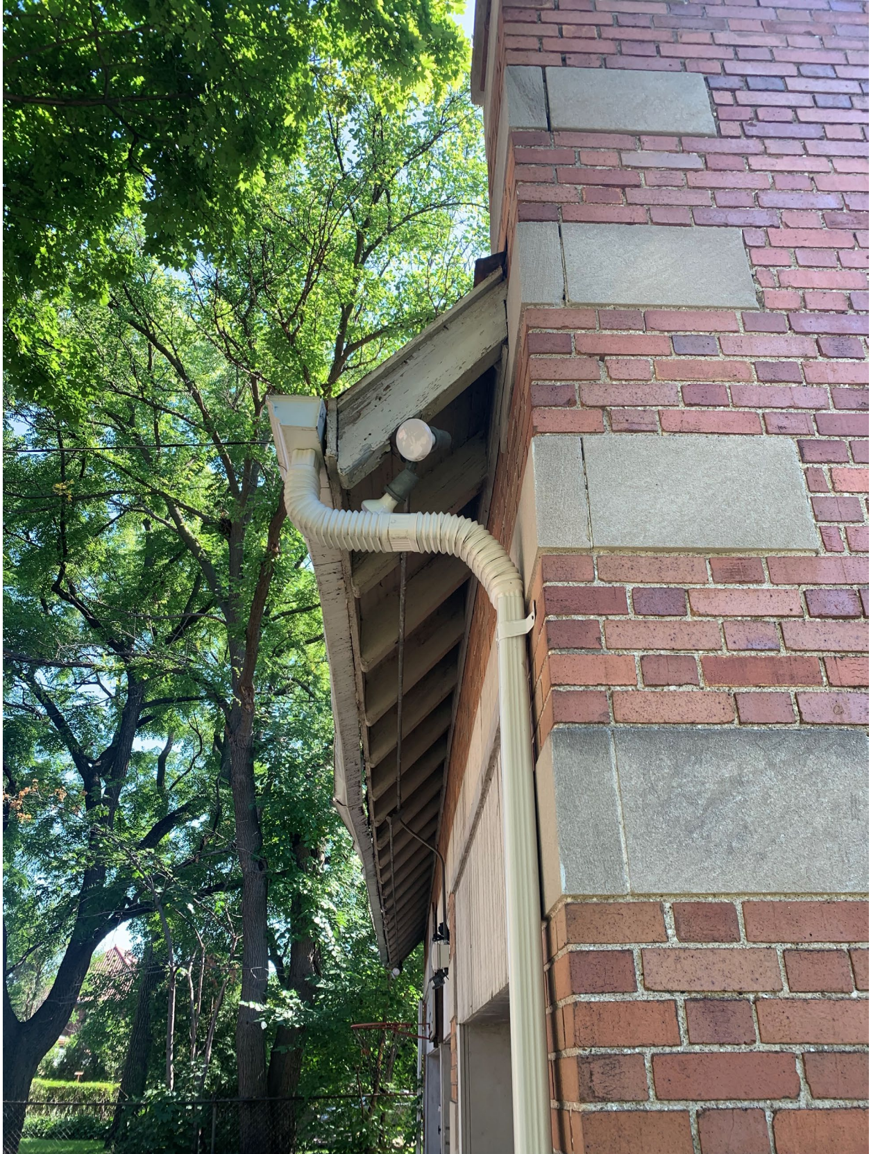
Garage: Brick Coursing And Limestone Masonry Quoins, Rafter Tails.
