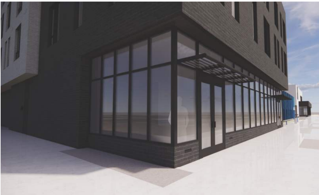
Prefabricated Sunshade reduced to cover South facing entrances. MANUFACTURER: Tubelite Inc (Same manufacturer as the storefront assemblies to ensure compatibility and color matching) Maxblock Airfoil, 35" Outrigger with 6 blades
