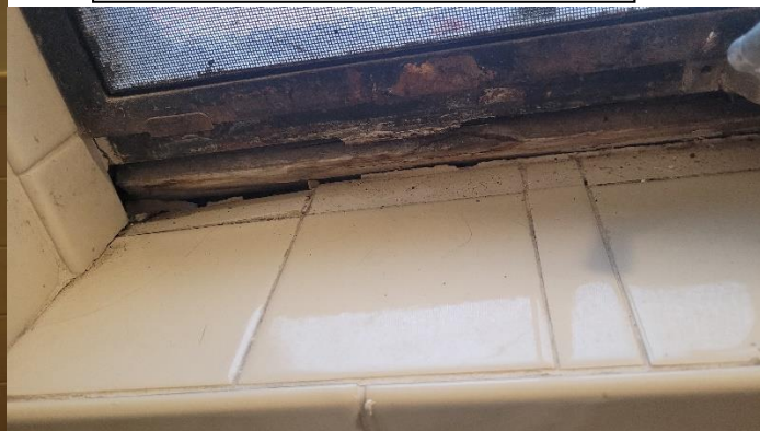
Rotting of trim around second story bathroom window
