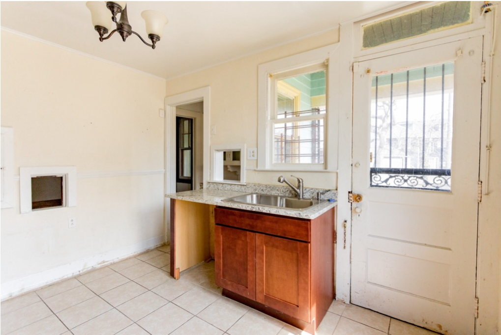
THE CURRENT KITCHEN IS A COMBINATION OF THE ORIGINAL CONFIGURATION AND A BAD RENOVATION SOME TIME LATER. BOTH ARE INADEQUATE FOR MODERN USE. TO HELP MAKE THE KITCHEN MORE FUNCTIONAL WE'D LIKE TO PROPOSE USING THE FRENCH DOORS IN THE LIVING ROOM AS THE MAIN ACCESS POINT TO THE REAR AND CLOSING OFF THIS DOOR IN THE KITCHEN, ADDING A SASH DOUBLE HUNG WINDOW IN ITS STEAD.
